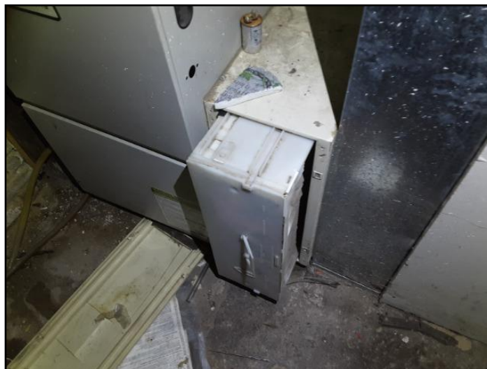
Furnace air filter location
