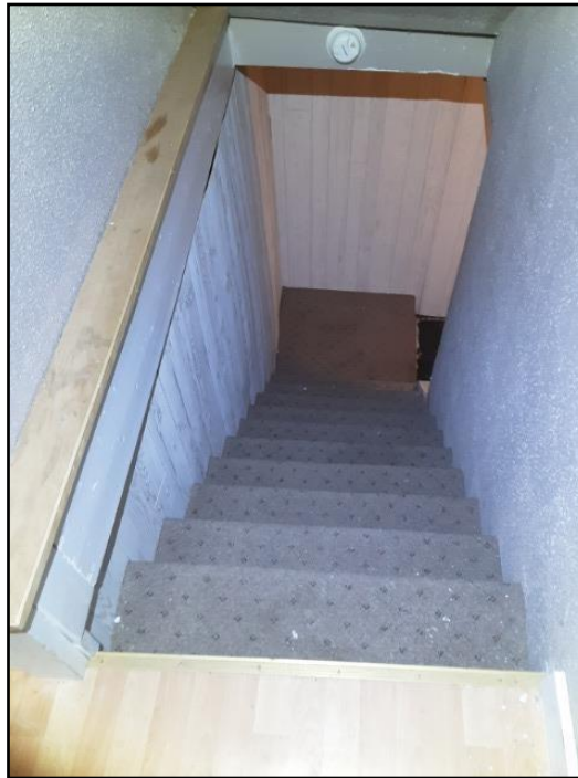
Handrail missing
