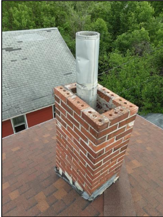
Missing chimney cap
