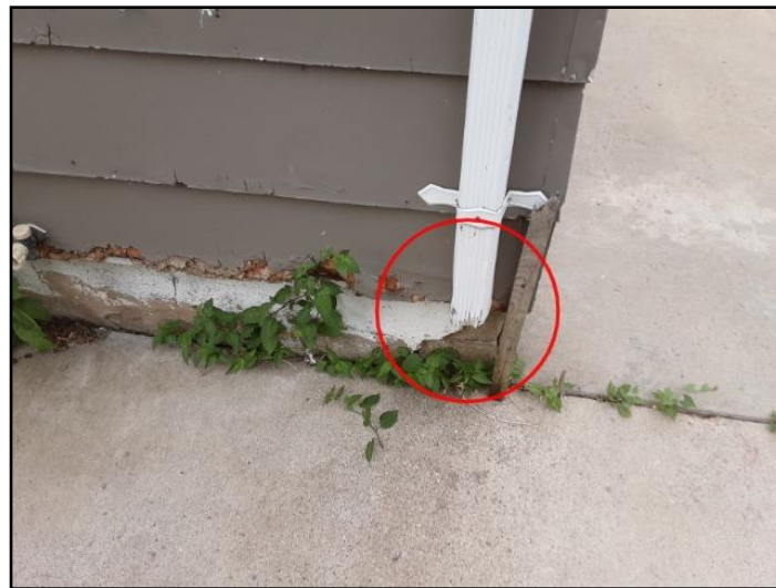
Downspout extension(s) missing
