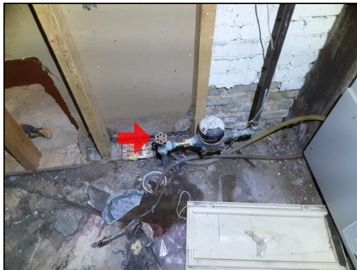
Water meter - Main water shutoff
