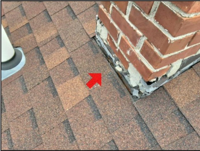
Flashing not set into shingles properly
