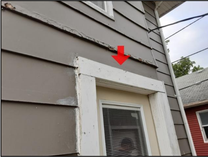
Drip cap(s) missing
