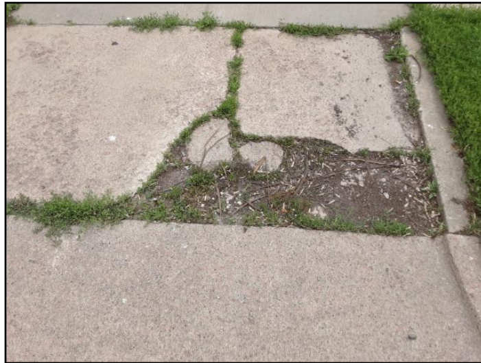
Cracked and damaged concrete
