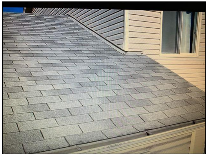
4. Asphalt shingles
