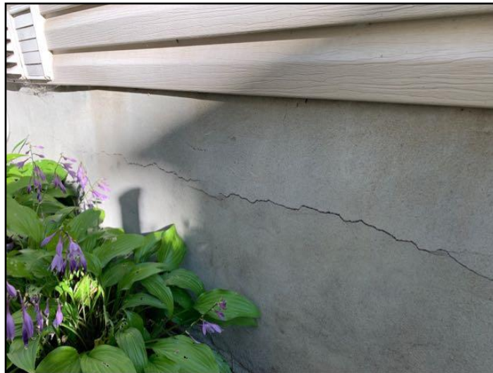
12. Cracked horizontally
