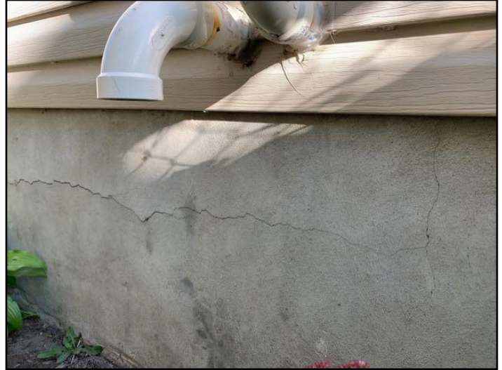
11. Cracked horizontally
