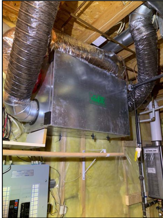
22. Heat recovery ventilator (HRV)
