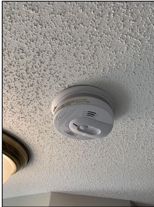
17. Combined Unit - Smoke and Carbon monoxide...
