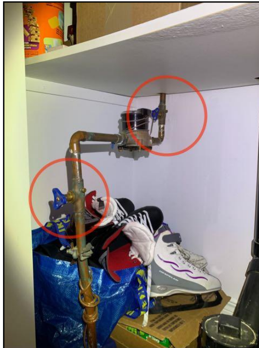
35. Main water shut off Valve
