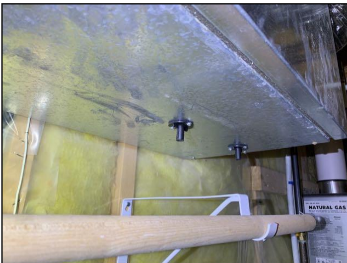
25. Missing the condensate line
