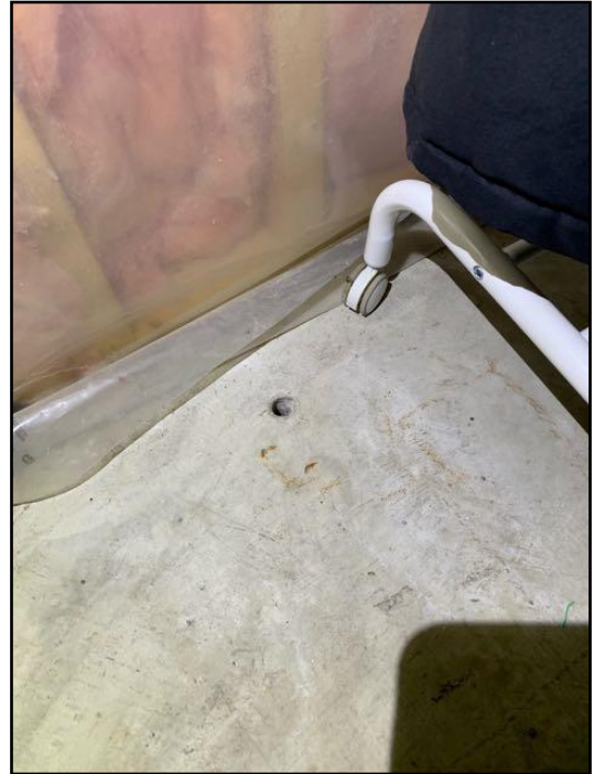
26. Drain hole for condensate line from HRV
