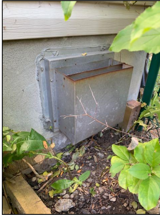
21. Sidewall venting
