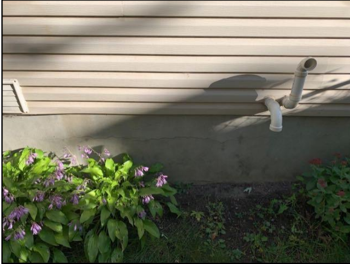
10. Cracked horizontally
