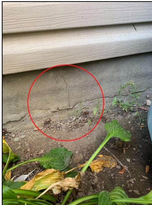
9. Typical minor cracks
