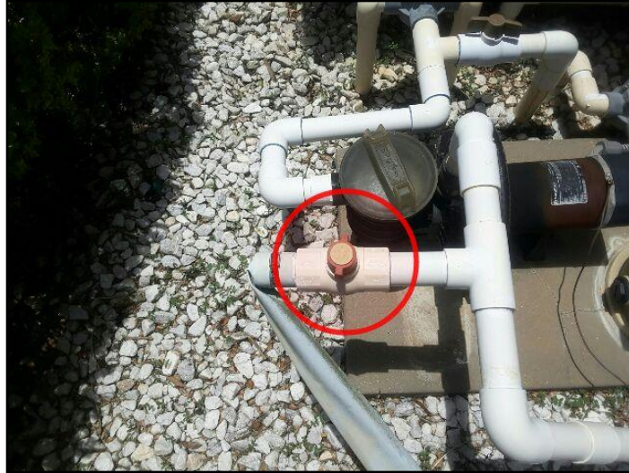
68. Valves broken or inoperable
