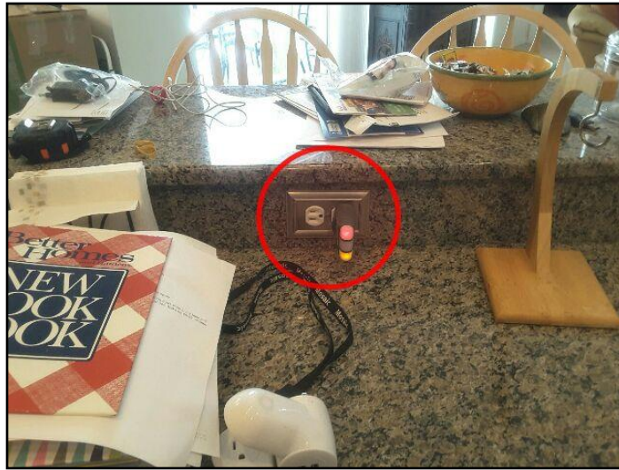
9. Reversed polarity
