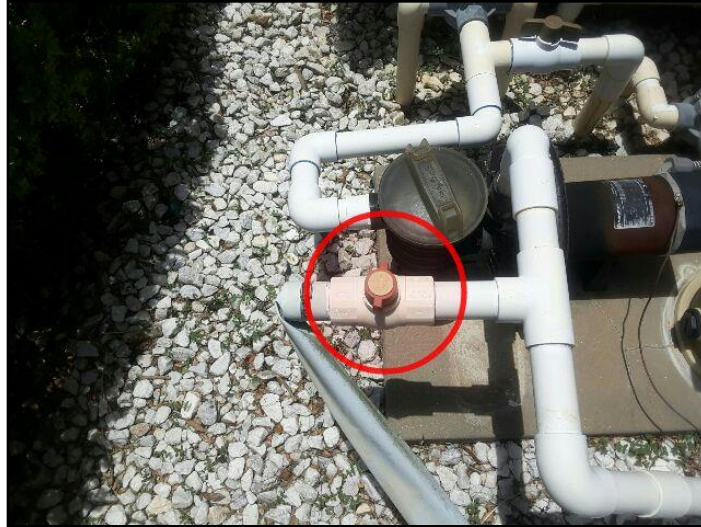
18. Valves broken or inoperable
