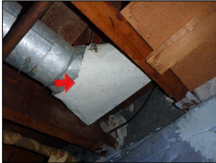
Likely an asbestos-containing material
