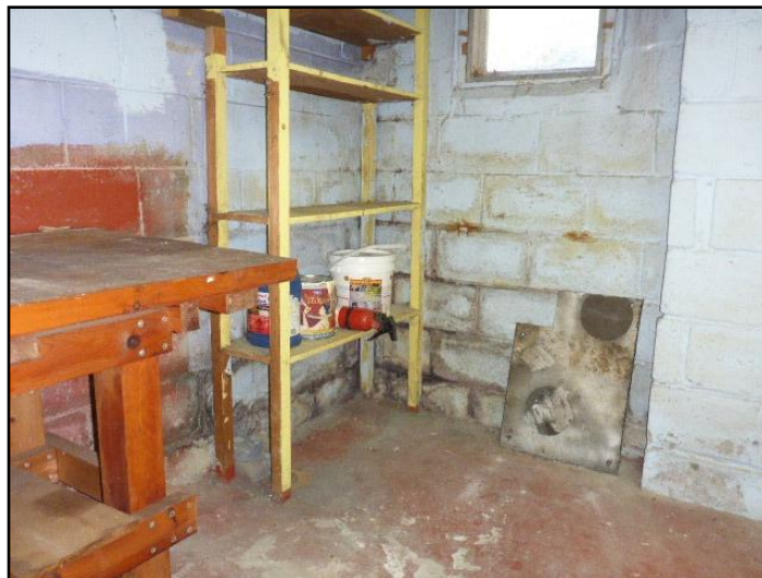
Mould/water stains in basement
