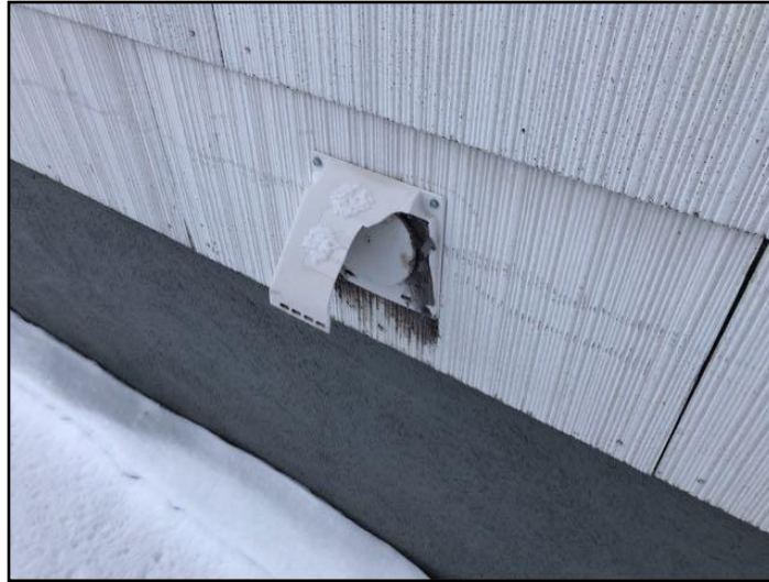
Cover damaged
