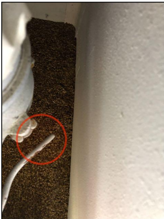
No jumper for meters and valves
