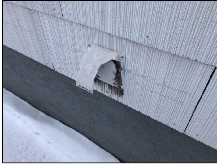
Cover damaged
