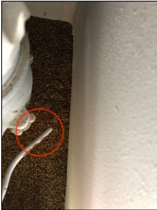
No jumper for meters and valves
