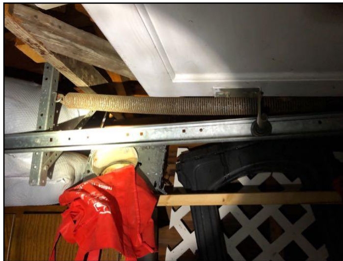
Missing safety cables
