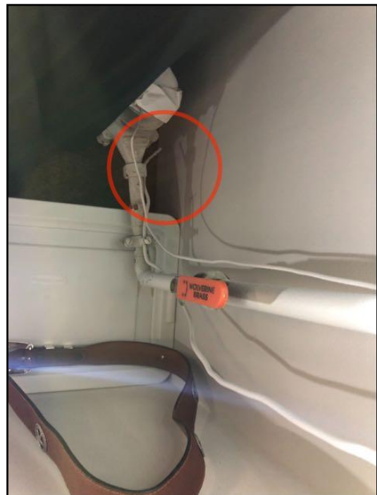
No jumper for meters and valves
