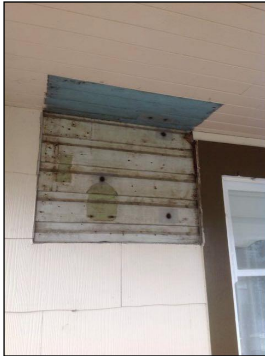
50. Siding - incomplete / missing
