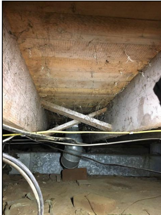
148. No Crawlspace Insulation
