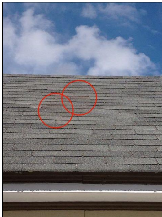
32. Missing Shingles
