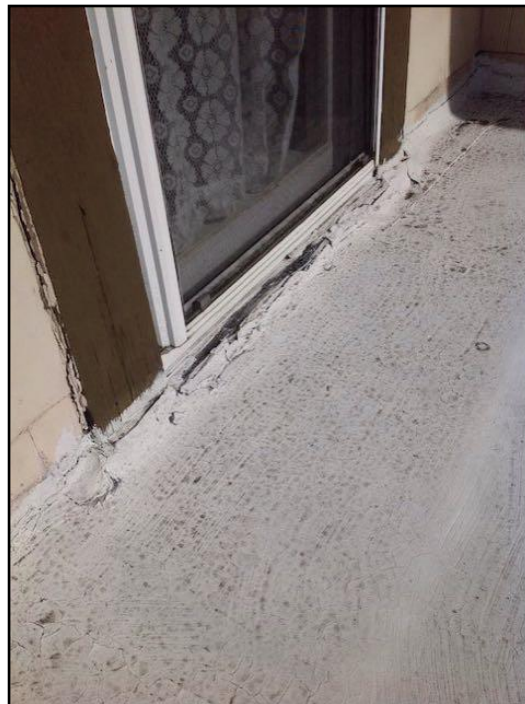
38. Questionable Flashing
