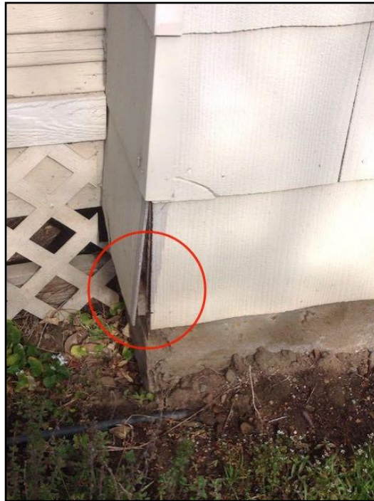
55. Flashings missing
