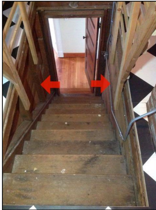
28. Missing Handrail
