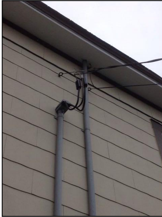
114. Service cables are securely attached.
