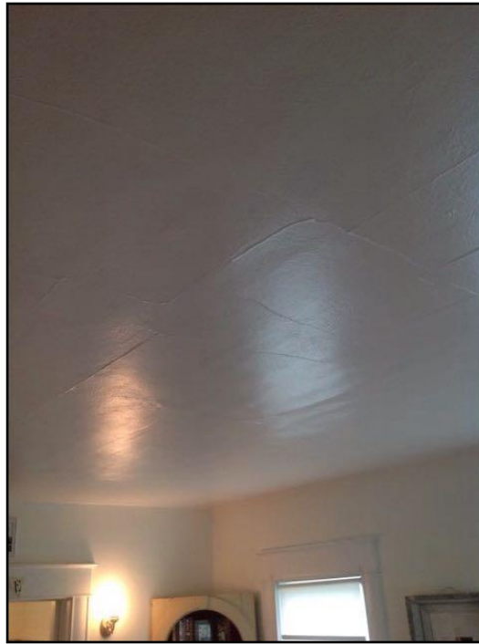
163. Ceiling Cracks
