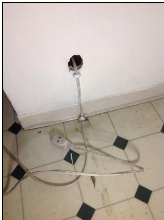
93. Extension cord used as permanent wiring
