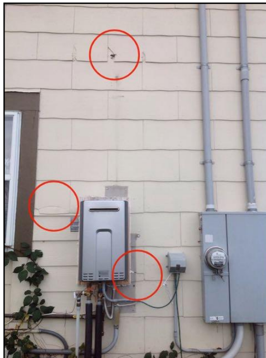
11. Siding - incomplete / missing
