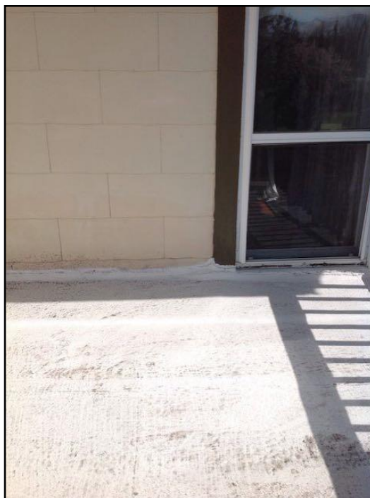
39. Questionable Flashing
