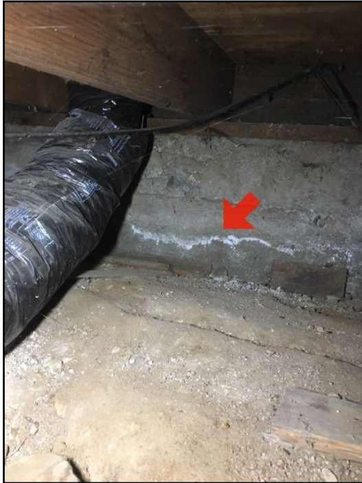
144. Efflorescence
