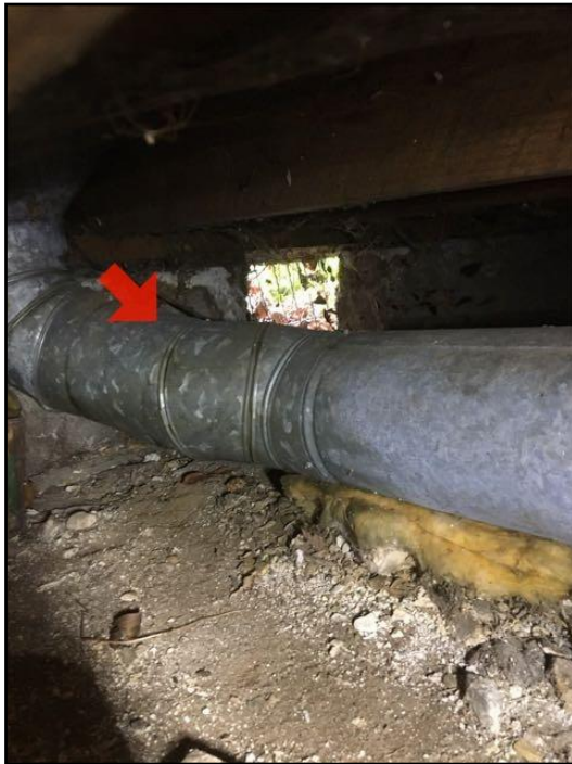
128. Insulation missing, damaged
