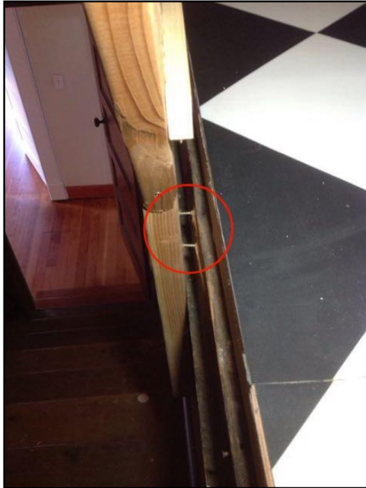
166. Loose handrail
