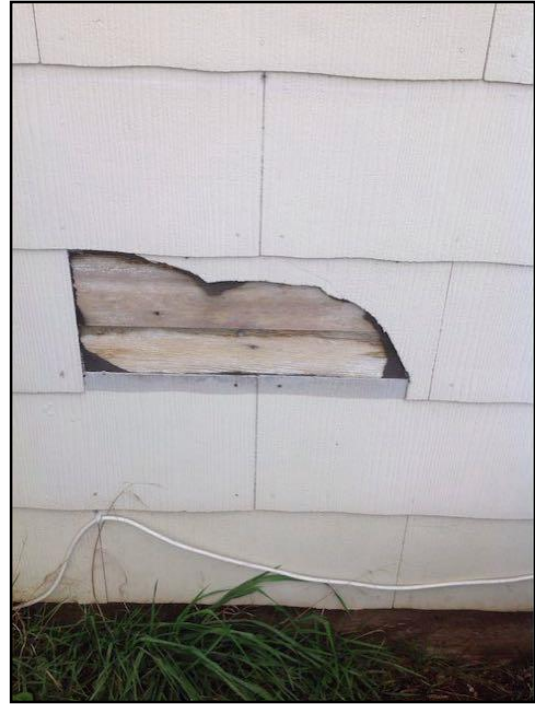
10. Siding - incomplete / missing
