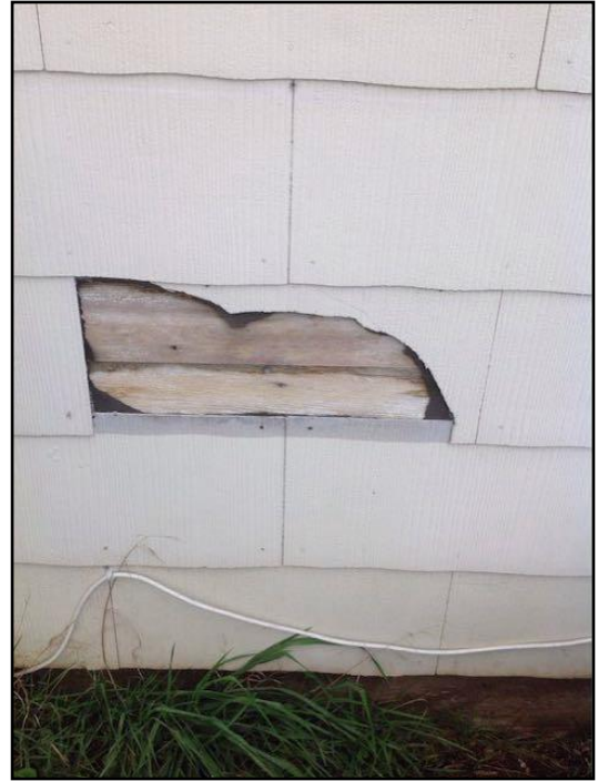
52. Siding - incomplete / missing
