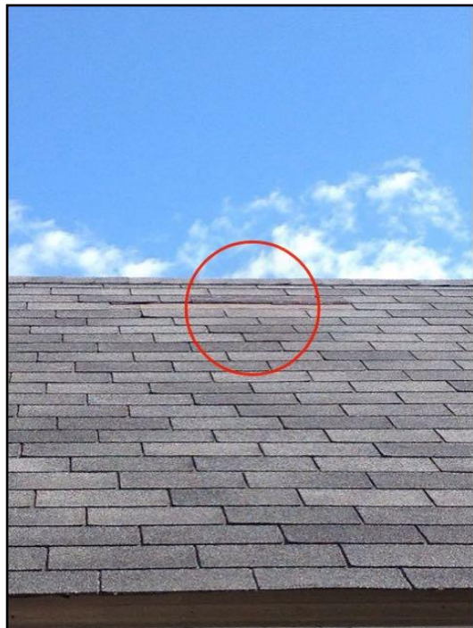
1. Missing Shingles
