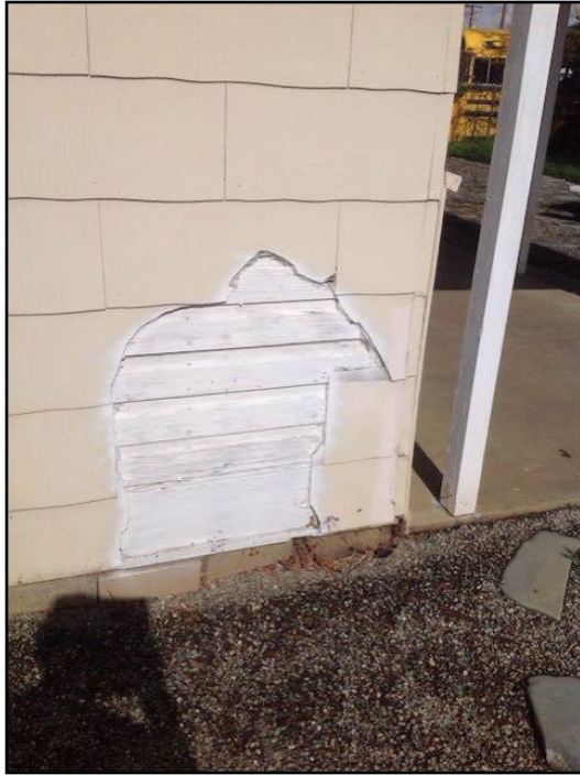
51. Siding - incomplete / missing
