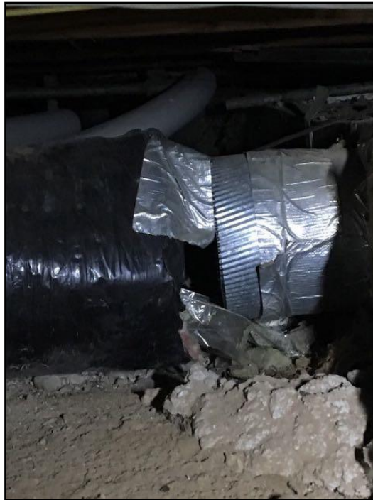
27. Disconnected duct
