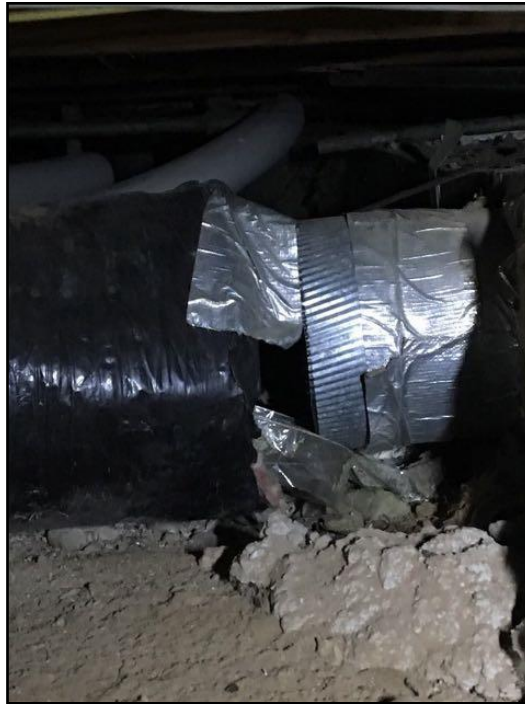
127. Disconnected duct
