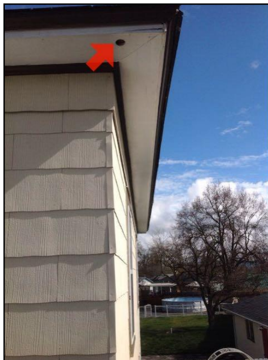
60. No Gutters Installed
