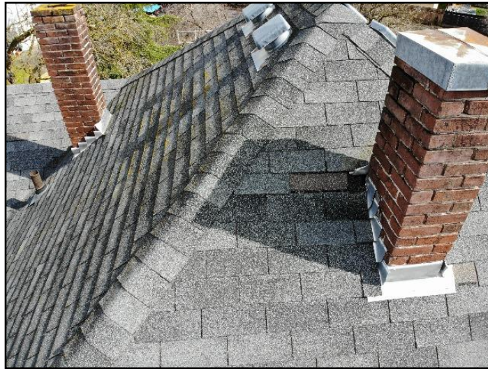
132. Loose, missing or deteriorated masonry
