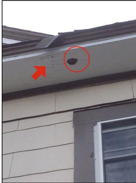
54. Moisture damage
