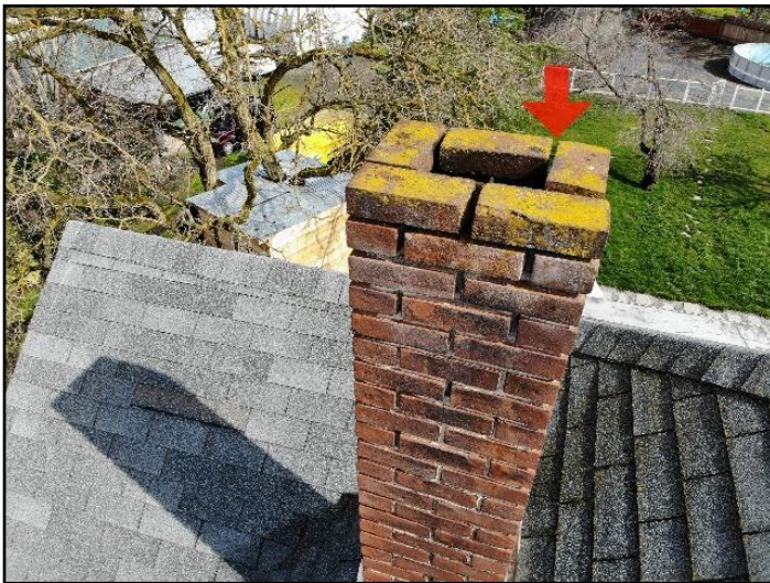
130. Loose, missing or deteriorated masonry
