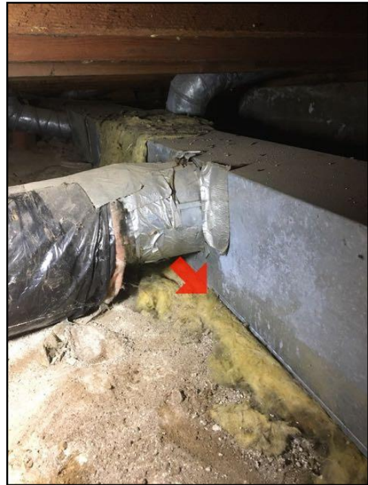
129. Disconnected ducts
