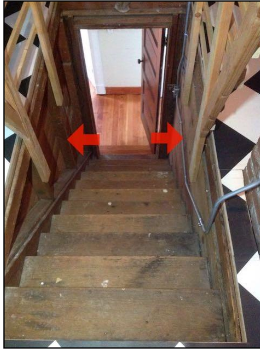
168. Missing Handrail
