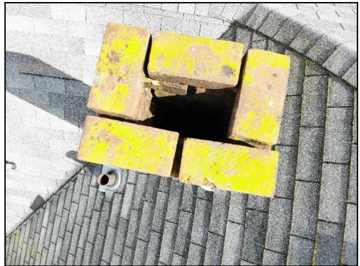
131. Loose, missing or deteriorated masonry
