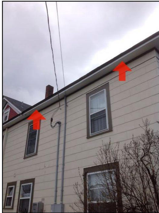
47. Missing Gutters
