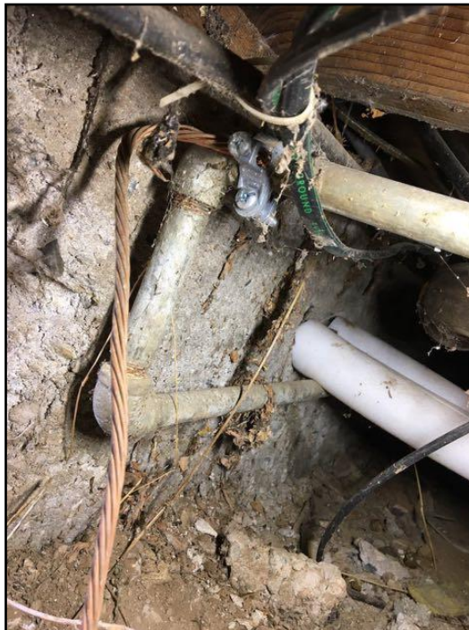
116. Copper - water pipe ground
