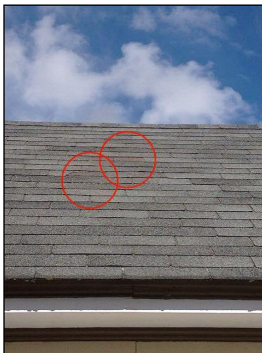
3. Missing Shingles
