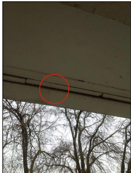
43. Leak behind gutter
