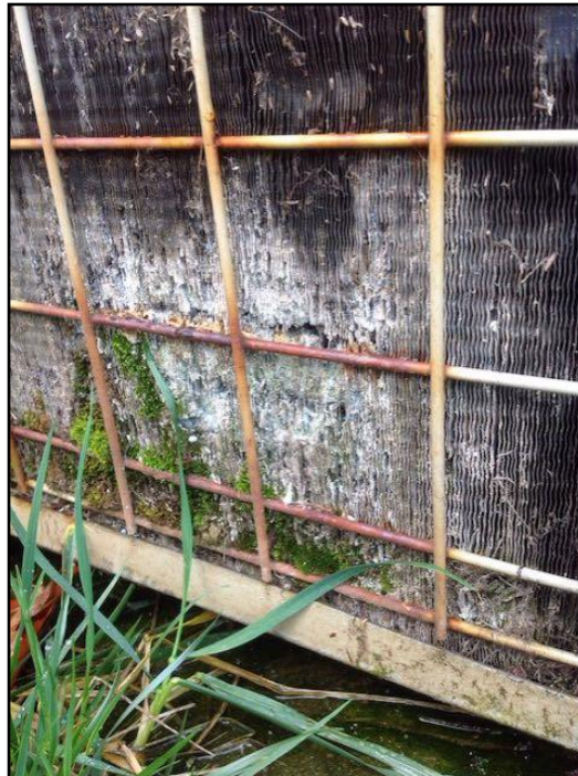
139. Corrosion
