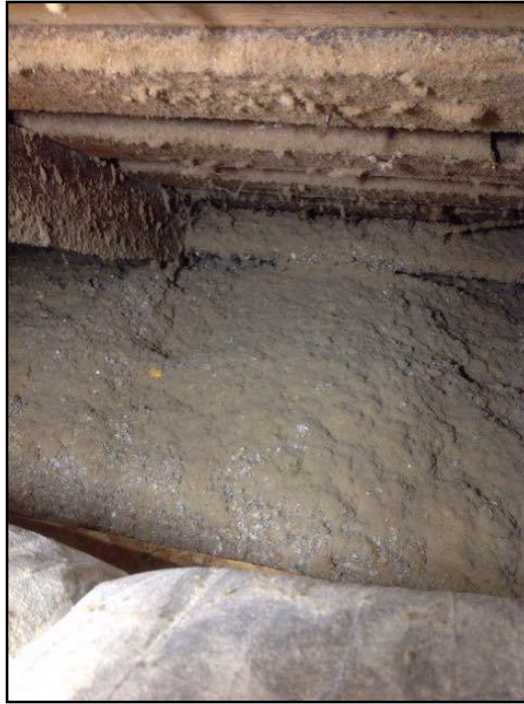
146. Blown-In Insulation
