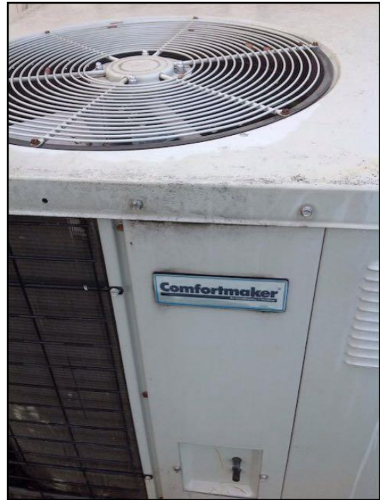
141. Heat Pump Downstairs Unit
