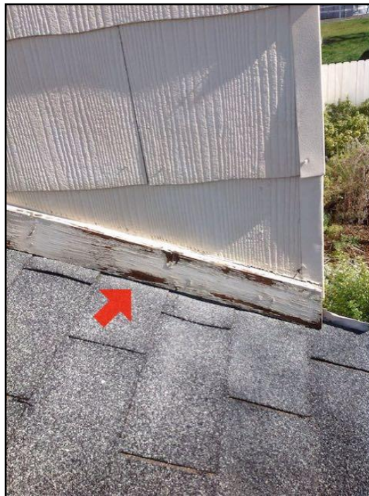
40. Improper Flashing
