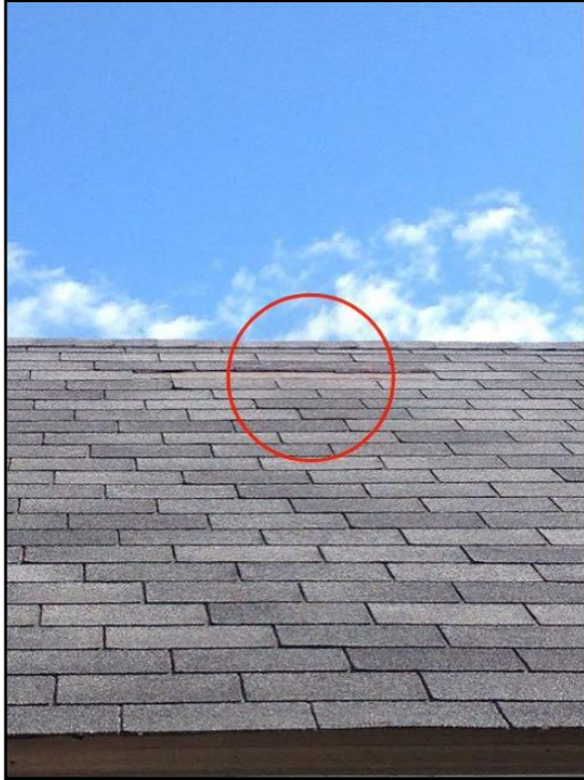
30. Missing Shingles
