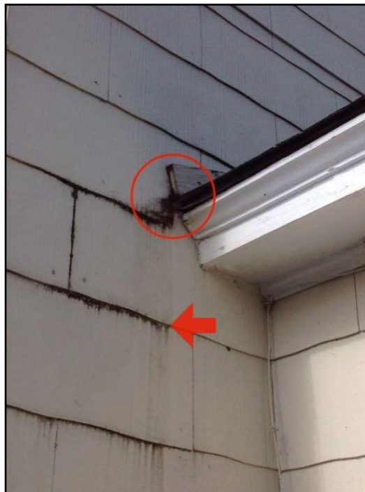
41. No kickout flashing
