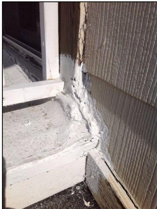
37. Questionable Flashing
