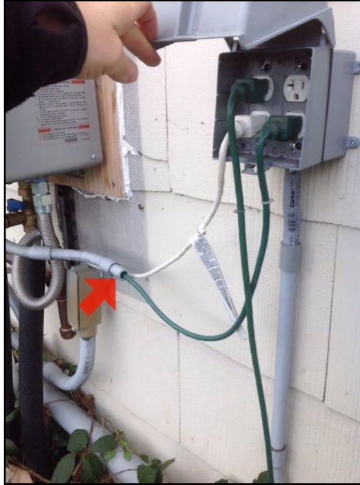
94. Extension cord used as permanent wiring
