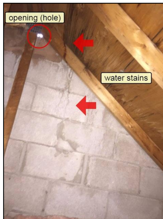
leak in attic
