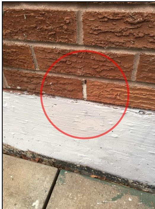
Weep holes obstructed
