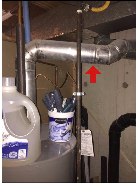
Vent Connector - slope inappropriate
