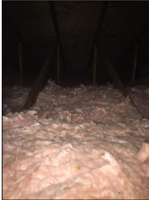
Insulation - compressed
