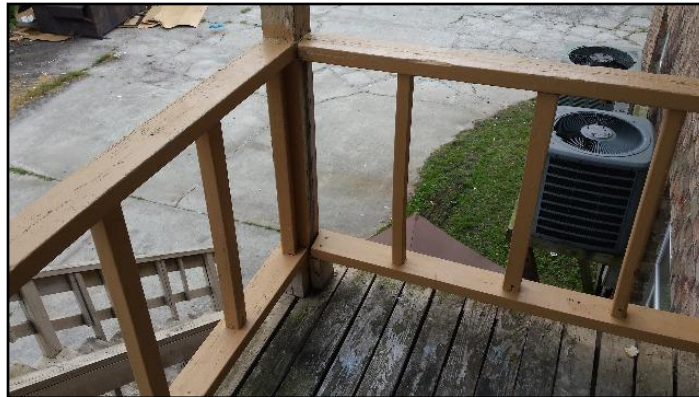
Openings between spindles (balusters) too...
