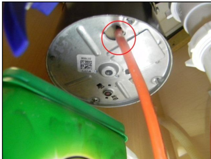
Loose connections
