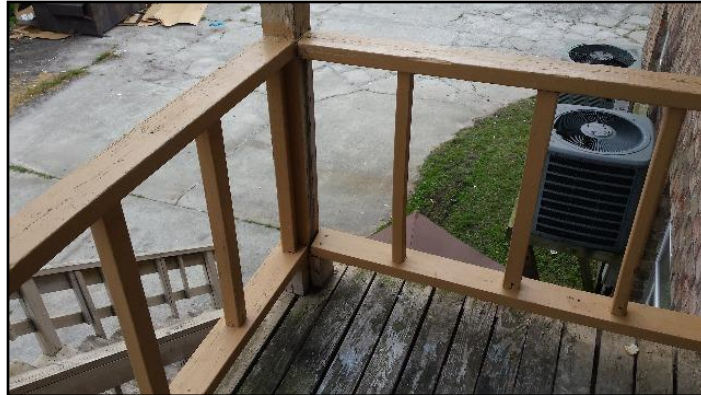
Openings between spindles (balusters) too...
