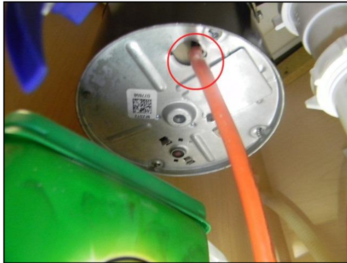
Loose connections
