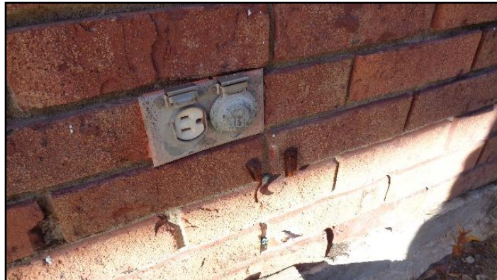
No GFCI/GFI (Ground Fault Circuit...
