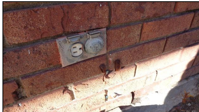
No GFCI/GFI (Ground Fault Circuit...
