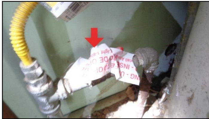
Improper connections
