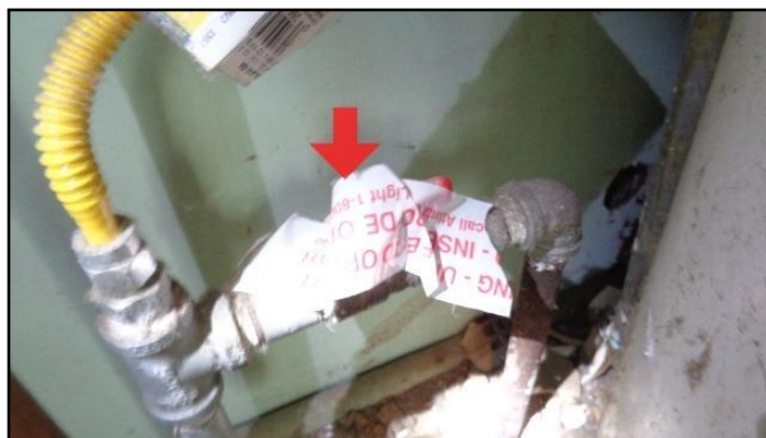
Improper connections
