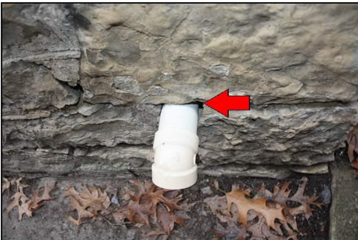
4. Caulking missing or ineffective
