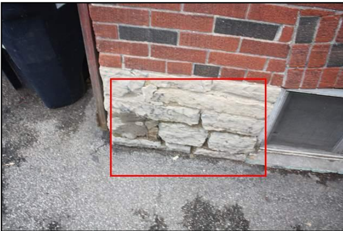
10. Mortar deterioration example at foundation
