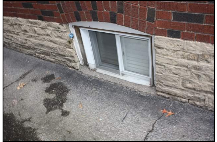
14. Window sill is at or below grade.
