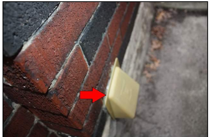
5. Caulking missing or ineffective
