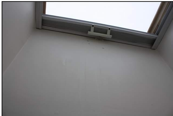
36. Condensation streaks on wall below skylight
