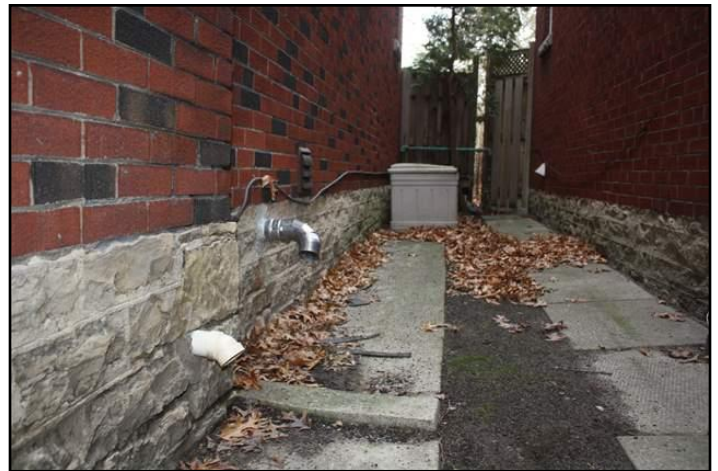
22. Improper slope or drainage
