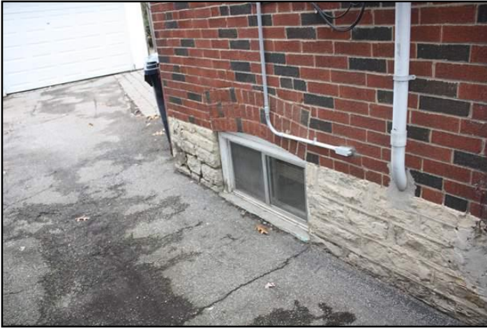
13. Window sill is at or below grade.
