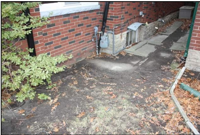
21. Improper slope or drainage
