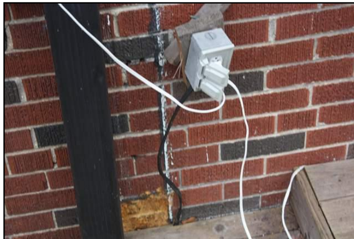
30. GFCI/GFI needed (Ground Fault Circuit...
