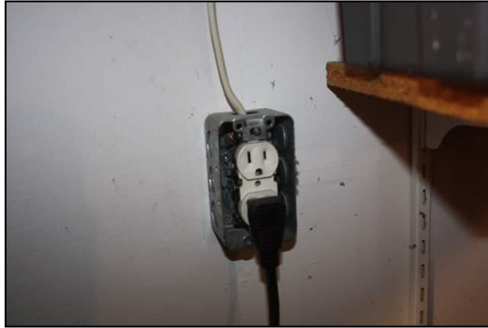
31. For outlet (receptacle) is missing
