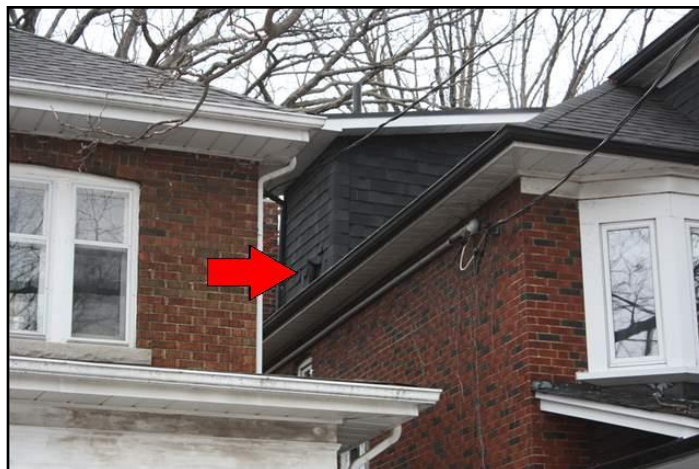
12. Loose, missing or torn tabs
