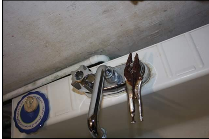
42. Handle damaged
