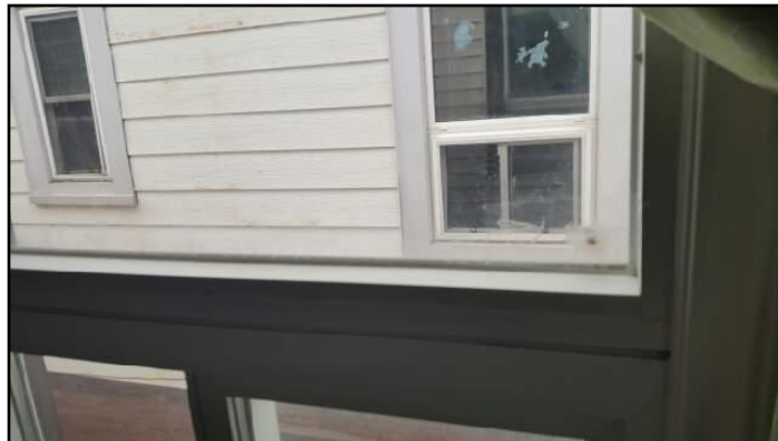
11. Lost seal on double or triple glazing
