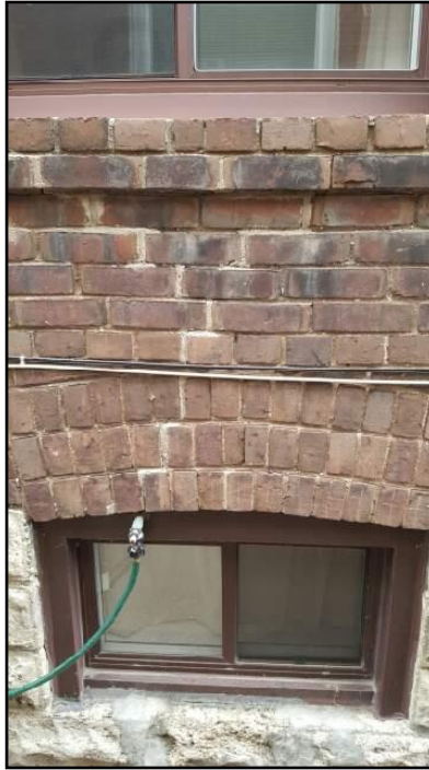
5. Typical minor crack
