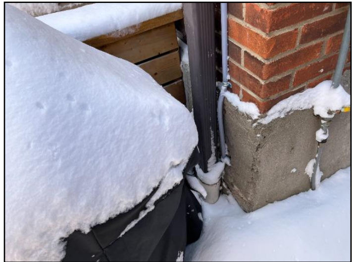
3. Downspouts below grade - Toronto. For more...
