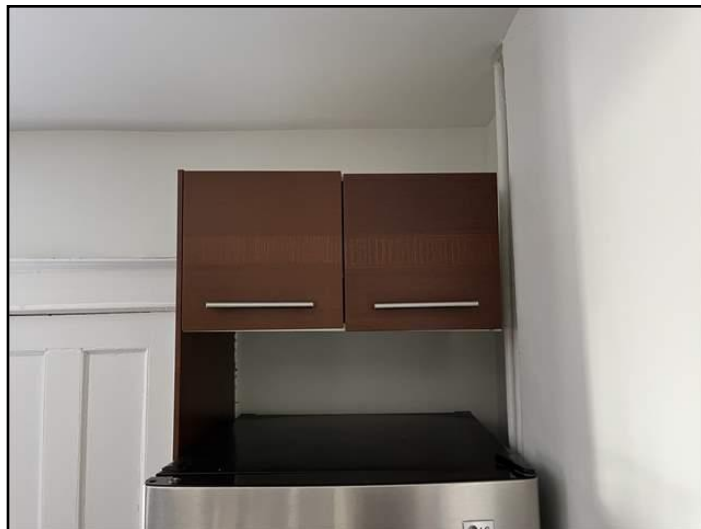
26. Not well secured to wall
