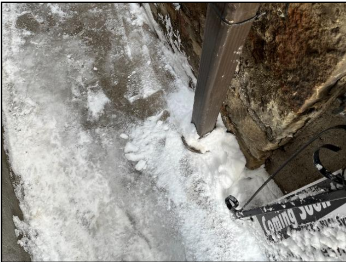
2. Downspouts below grade - Toronto. For more...
