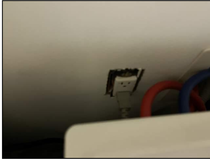
15. For outlet (receptacle) is missing
