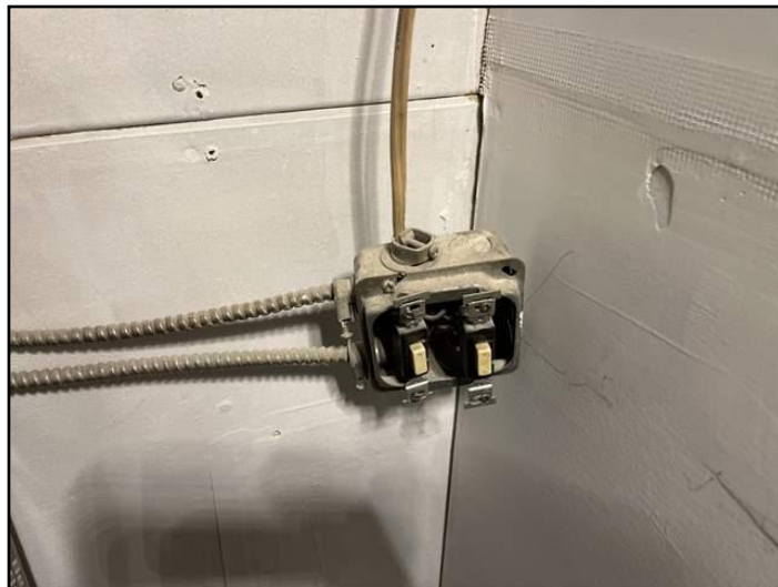
14. For switch is missing
