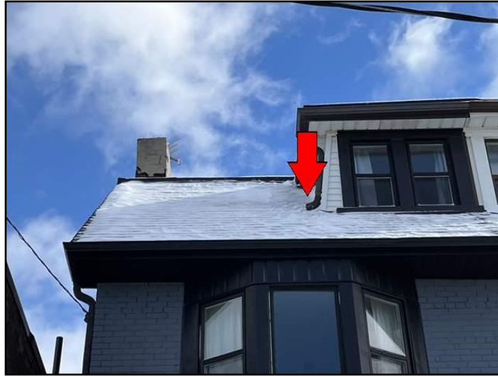
1. Discharge onto roofs
