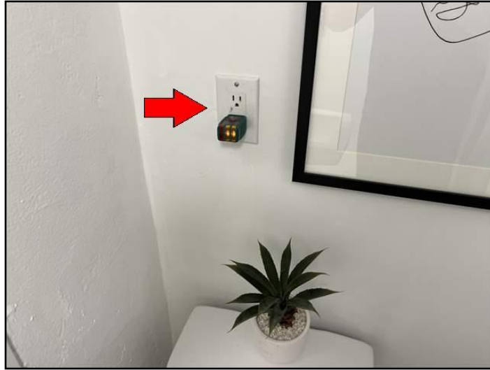
13. GFCI/GFI needed (Ground Fault Circuit...
