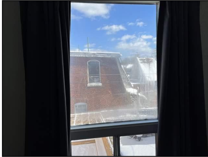
25. Lost seal on double or triple glazing
