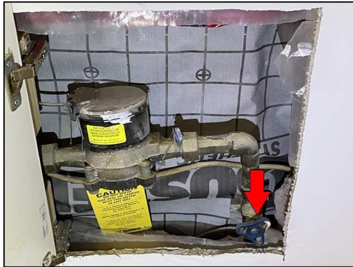
19. Main water shut off valve
