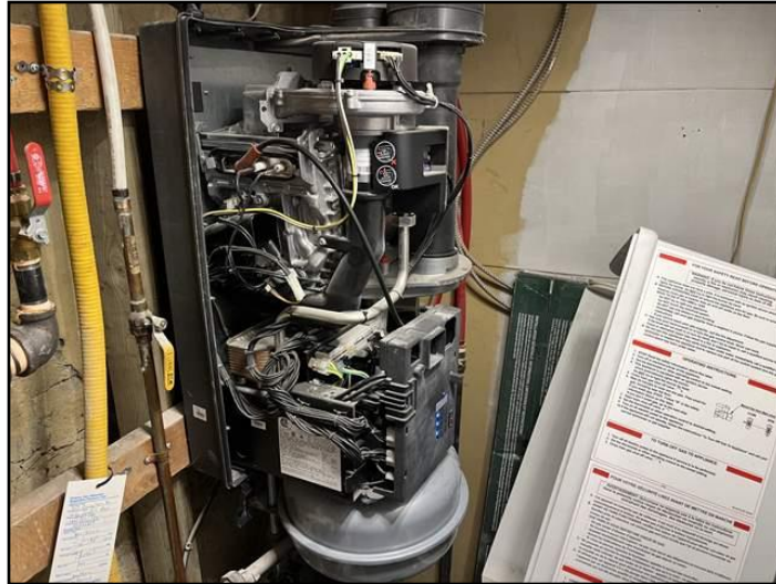
16. Boiler/Tankless with cover removed
