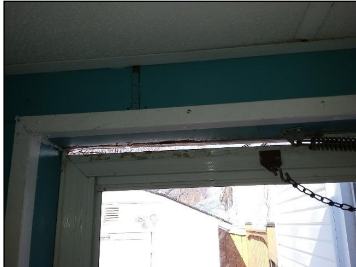
Deformation of door frame
