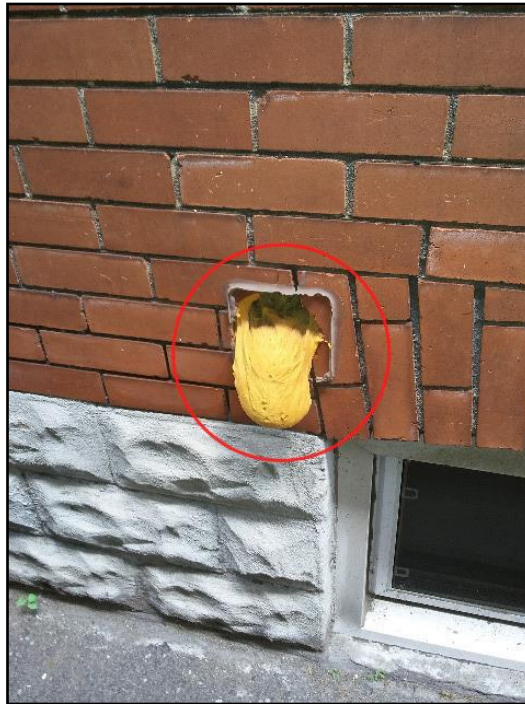
Abandoned dryer vent sealed improperly
