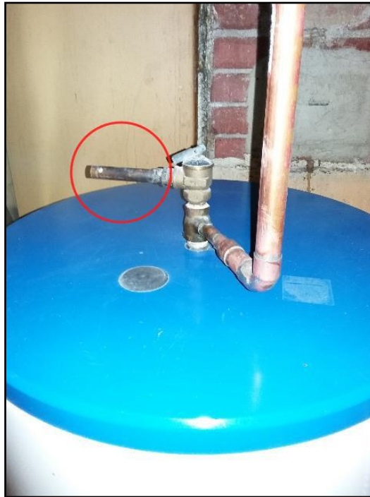
Discharge tube missing
