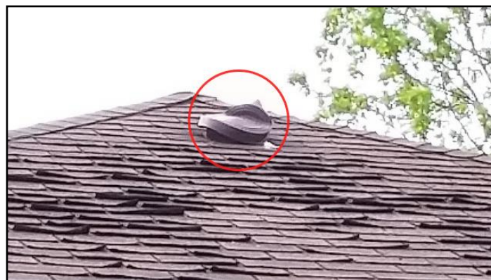
Damaged roof vent
