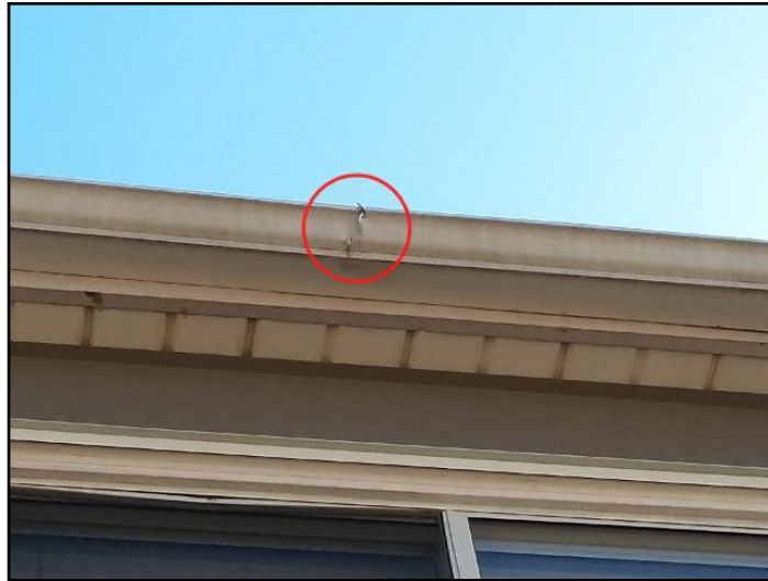
Damaged gutter
