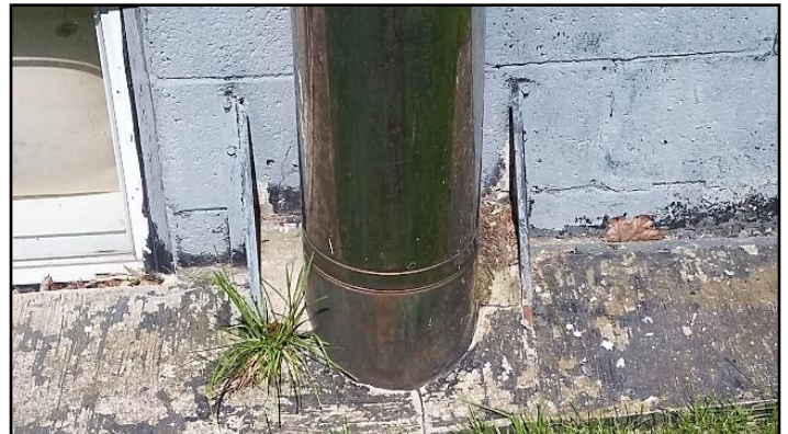
Chimney cleanout buried below ground
