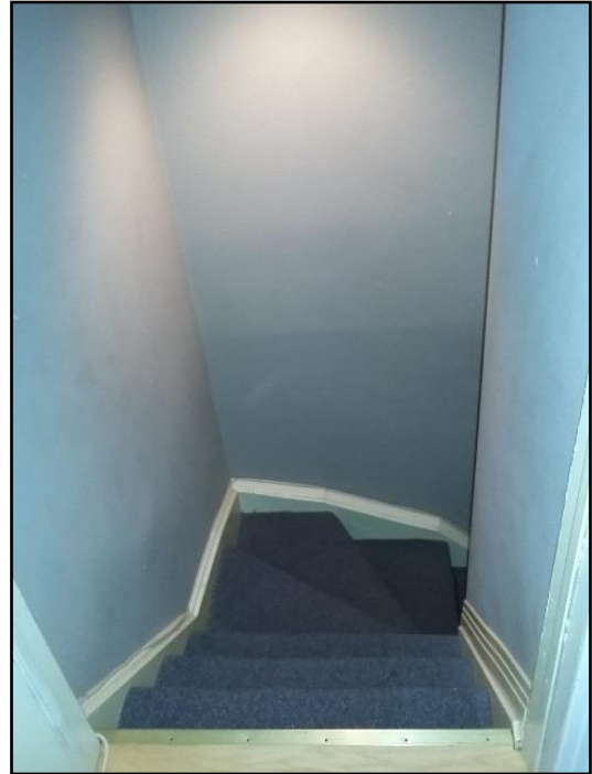
Missing handrails
