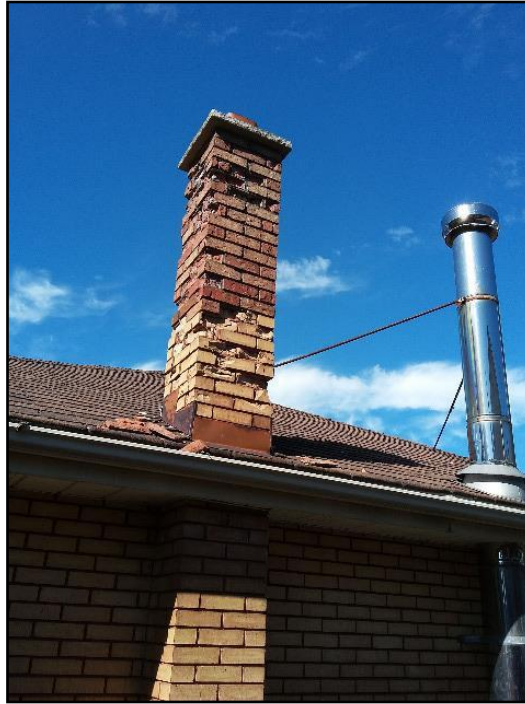
Loose, missing or deteriorated masonry
