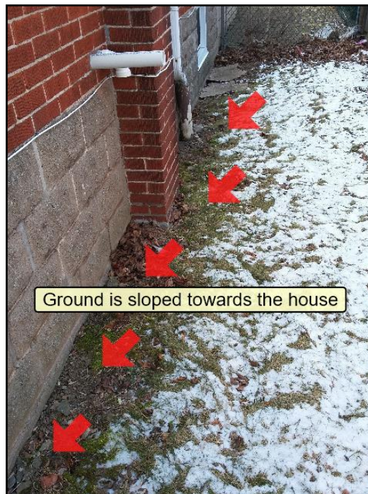
Improper slope or drainage
