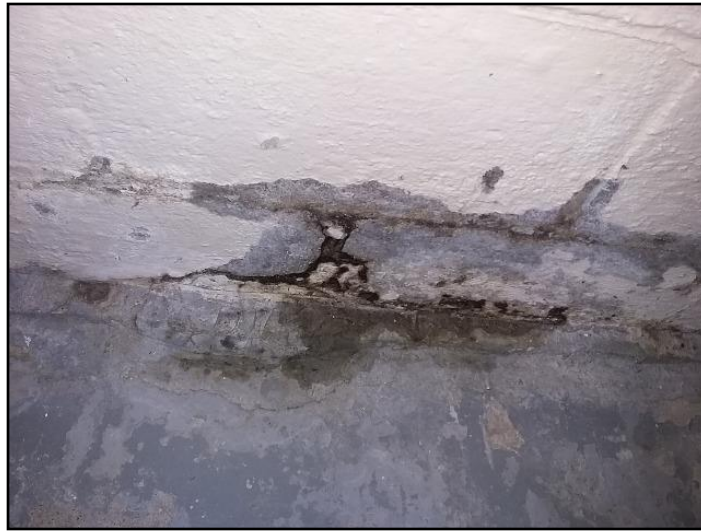
Leakage and apparent mold growth
