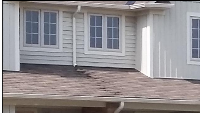
Downspout discharging onto roof
