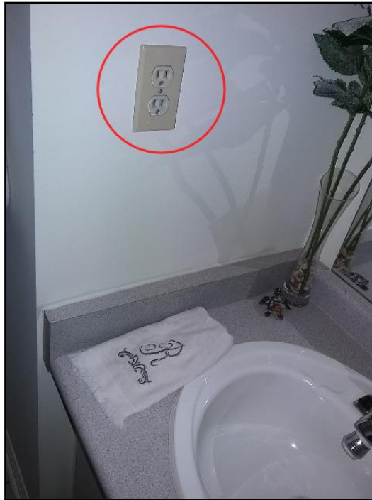
No GFCI/GFI in bathroom
