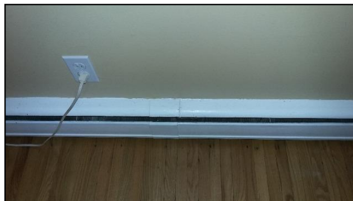
Electrical receptacle above baseboard heater
