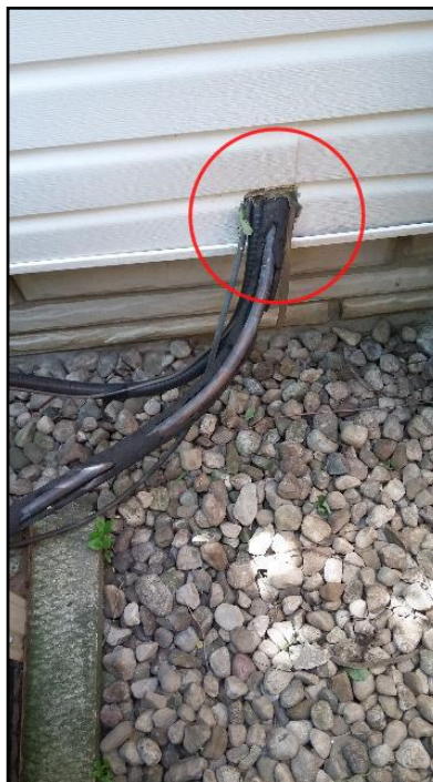
Missing electrical shutoff
