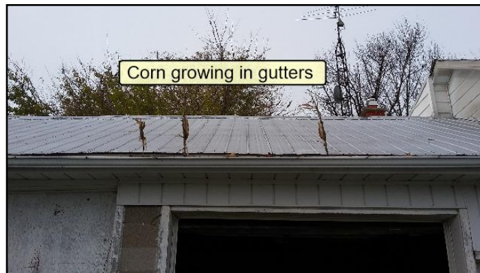
Dirt, debris & corn growing in gutters
