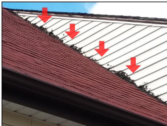
Leak sealed with roofing tar
