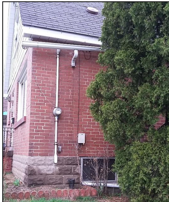
Missing downspout & loose gutter
