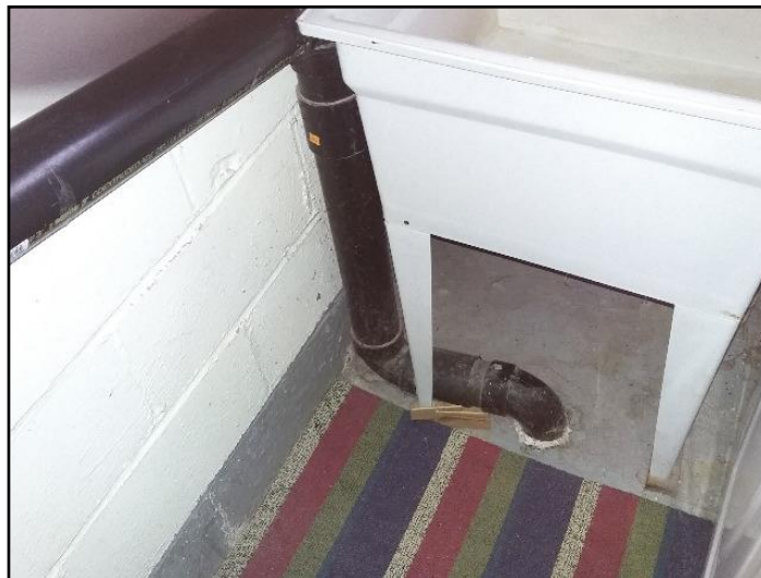
Waste pipe in floor drain
