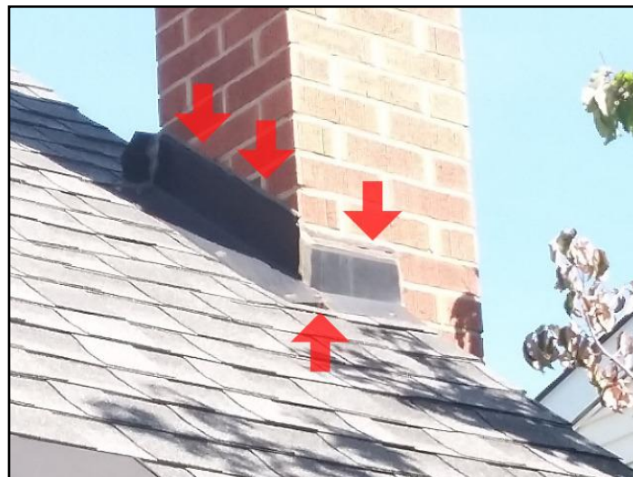
Failed caulking & lifted nail
