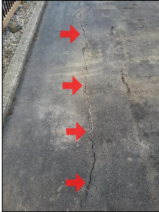
Cracks in asphalt driveway
