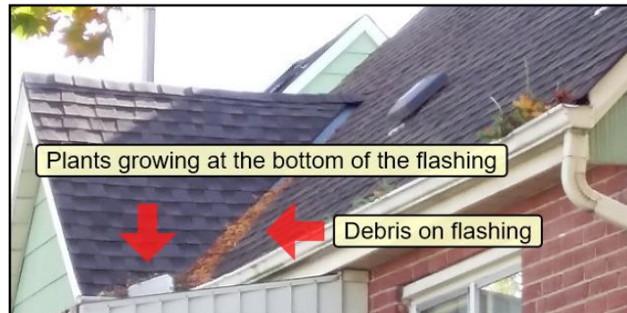
Debris & plants growing on flashing
