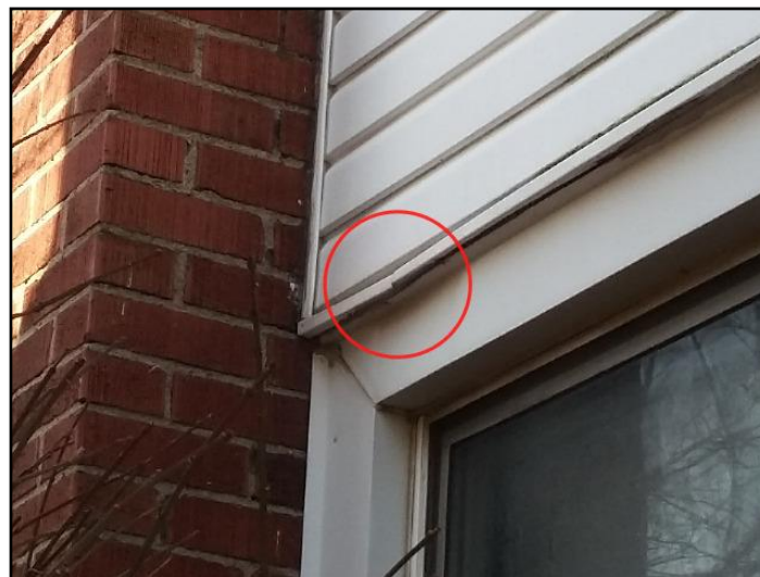
Inadequate flashing
