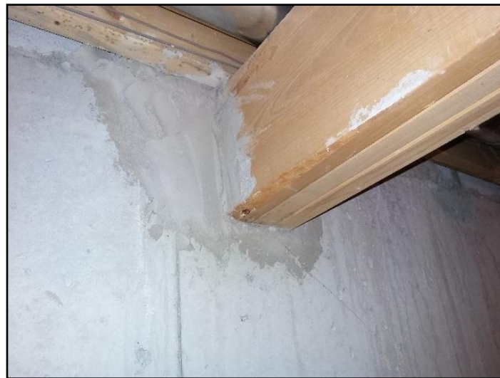
No air gap at the end of wood beam
