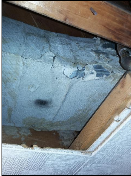
Suspected asbestos
