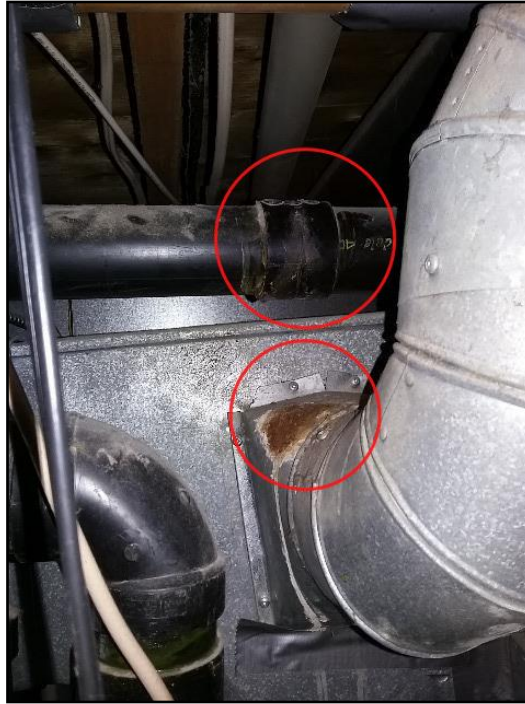
Leaking ABS piping
