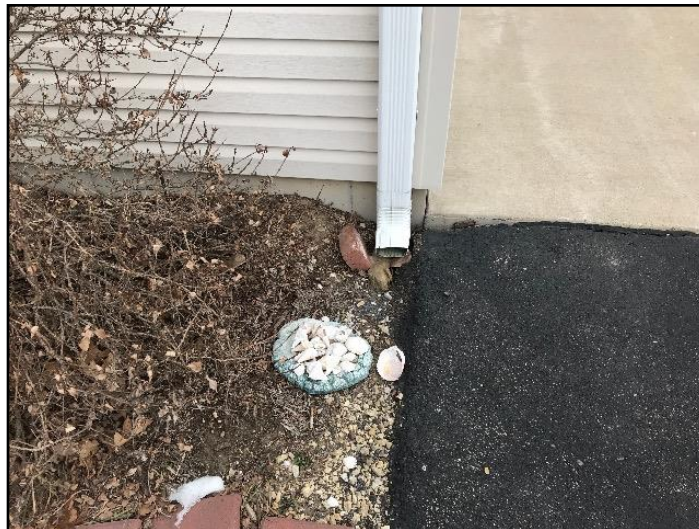
Should discharge 6 feet from building
