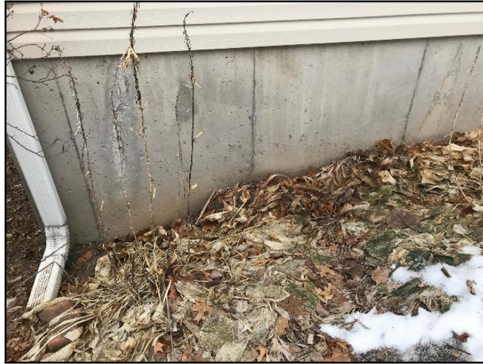
Improper slope or drainage
