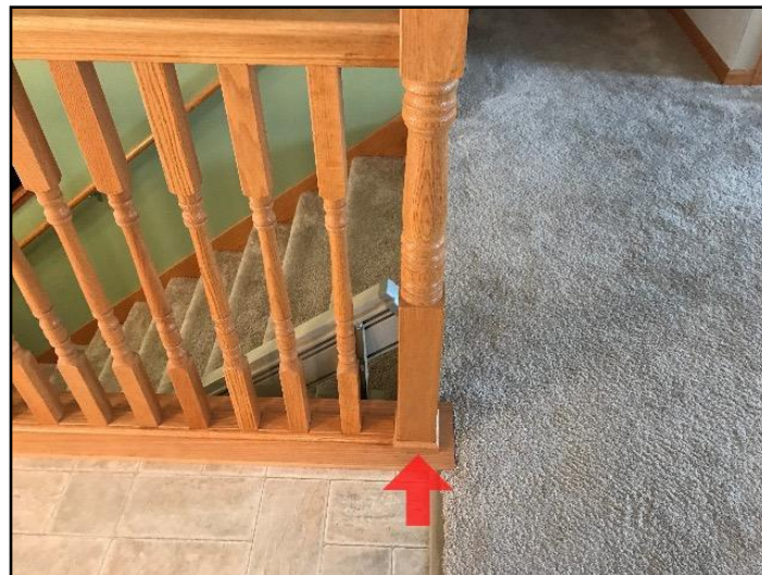
Loose guardrail post.
