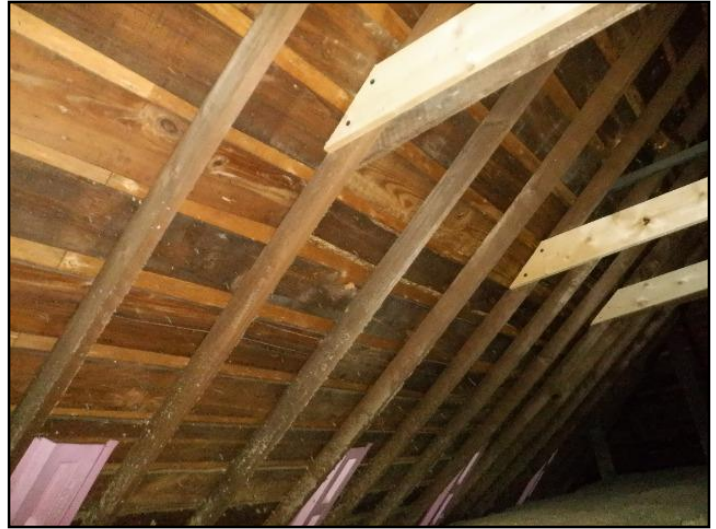
29. Roof Joists
