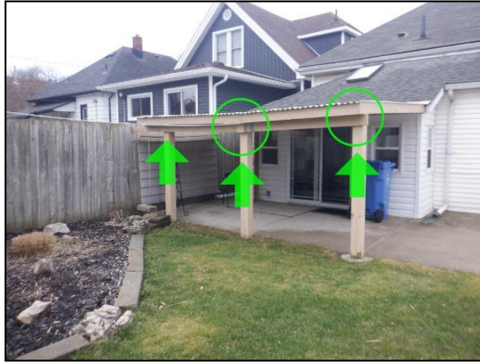
23. Reinforce header for snow loads
