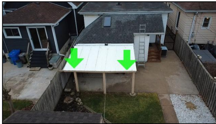
22. Install trough and downspout
