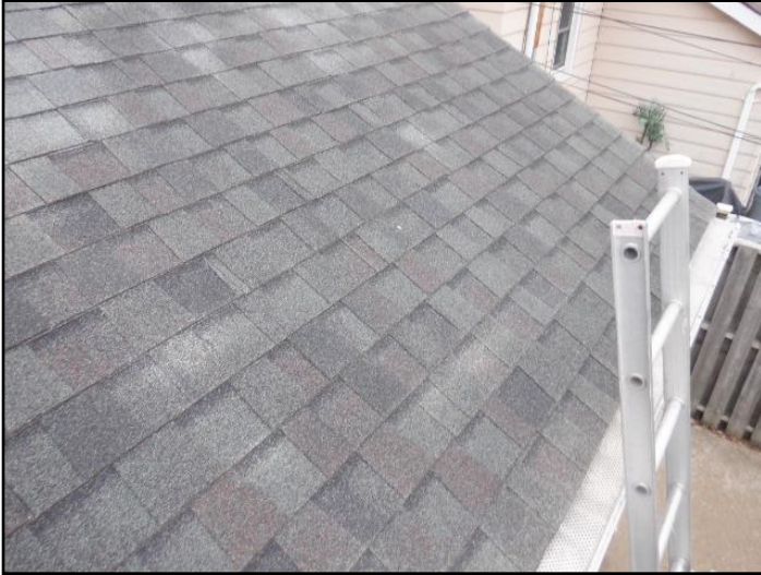
11. Roof Walked/ No Damage/ No Soft Spots
