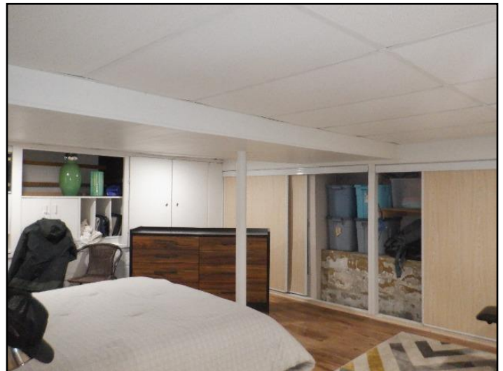
35. Ceiling, wall and floor coverings
