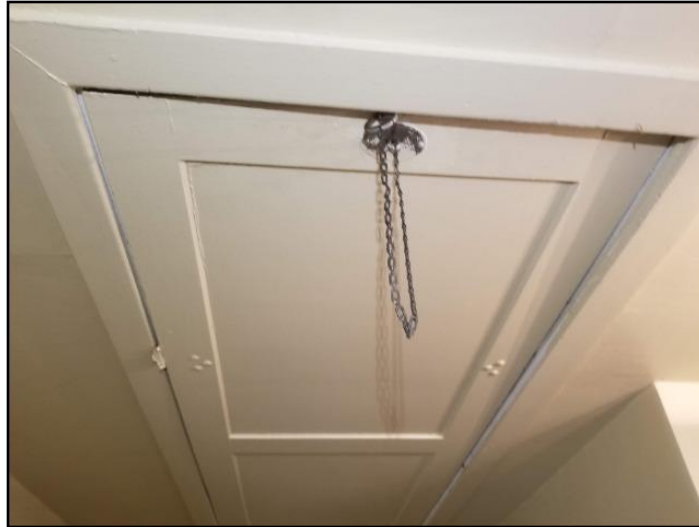
92. Not insulated and not weatherstripped
