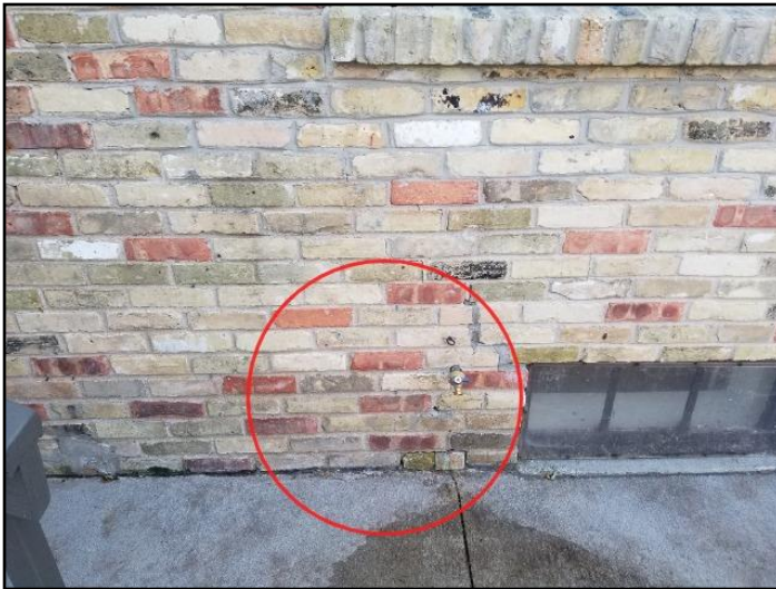
43. Mortar deterioration
