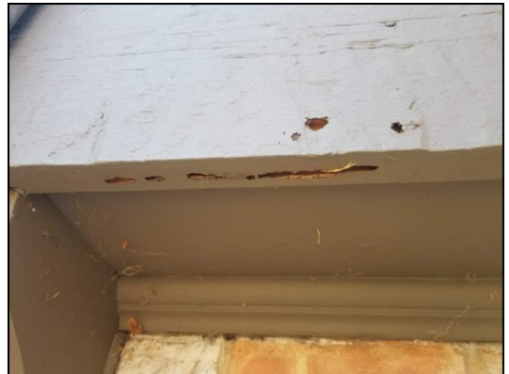
27. Rot or insect damage
