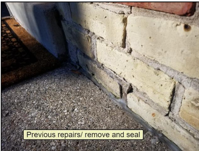
53. Improper slope or drainage
