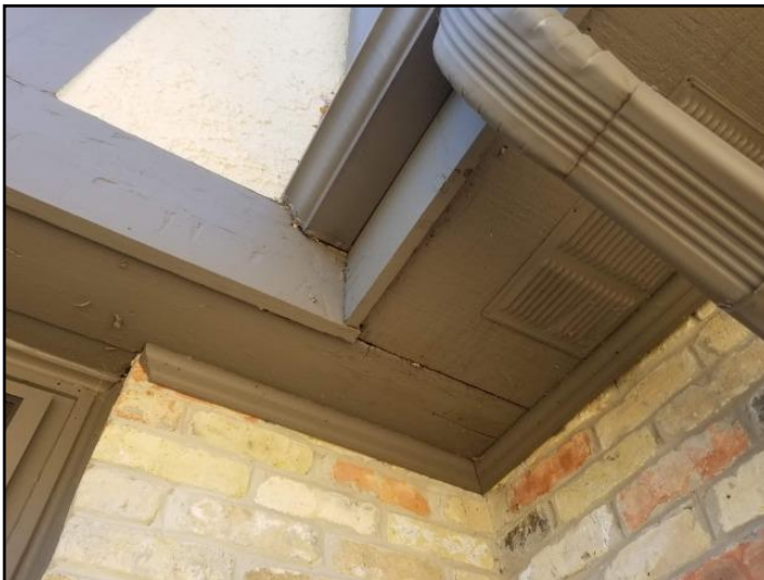
26. Rot or insect damage
