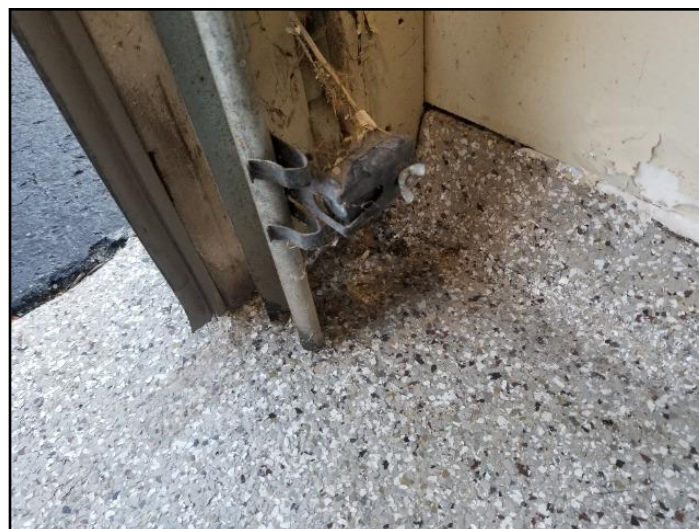
119. Sensors poorly located
