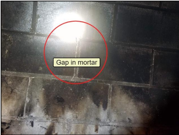
86. Deteriorated, missing or loose masonry or...
