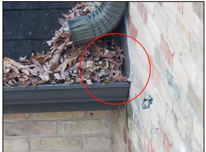
18. Kickout flashing - missing
