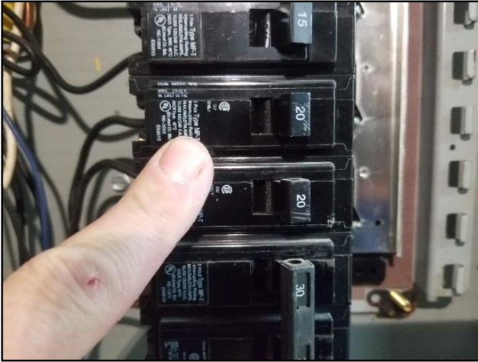
59. Breaker bridge missing
