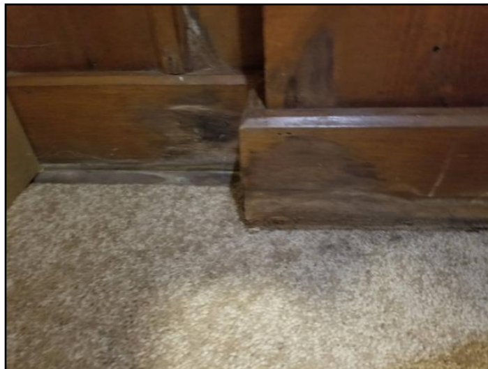
115. Water damage
