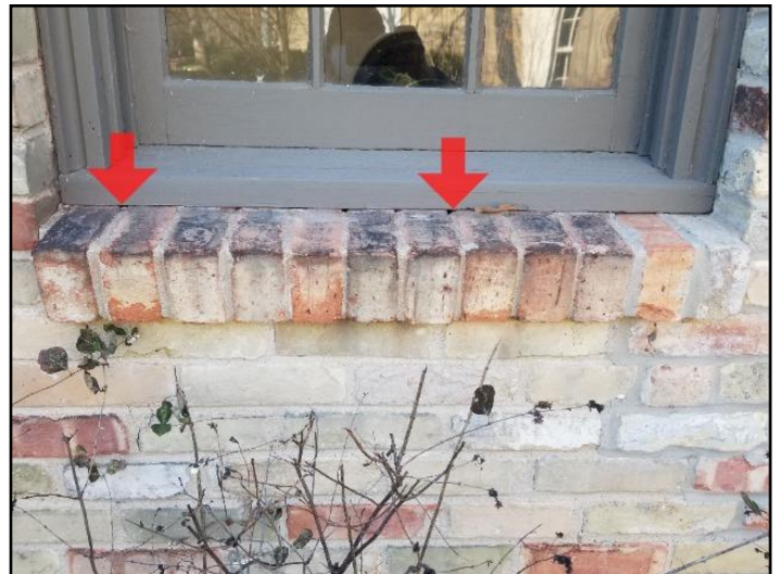
47. Caulking loose, missing or deteriorated
