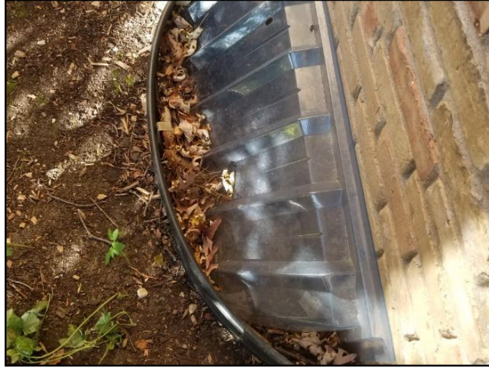
48. Clean out window wells of debris and dirt....
