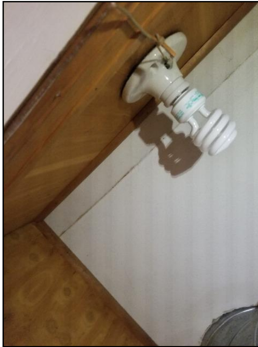
80. Improper closet lighting
