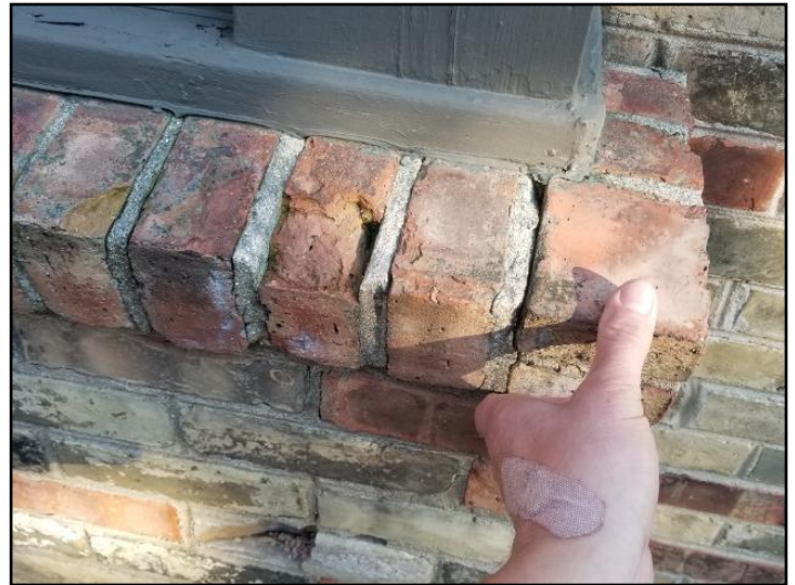
38. Masonry deterioration
