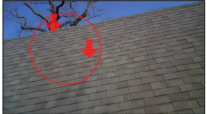
8. Nail Pop Have roofer or handyman correct...
