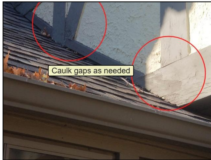
31. Caulking missing or deteriorated
