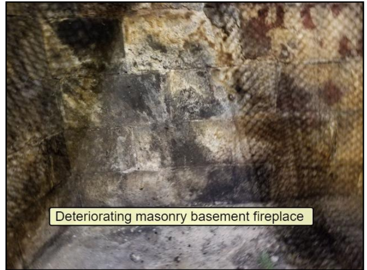
87. Deteriorated, missing or loose masonry or...
