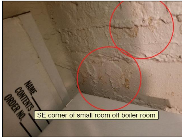
117. Efflorescence
