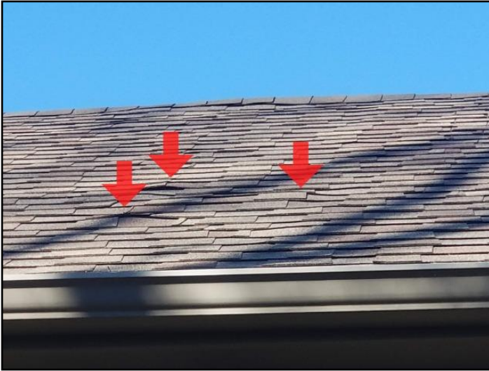
7. Nail Pop Have roofer or handyman correct...
