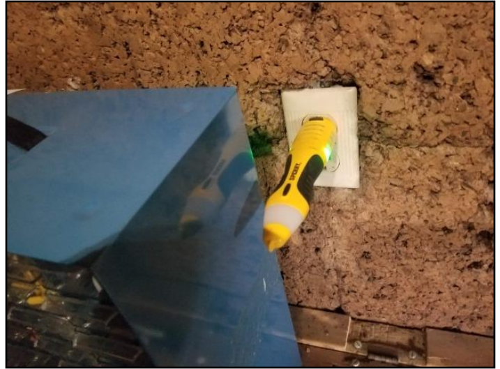
75. GFCI/GFI needed (Ground Fault Circuit...
