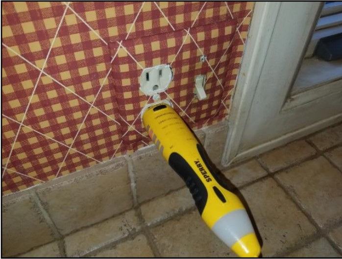
74. GFCI/GFI needed (Ground Fault Circuit...
