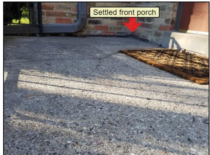
54. Improper slope or drainage
