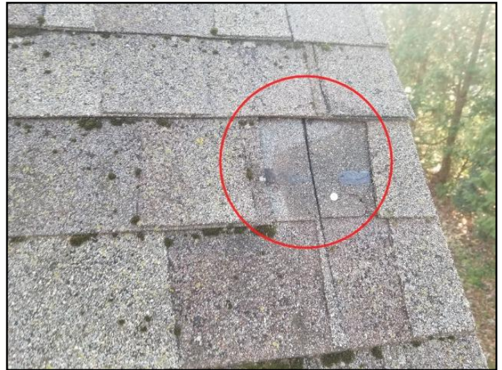
2. Missing, loose or torn
