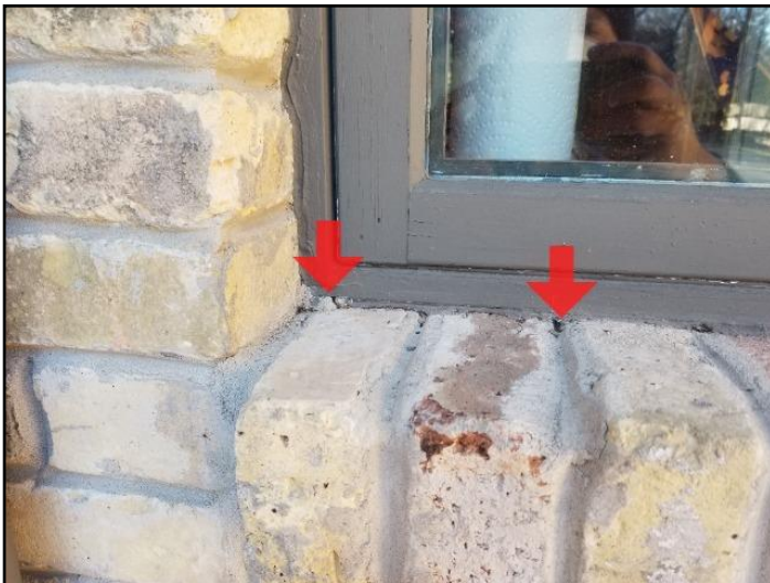
46. Caulking loose, missing or deteriorated
