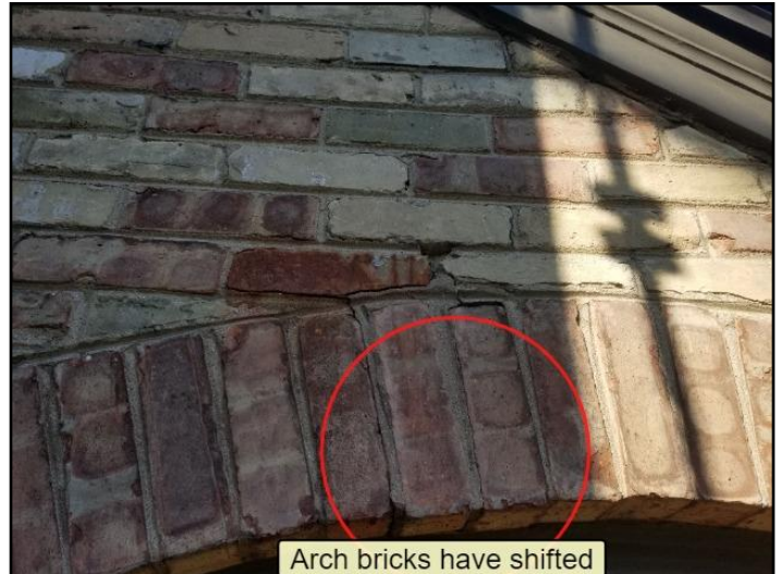
36. Masonry deterioration
