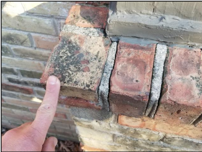
37. Masonry deterioration
