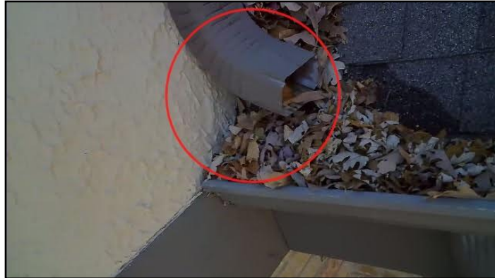
19. Kickout flashing - missing
