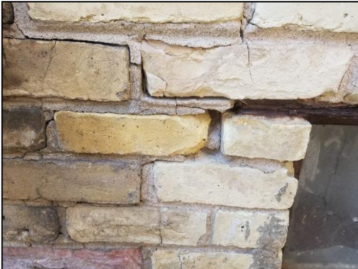
35. Masonry deterioration
