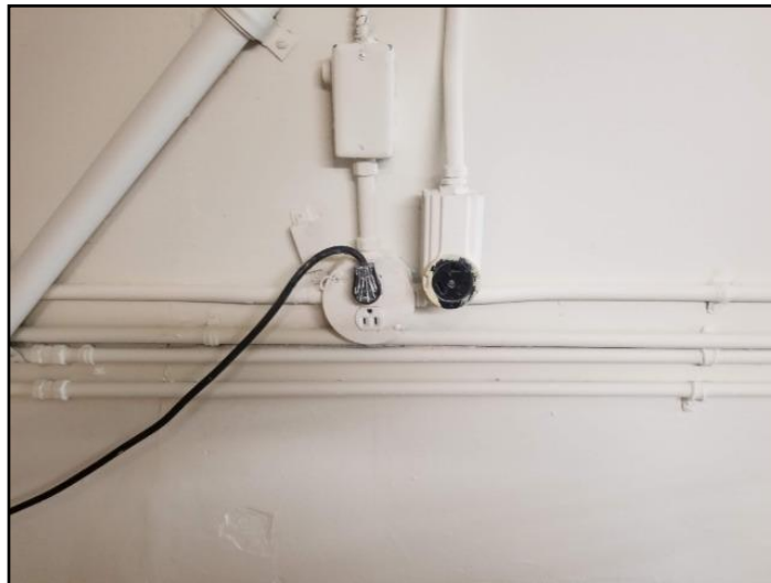
76. GFCI/GFI needed (Ground Fault Circuit...
