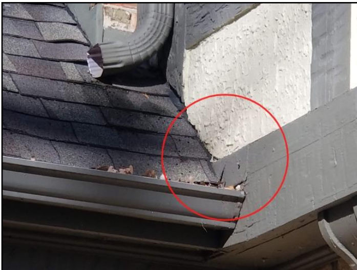
17. Kickout flashing - missing
