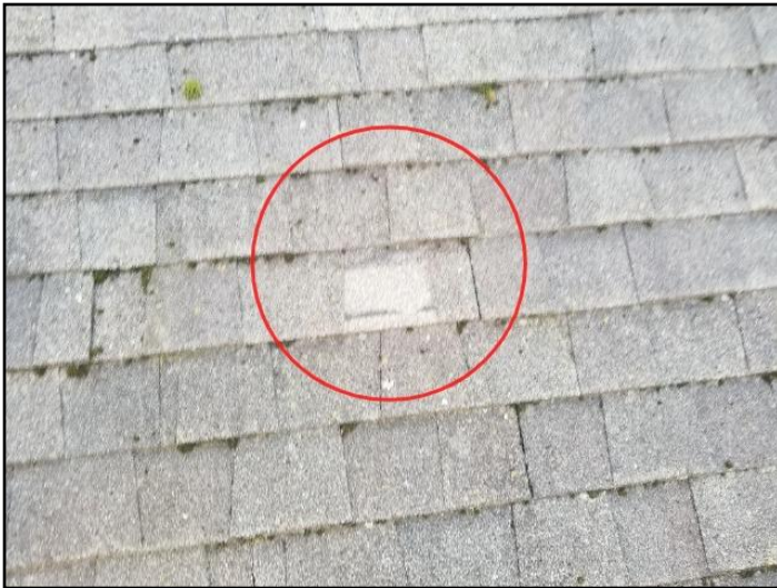
1. Missing, loose or torn
