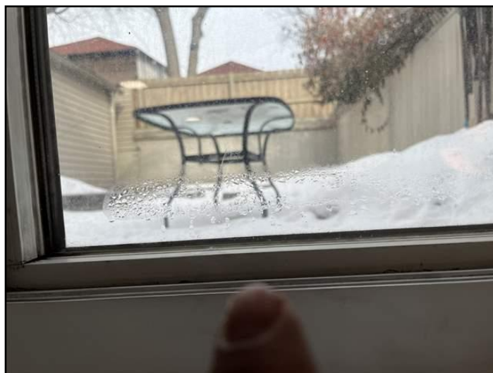
15. one example of lost seal
