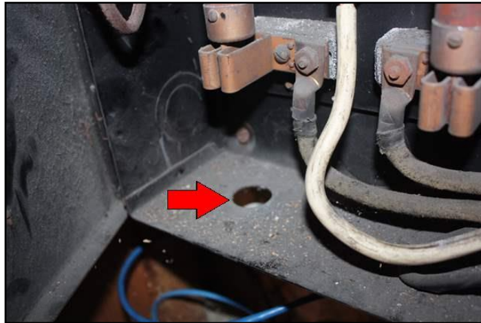
10. Unprotected openings
