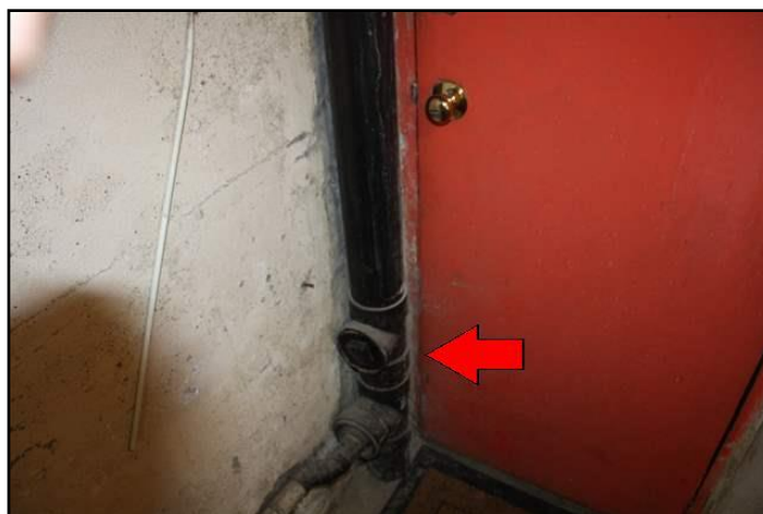
18. Loose or poor fit
