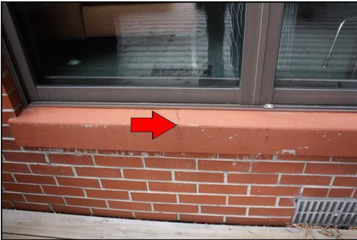
7. Minor sill cracks
