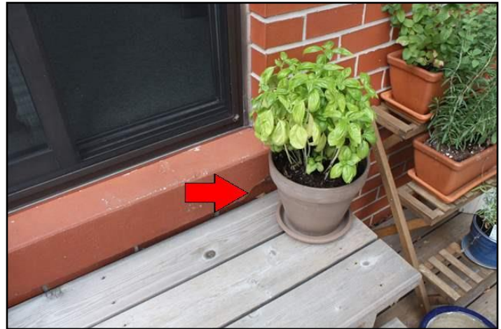
8. Sill deteriorated
