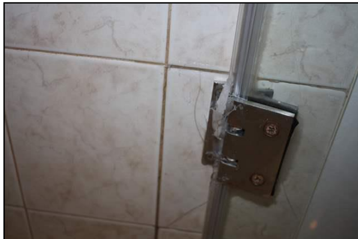
8. Tile loose, broken or missing tile
