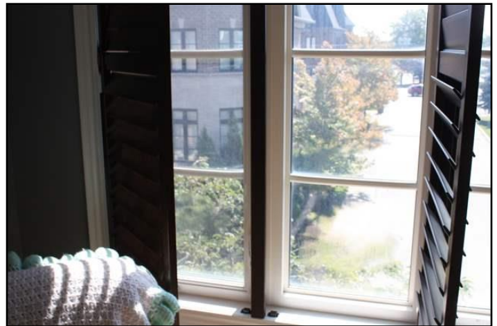
13. Lost seal on double or triple glazing
