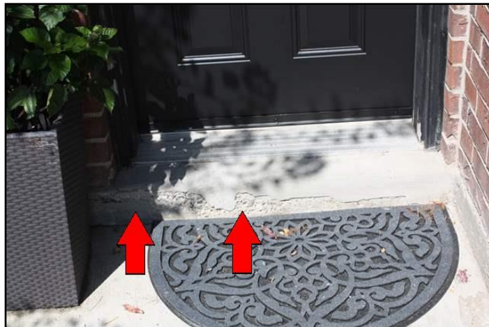
3. Parging damaged or missing
