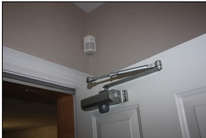
4. Self-Closer Damaged.
