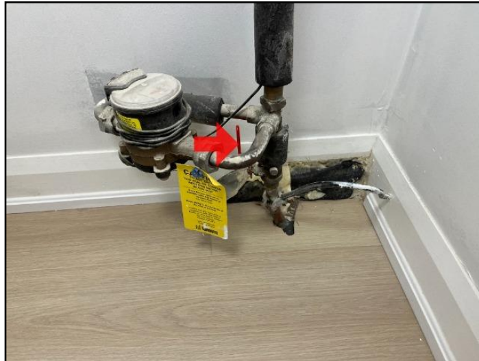
22. main water shut off valve
