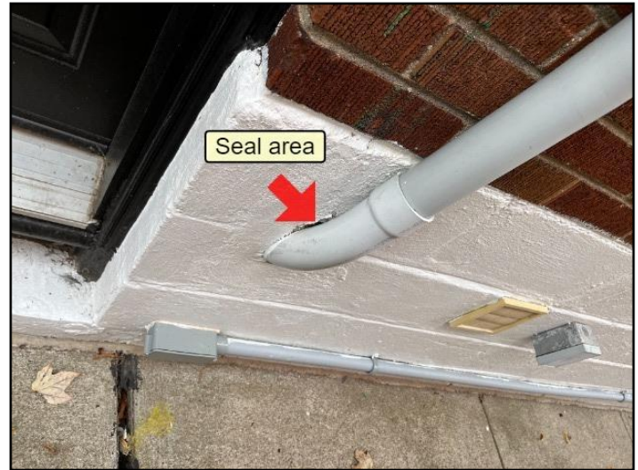
5. Caulking missing or ineffective
