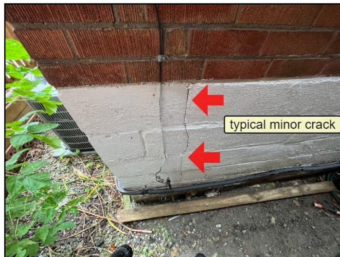
9. Example of typical minor crack
