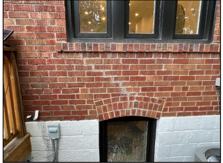
11. Cracks or prior repairs
