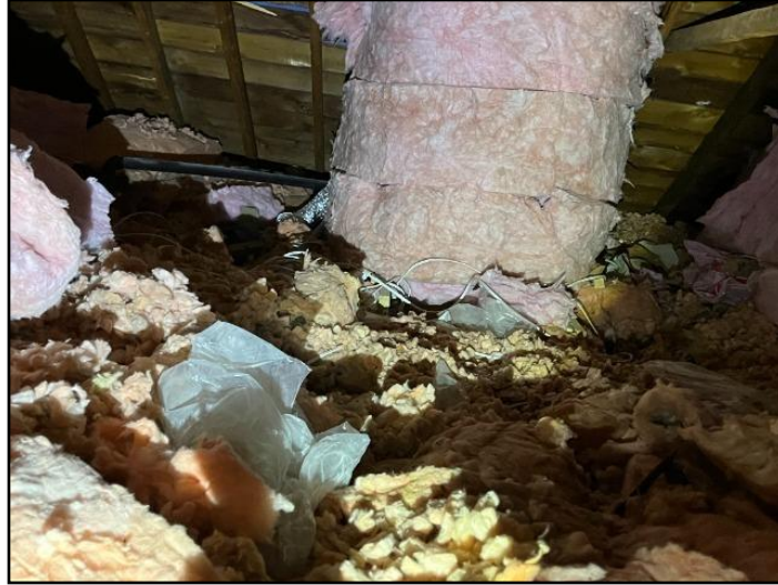
18. Exposed wiring in attic
