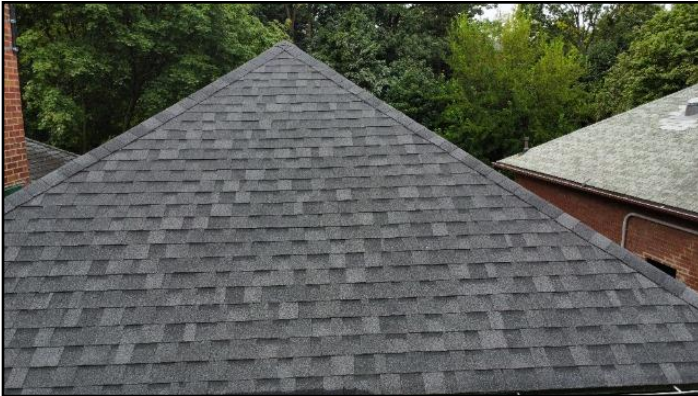
1. Asphalt shingles
