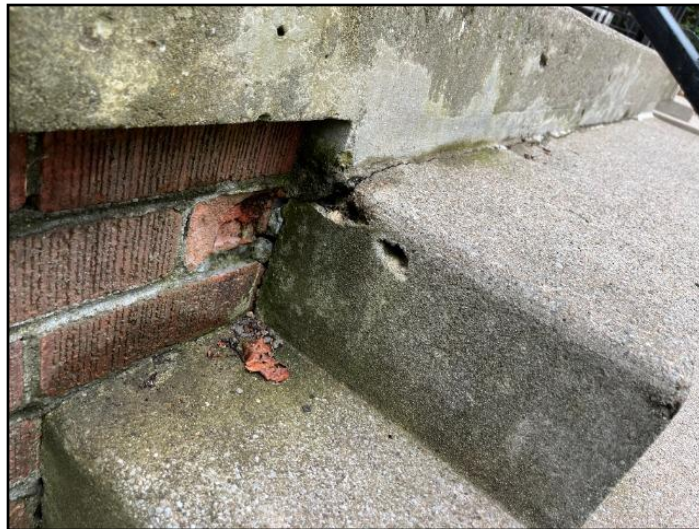
7. example of spalled area
