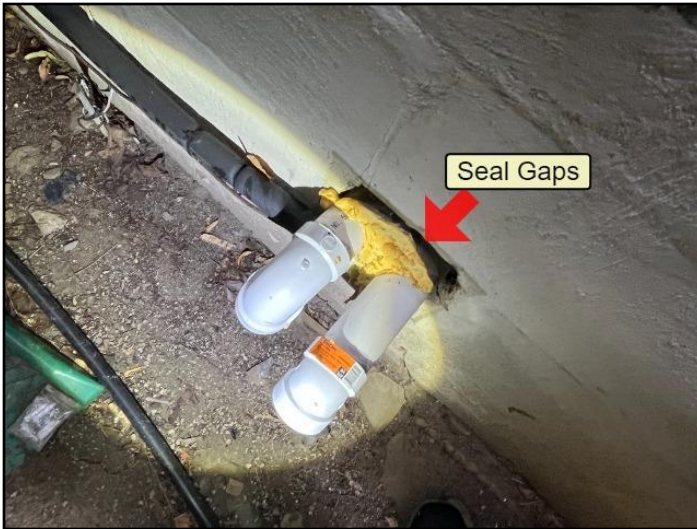
4. Caulking missing or ineffective
