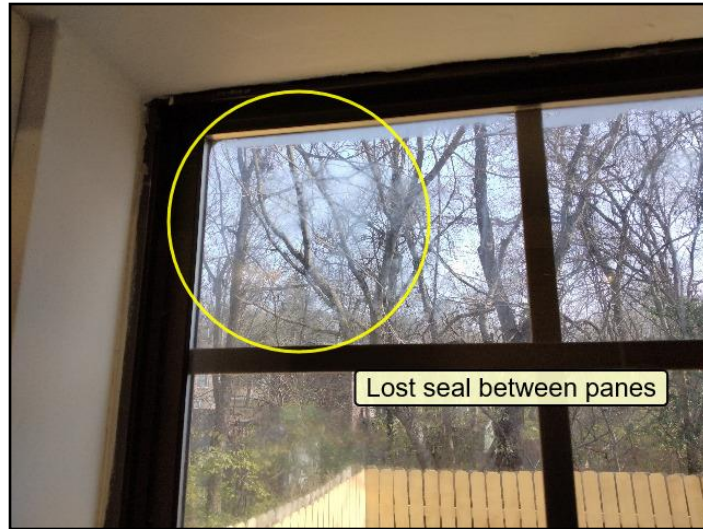
Lost seal on double or triple glazing
