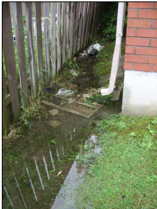
Downspouts end too close to building
