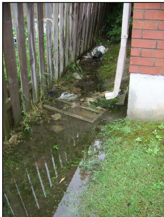
Downspouts end too close to building
