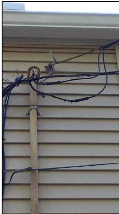
Damaged, frayed wires
