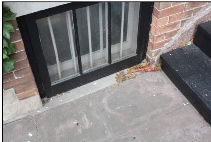
Sill - clearance inadequate (above grade...
