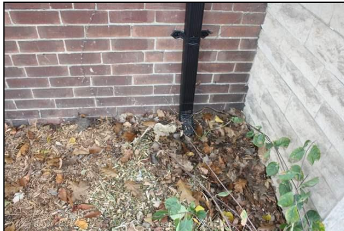
Discharge too close to Foundation (should...
