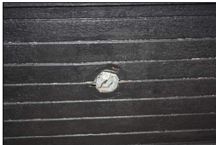
Missing on junction boxes
