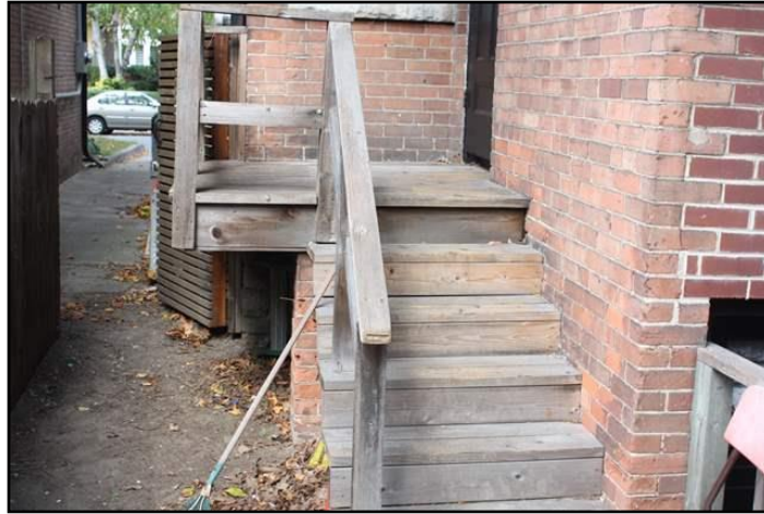
Boards poorly supported
