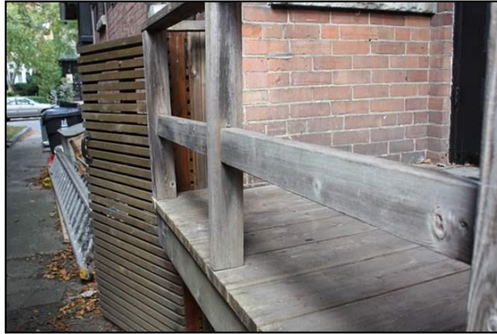
Railing not secure
