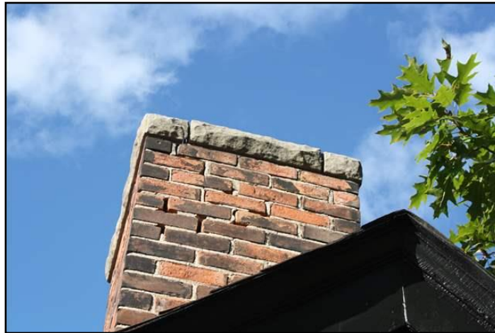
Abandoned (vulnerable area for leaks)
