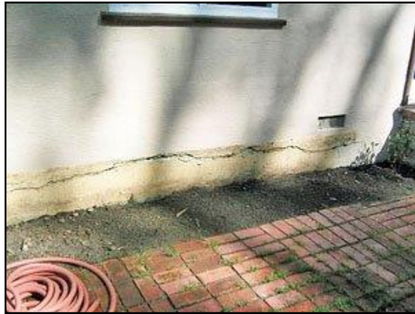
19. Cracked horizontally
