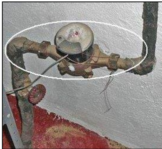
8. No jumper for meters and valves
