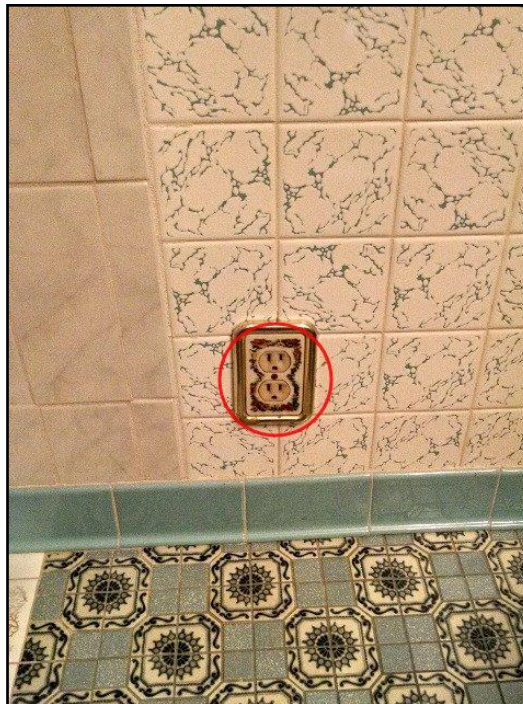
9. No GFCI (Ground Fault Circuit Interrupter)
