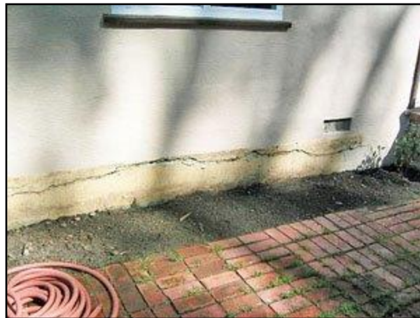
7. Cracked horizontally
