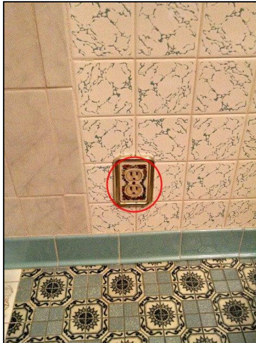
21. No GFCI (Ground Fault Circuit Interrupter)
