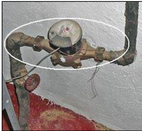
20. No jumper for meters and valves
