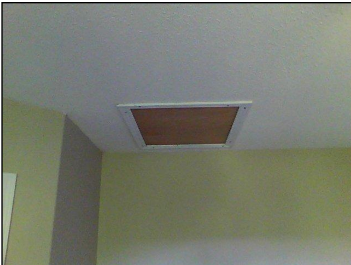
34. Not insulated and not weatherstripped
