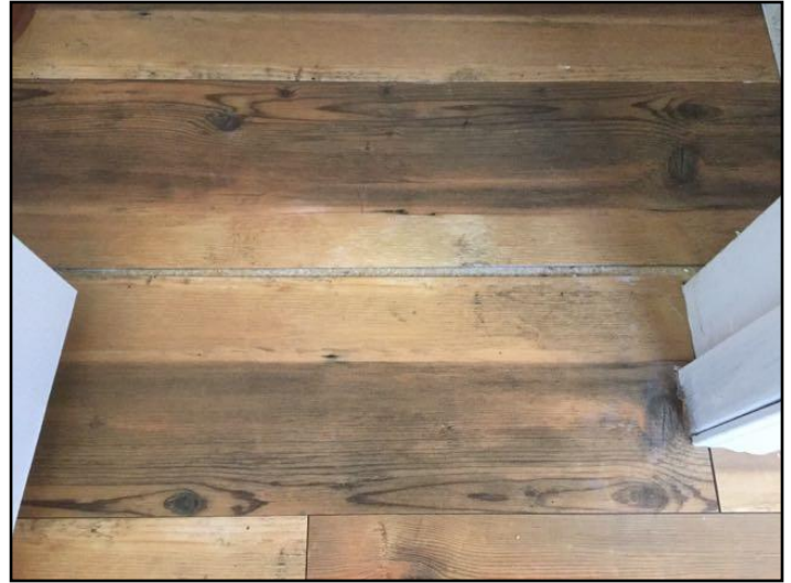
46. Loose or missing sections
