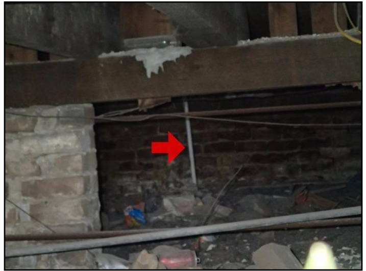
64. Improper discharge point
