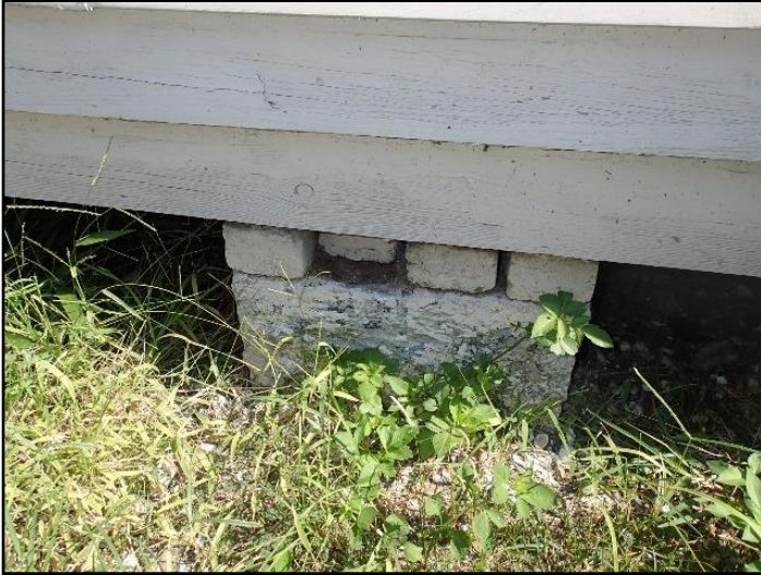
25. Loose or missing bricks.
