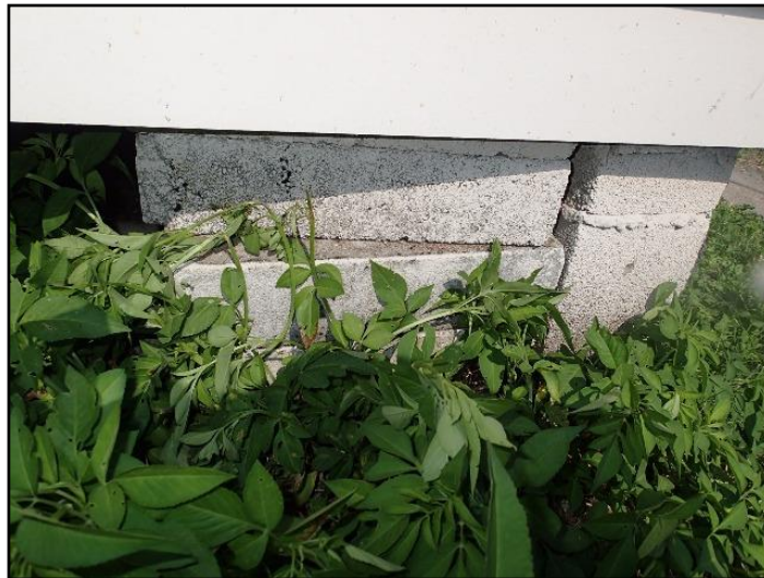
27. Loose or missing bricks.
