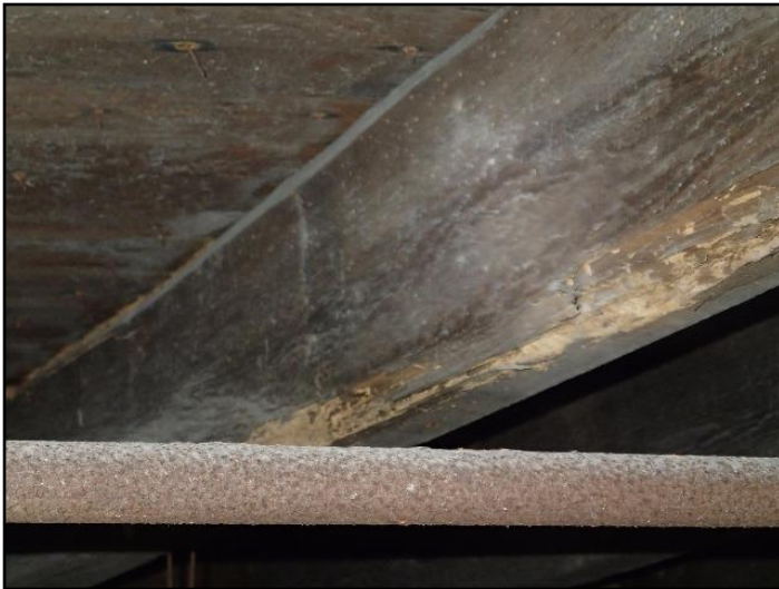
31. Rot, insect or fire damage
