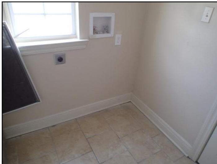
92. Dryer not vented to exterior
