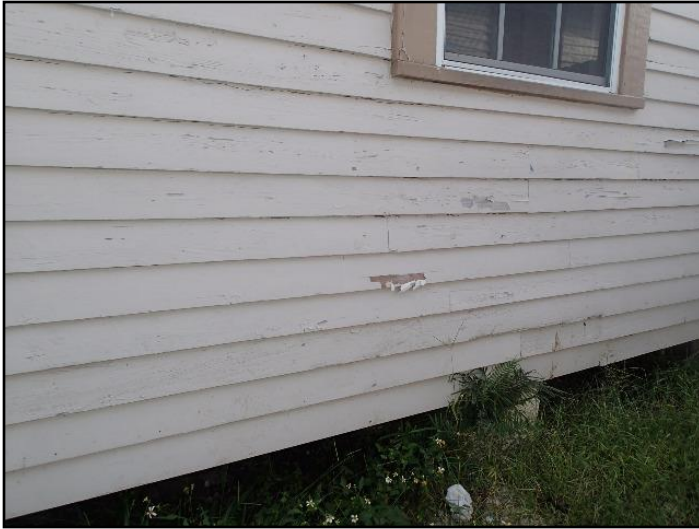
9. Peeling paint on exterior wood surfaces....
