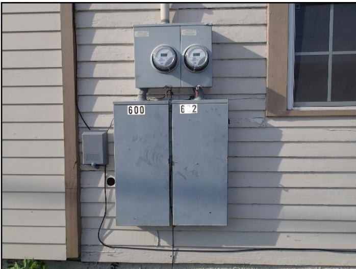
38. Combination panel - cover on
