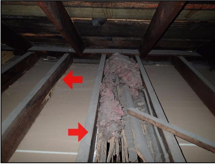
33. Damaged ceiling joist
