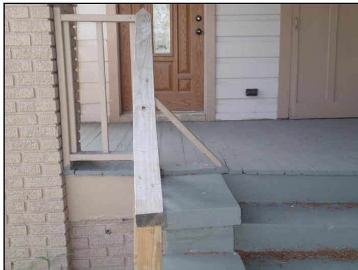
20. Handrails should be easy to grasp.
