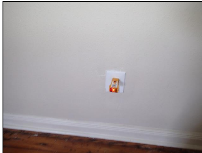
47. Reversed polarity
