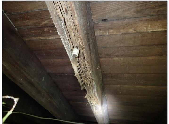
32. Rot, insect or fire damage
