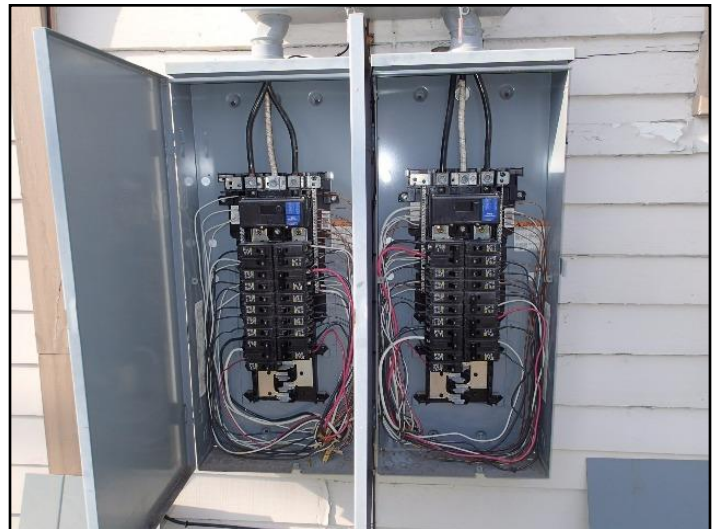
39. Combination panel - Cover removed
