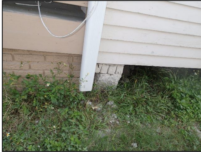
14. No diverter at end of downspout
