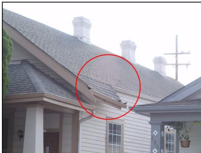
24. Falling roof/framing
