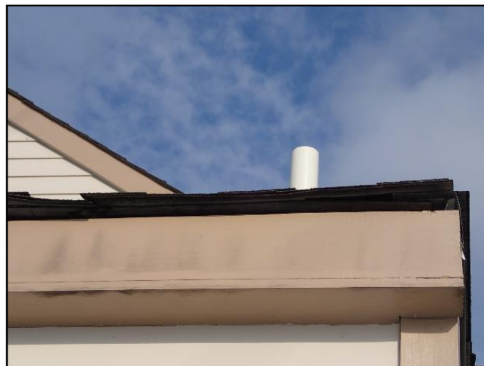
8. Missing drip edge flashing
