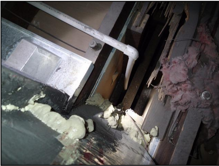
63. Improper discharge point
