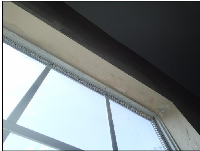
79. Water damage
