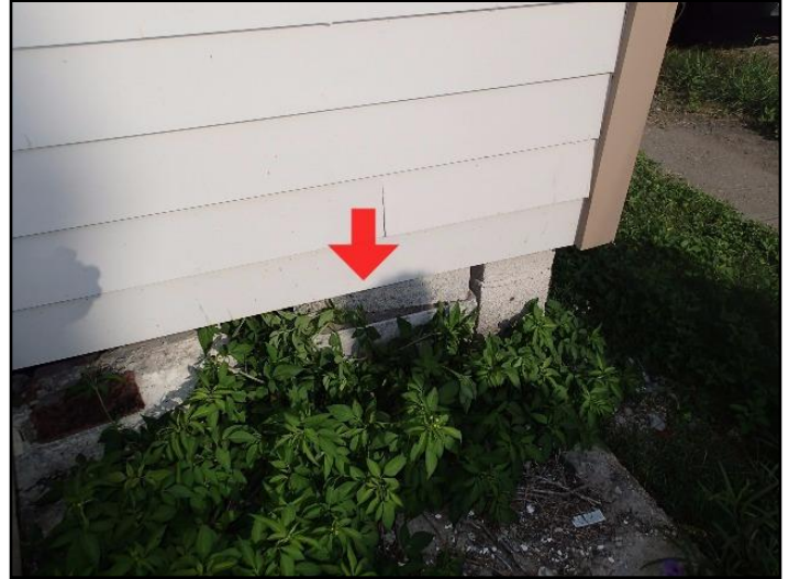
26. Loose or missing bricks.
