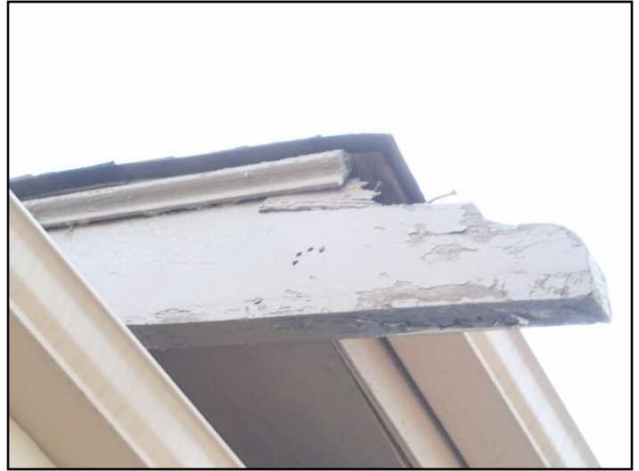
10. Peeling paint on exterior wood surfaces....
