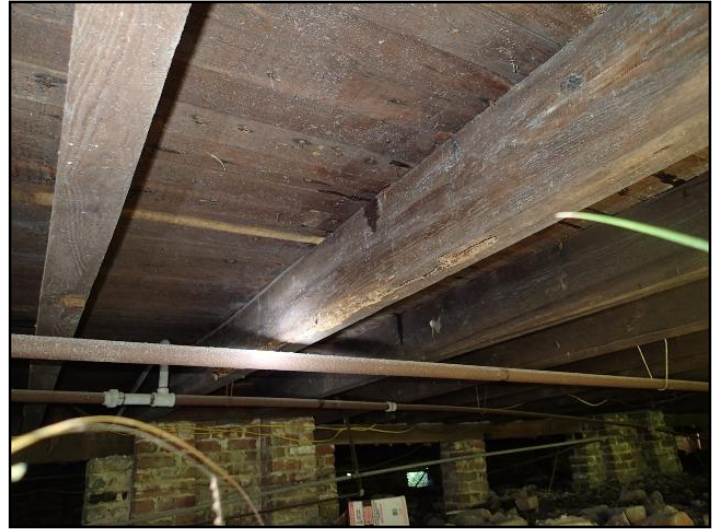
34. Rot, insect or fire damage
