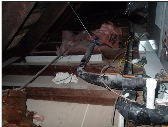
57. No flooring for servicing unit
