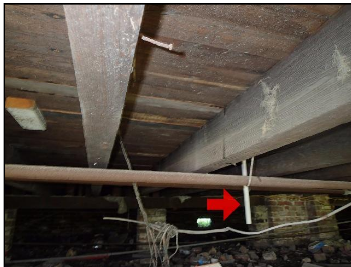
65. Improper discharge point
