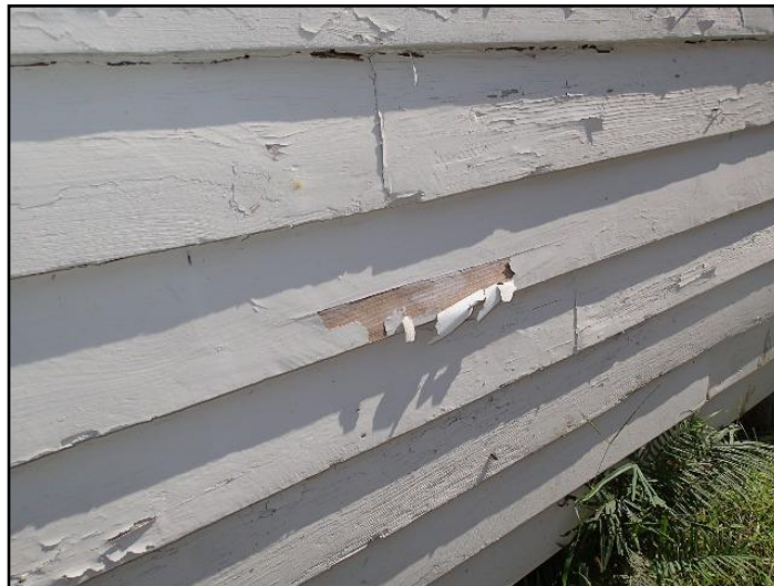
11. Peeling paint on exterior wood surfaces....
