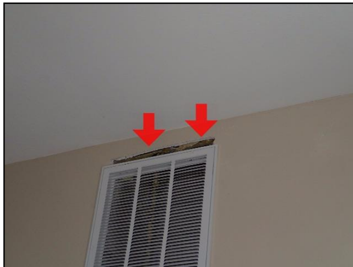
80. Poor joints
