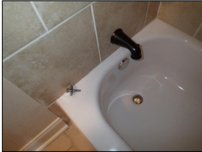
78. Drain stop missing
