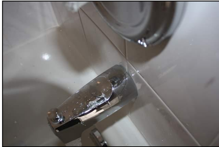
6. Caulking loose, missing or deteriorated
