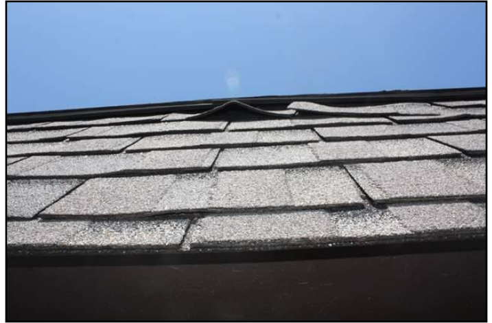
2. Loose, missing or torn tabs
