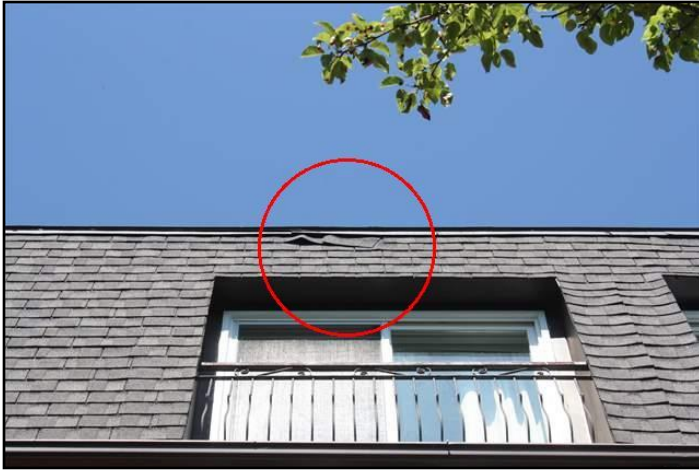
1. Loose, missing or torn tabs
