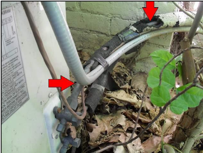
Insulation - missing
