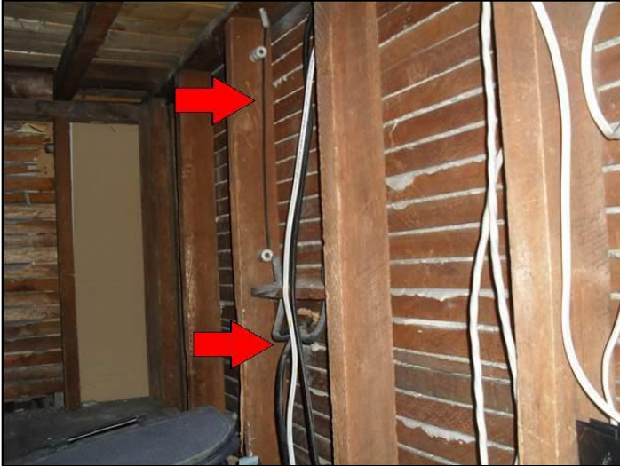
Copper - knob and tube
