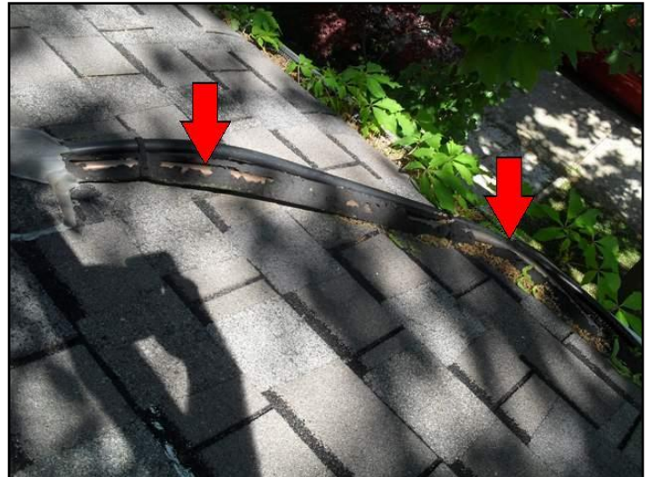
Insulation - missing
