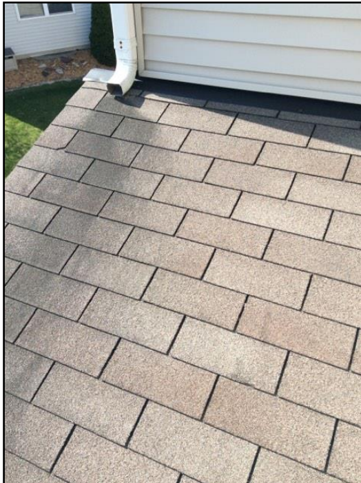
1. Downspouts discharging onto roofs
