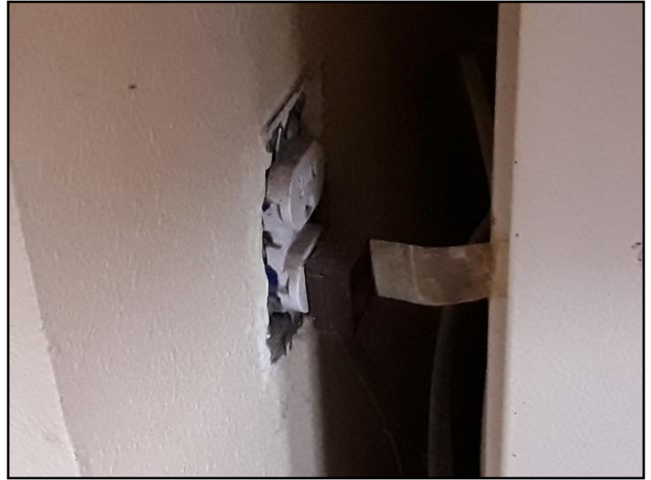
Missing cover - Refrigerator
