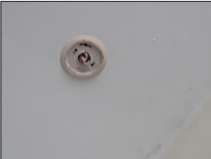
Damaged smoke detectors - Garage
