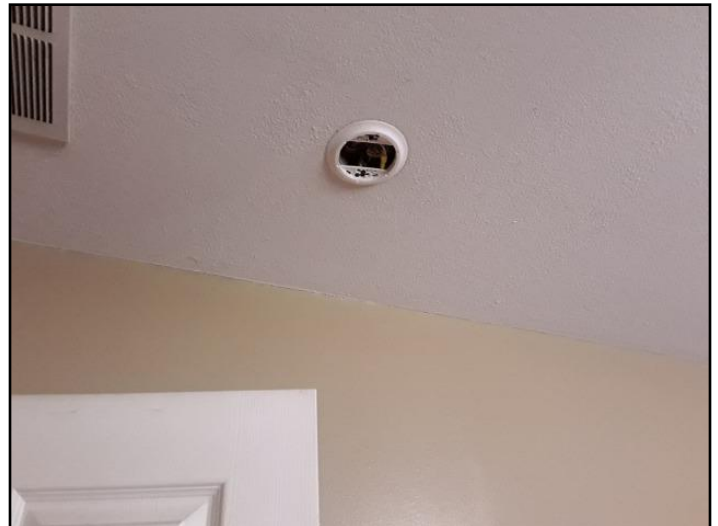
Damaged smoke detectors - Bedroom
