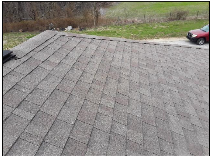
Asphalt composition shingles
