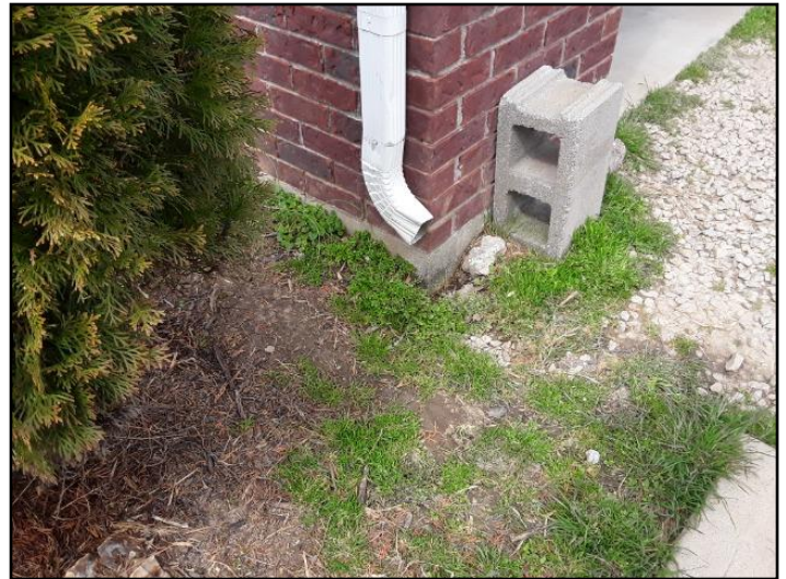
Missing splash block
