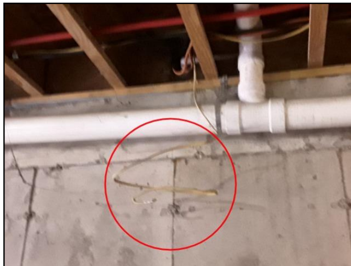
Exposed "Hot" wires
