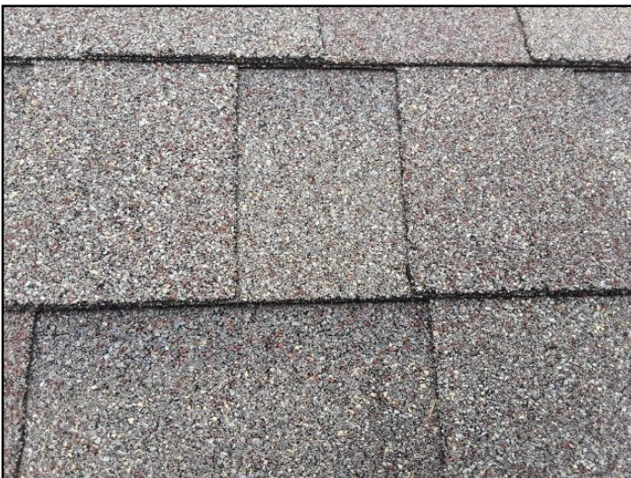
Asphalt composition shingles
