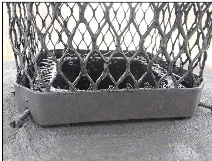
Creosote build-up (front flue)
