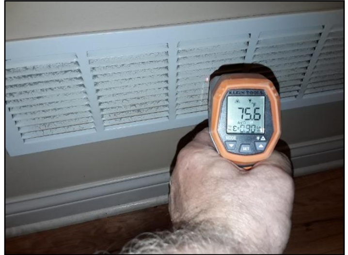
Cooling return temp 76 deg
