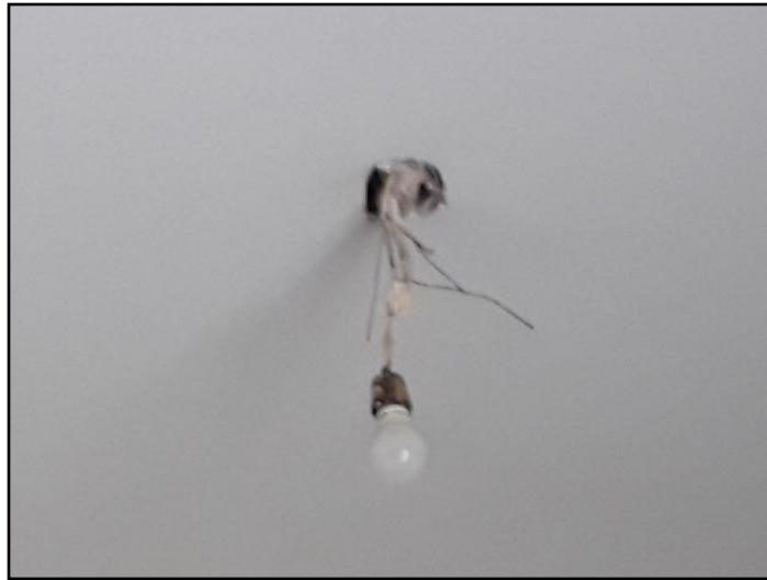
Damage light fixture
