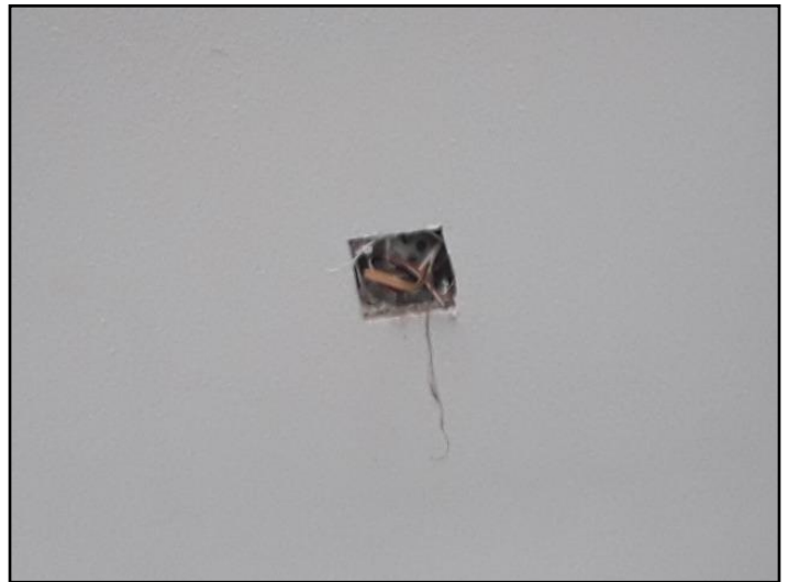
Missing cover - Garage ceiling
