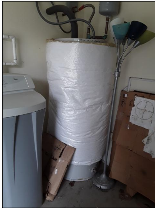
Electric water heater
