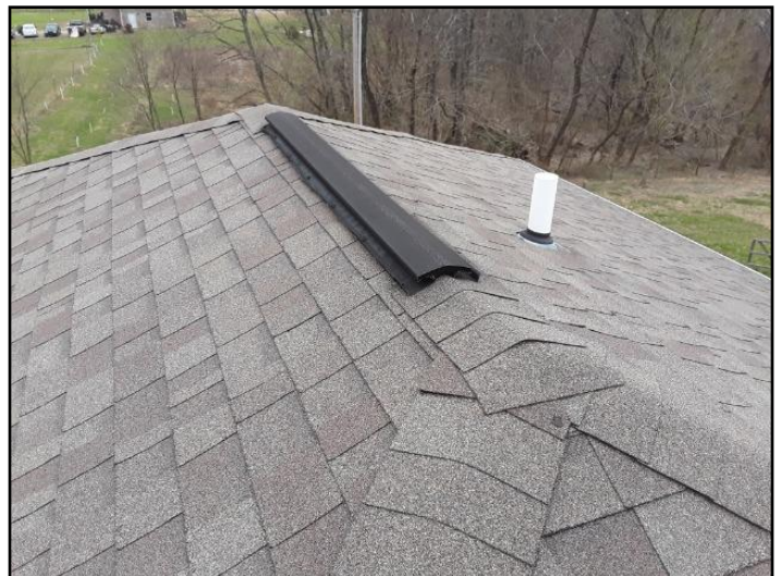
Asphalt composition shingles
