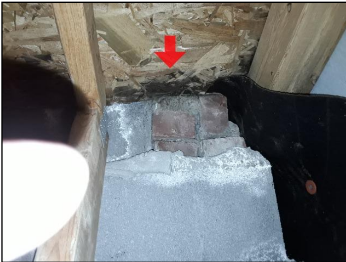
Signs of past leak (viewed from attic)
