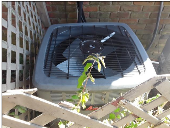
Air flow around A/C was restricted
