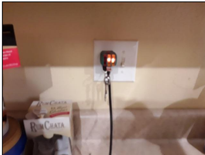
GFCI Outlet recommended
