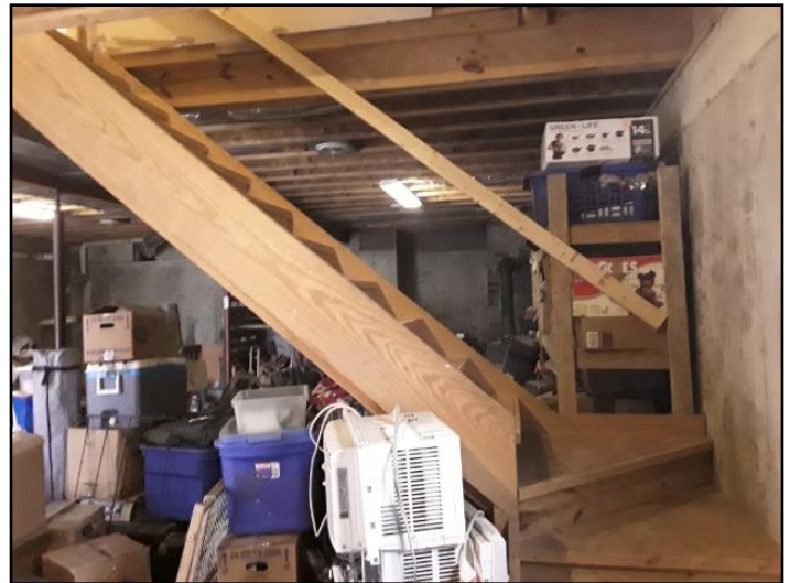
Sub-standard handrails
