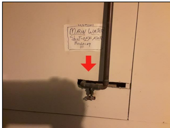
Main water shut-off valve
