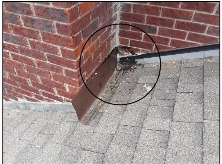
Evidence of trapped water
