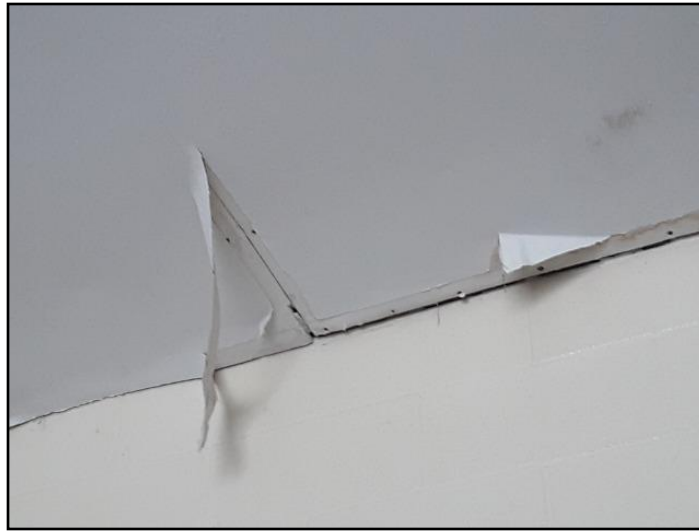
Ceiling drywall damage
