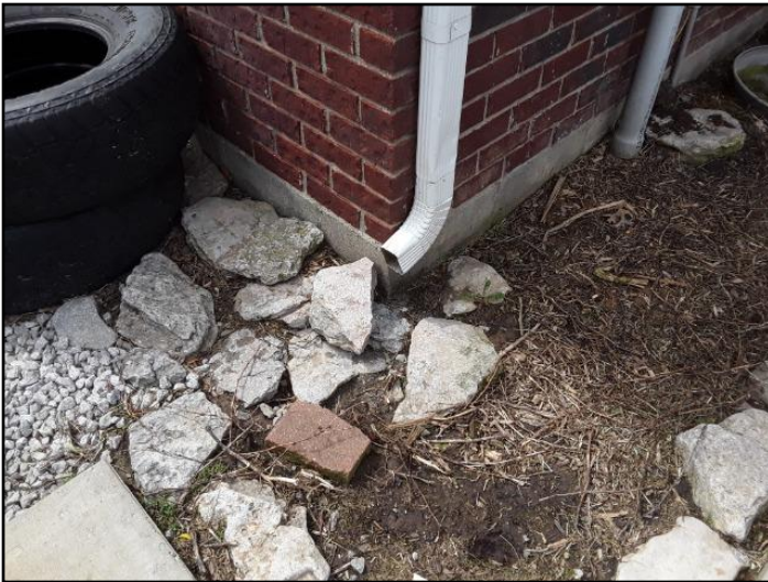
Missing splash block
