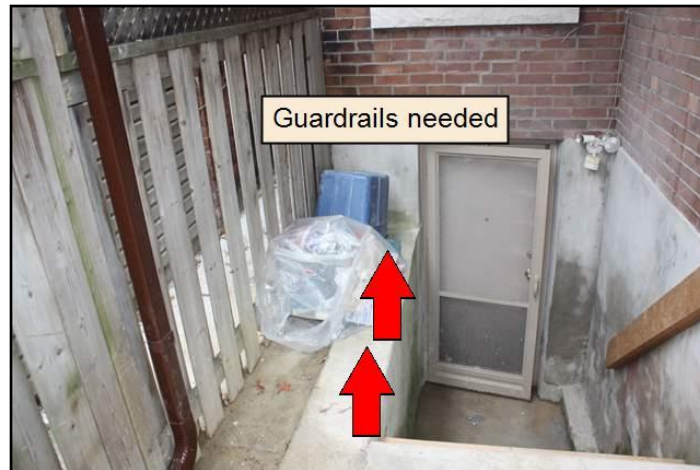
17. Guard and handrail problems
