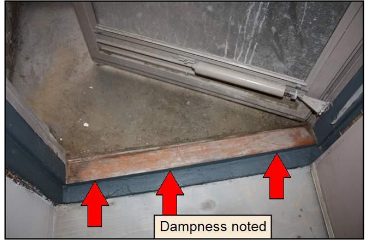
19. Door threshold missing, too low, not...
