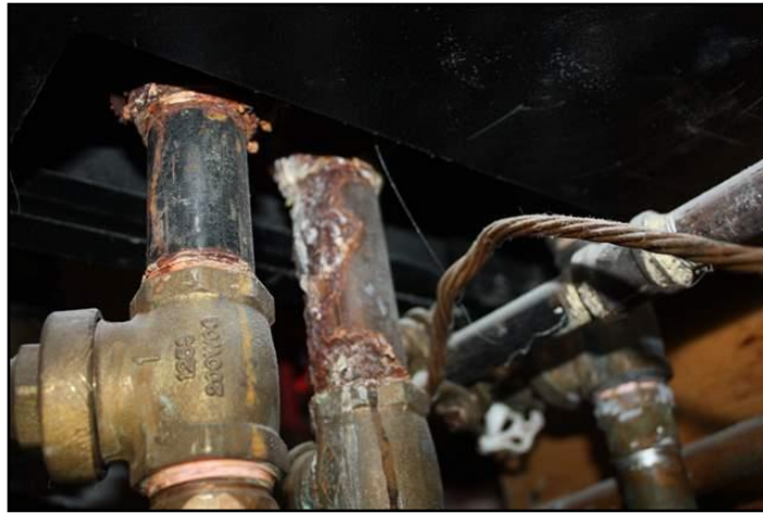
32. Rust / Corrosion
