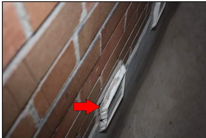
7. Caulking missing or ineffective
