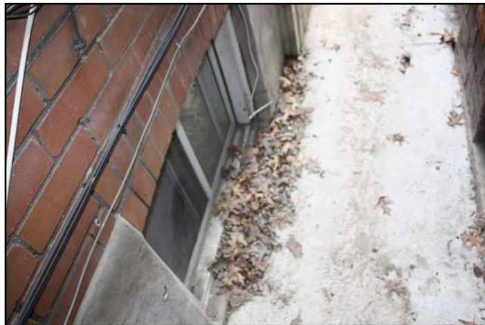
9. Sill - Near or at Grade Level
