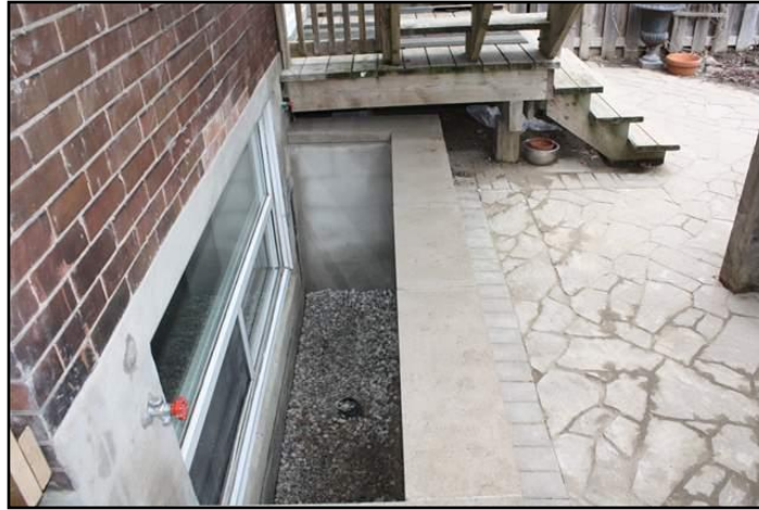
14. Missing Guardrail around window well
