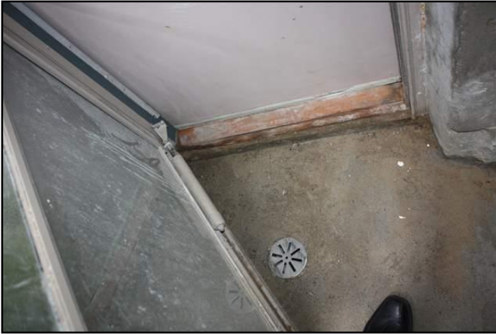
18. Door threshold missing, too low, not...
