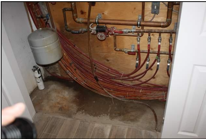
42. Dampness on floor or walls
