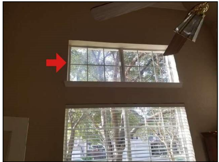
20. Lost seal on double or triple glazing
