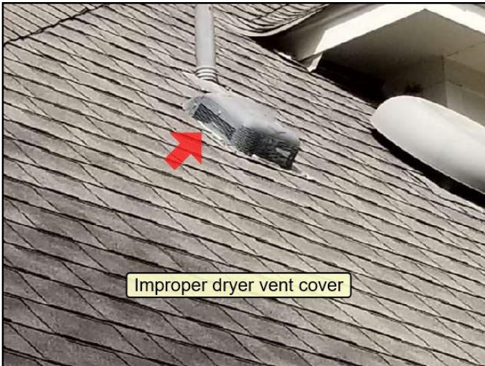
24. Improper roof top dryer vent discharge and...
