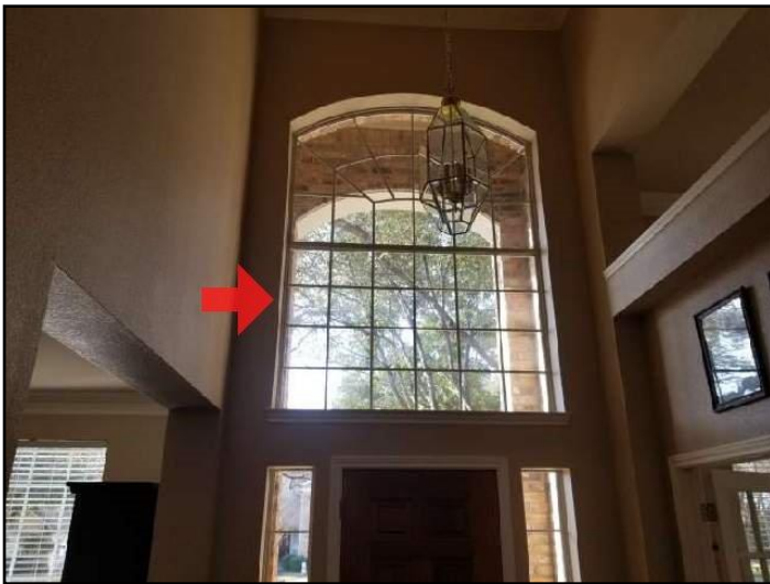
19. Lost seal on double or triple glazing
