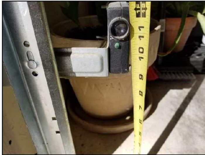
22. Sensors poorly located
