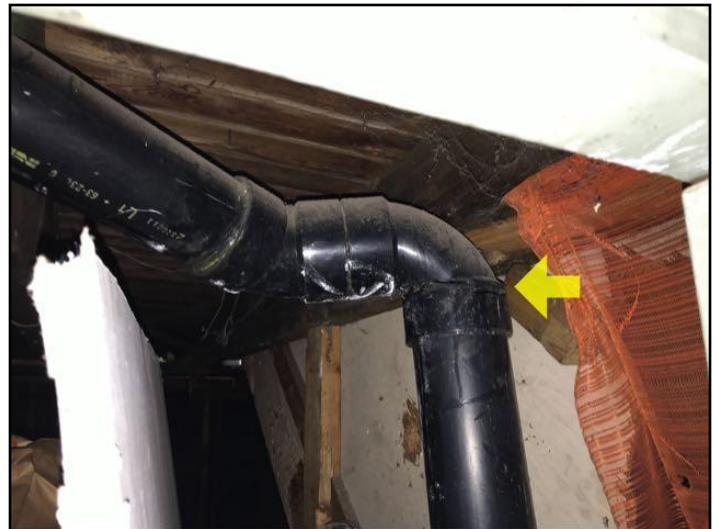
Damage, leak
