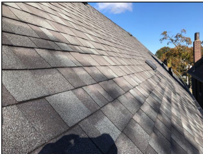
Asphalt shingles
