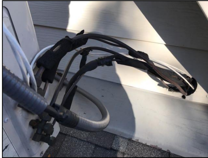
Insulation - incomplete/missing
