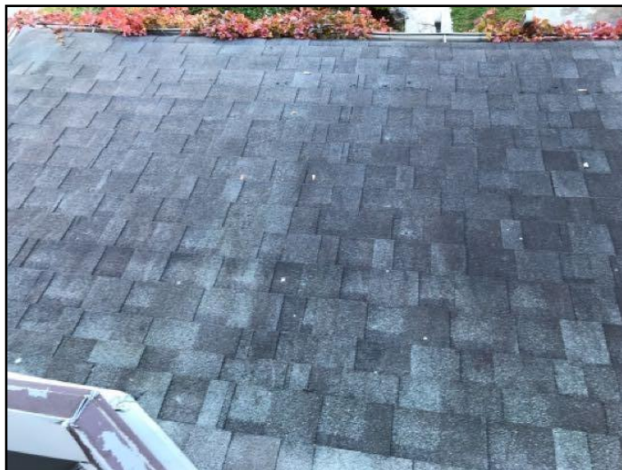
Asphalt shingles
