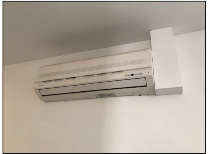
Ductless (Mini split) system
