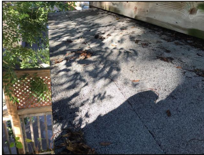
Modified bitumen membrane
