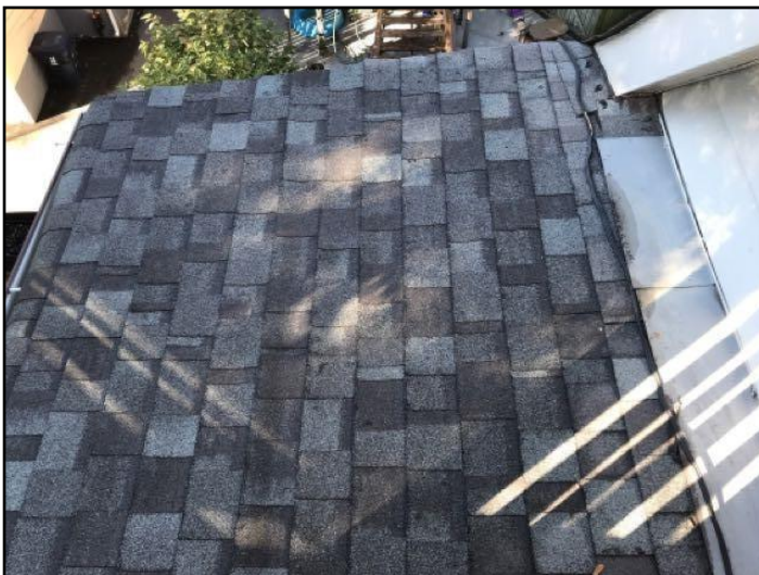
Asphalt shingles
