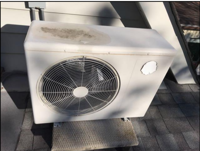
Ductless (Mini split) system
