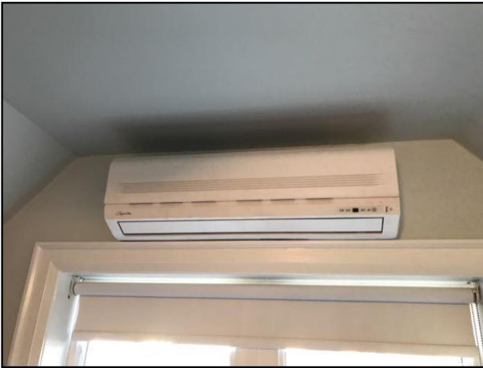
Ductless (Mini split) system
