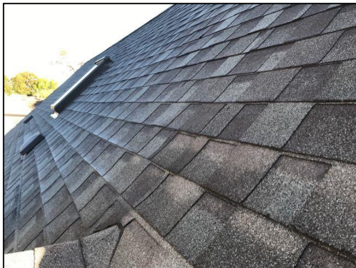
Asphalt shingles
