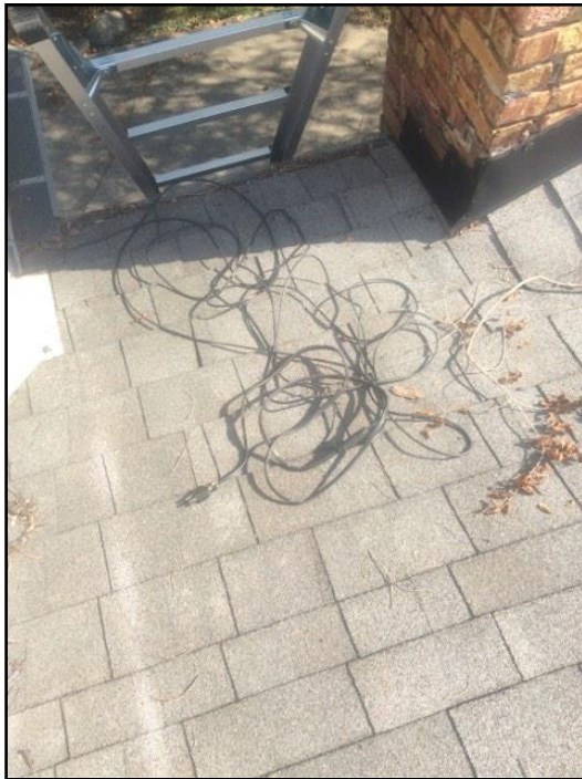
1. Heat tape indicates ice damming issues
