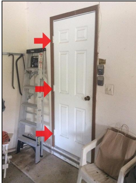
15. Installed backwards
