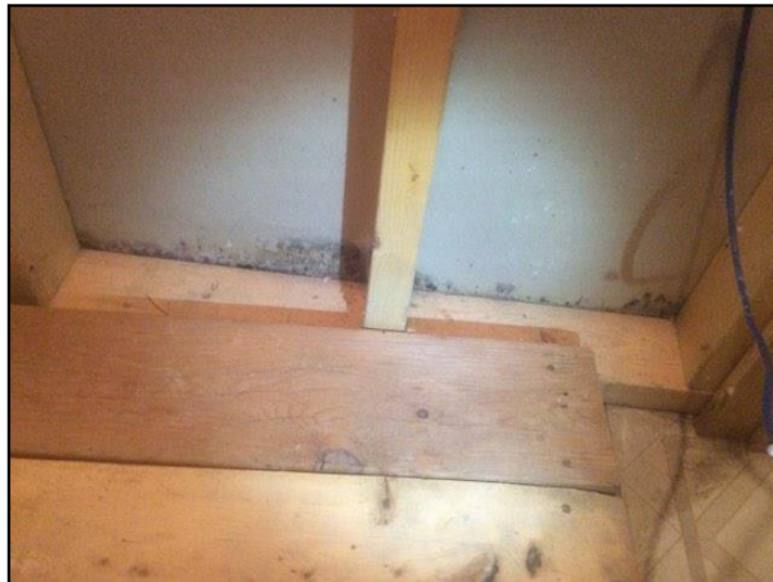
58. Mold in sump closet
