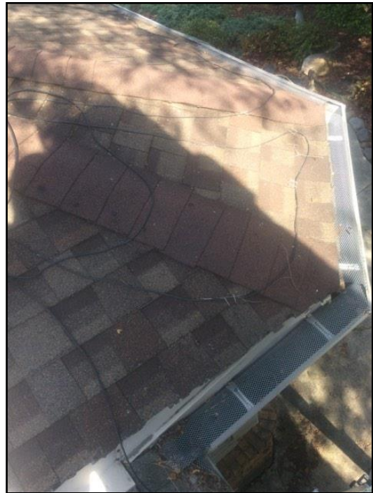
2. Heat tape indicates ice damming issues
