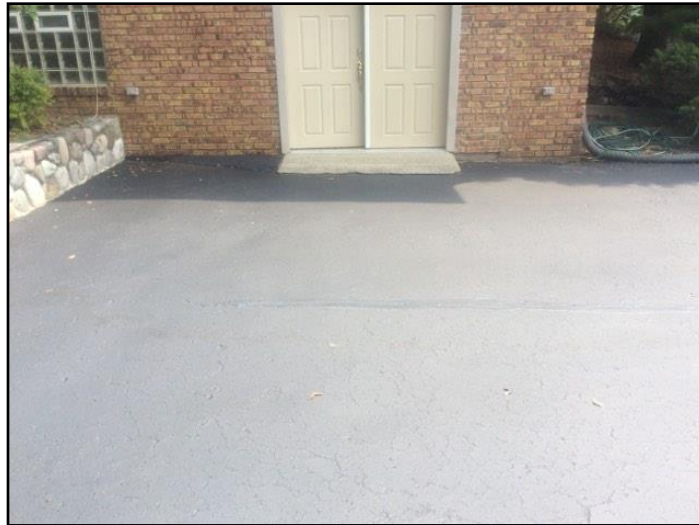
18. Improper slope or drainage
