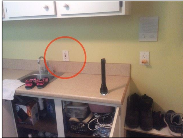
35. Test faulty on Ground Fault Circuit...
