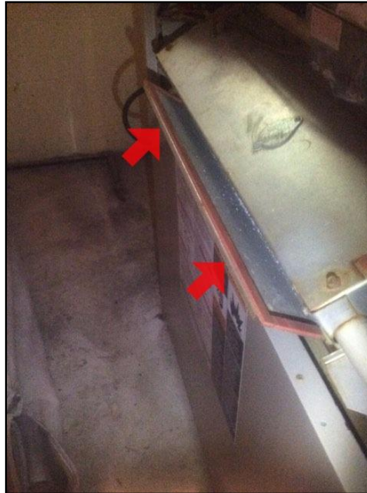
40. Vent damper stuck
