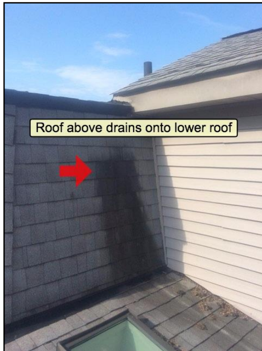
4. Poor drainage arrangement
