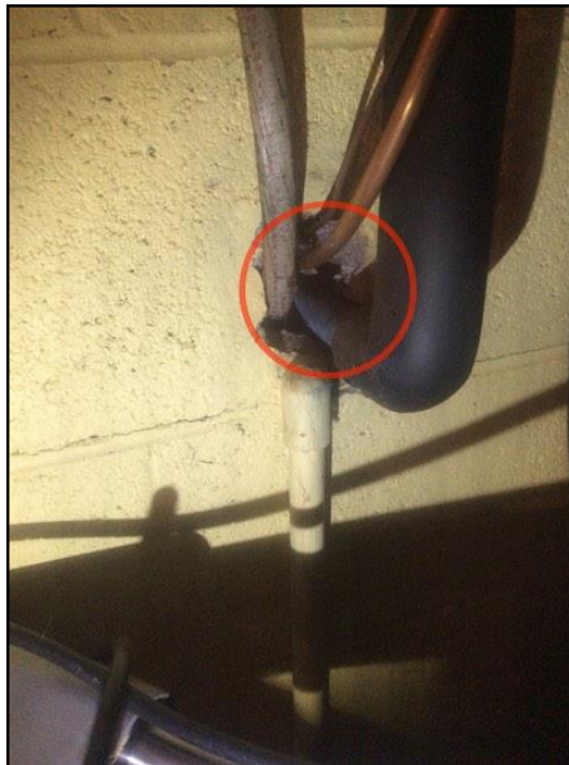
43. Poor seal at building
