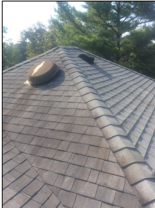
46. Cannot mix different types of exhaust vents
