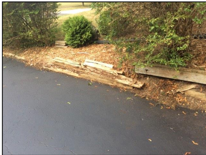
20. Rot or insect damage
