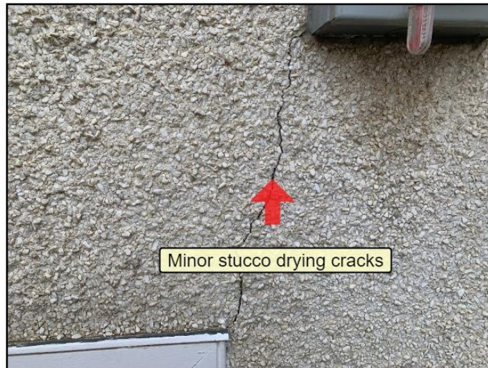
10. Minor stucco drying cracks
