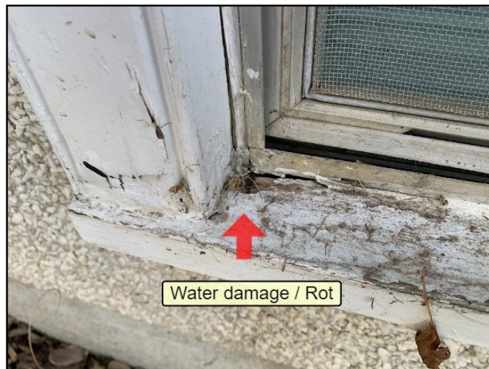
11. Water damage / Rot
