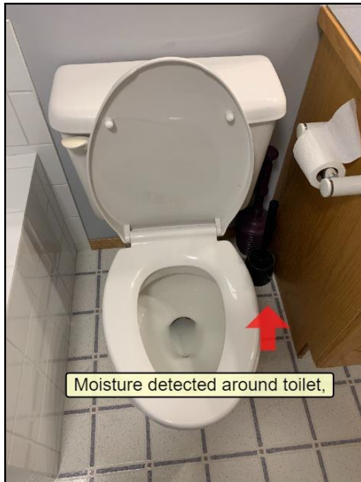
57. Moisture detected around toilet,
