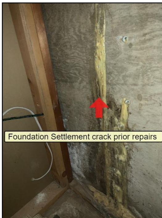
16. Foundation Settlement crack prior repairs
