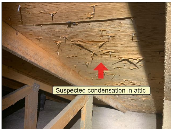
47. Suspected condensation in attic
