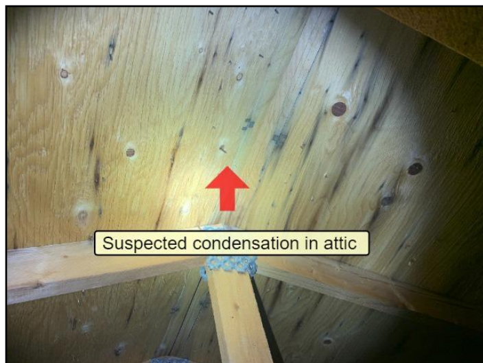
48. Suspected condensation in attic
