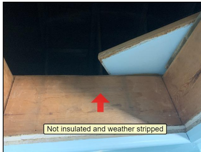
46. Not insulated and weather stripped
