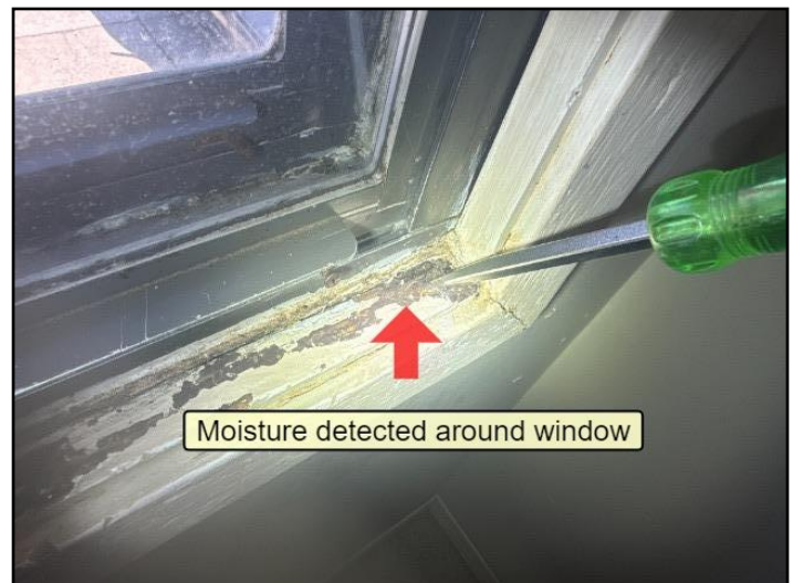
64. Moisture detected around window
