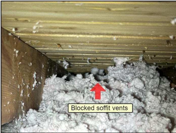
59. Blocked soffit vents
