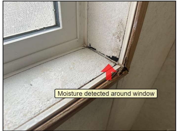
66. Moisture detected around window
