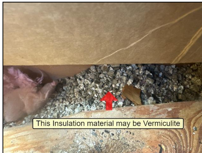
43. This Insulation material may be Vermiculite
