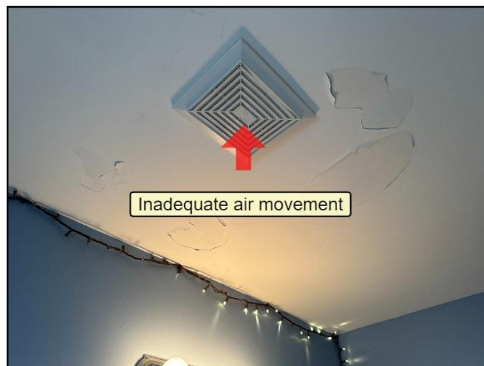
68. Inadequate air movement
