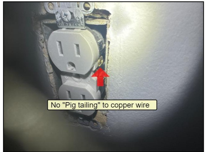
23. No "Pig tailing" to copper wire
