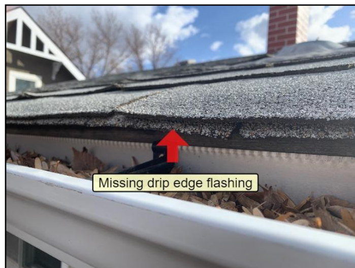
7. Missing drip edge flashing
