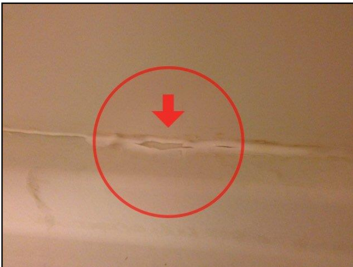
Caulking loose, missing or deteriorated
