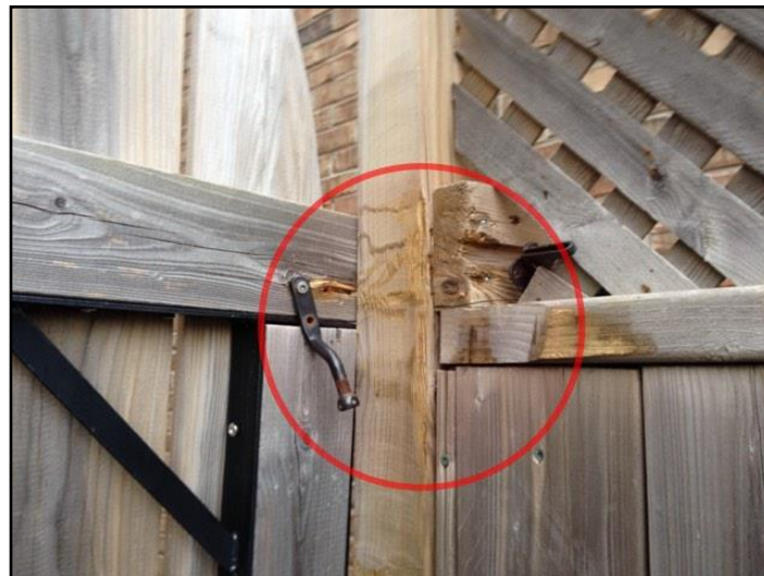
Gate latch - adjustment needed
