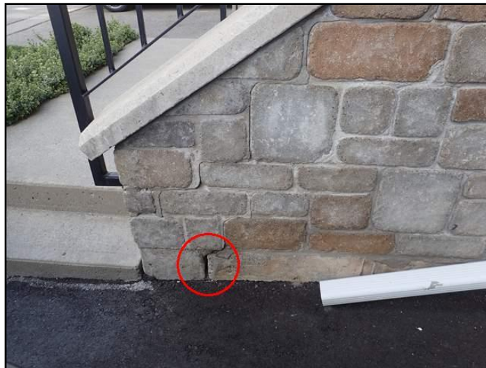
Improve mortar at front steps
