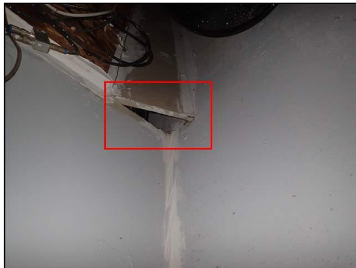
Seal any gaps between garage and house
