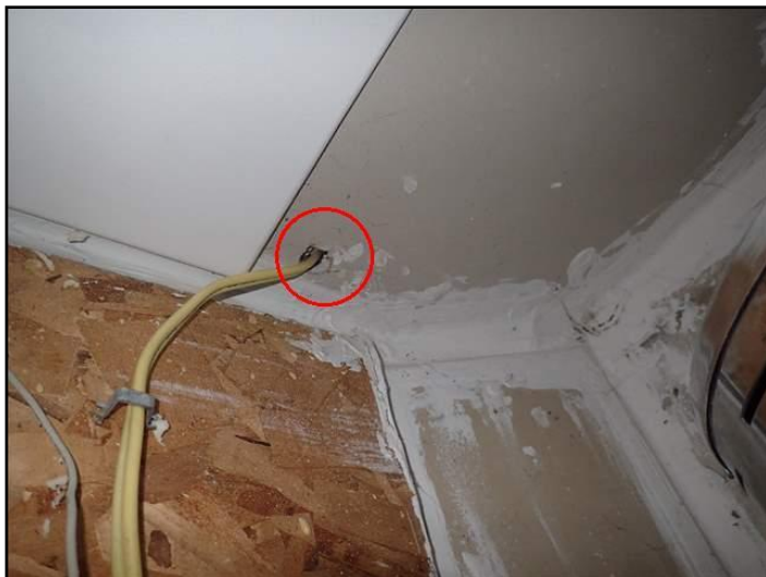
Seal any gaps between garage and house
