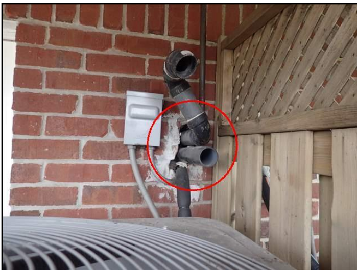
Poor seal at exterior wall
