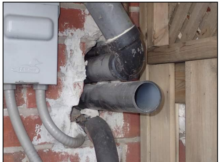
Poor seal at exterior wall
