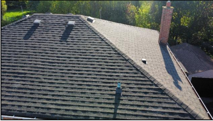
1. Asphalt shingles
