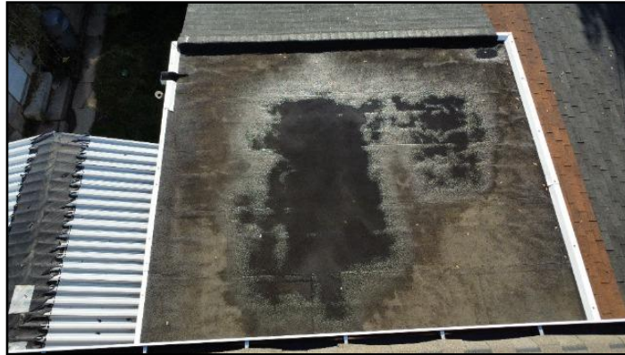
3. Modified bitumen membrane
