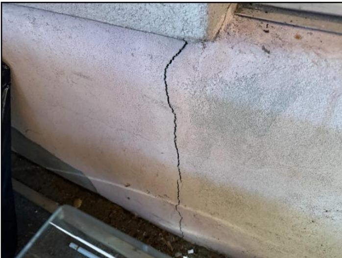
26. Walls cracking
