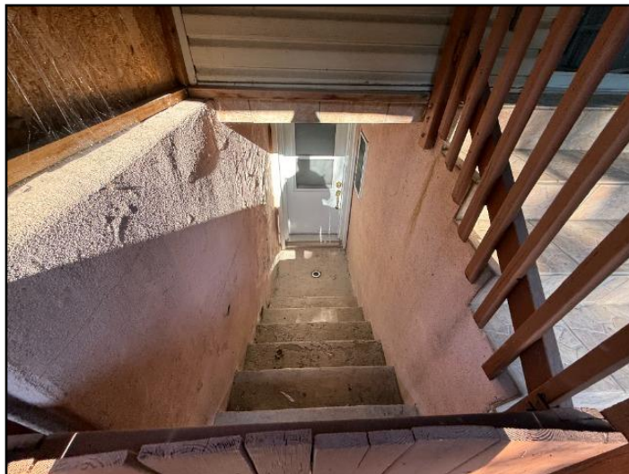
29. Handrail missing
