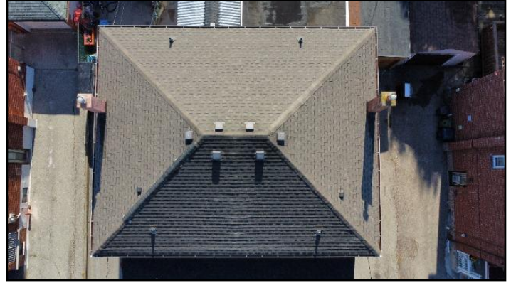
2. Asphalt shingles
