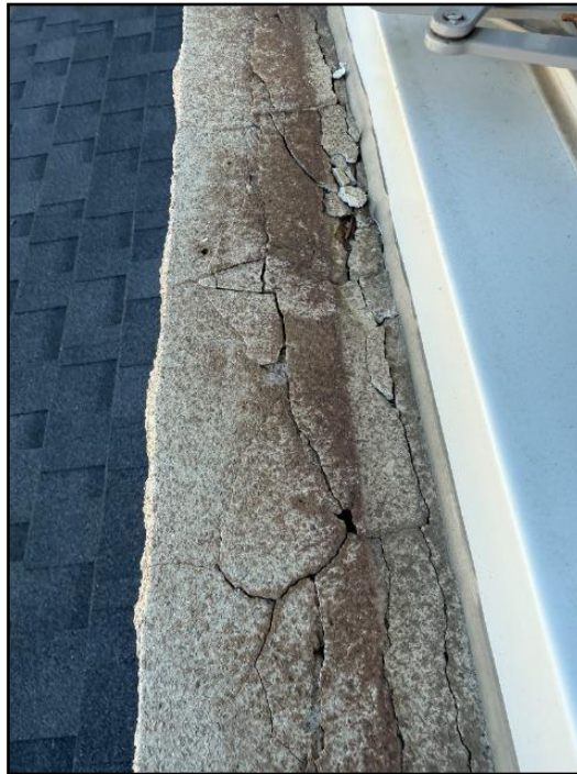
19. Sill deteriorated
