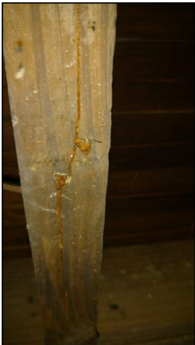
104. Rot, insect or fire damage
