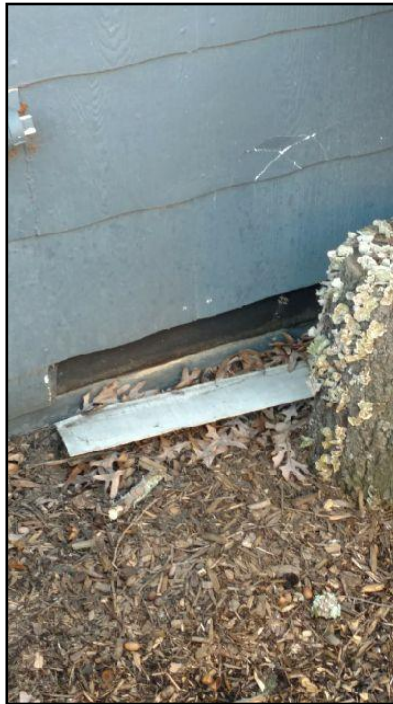
6. Mechanical damage
