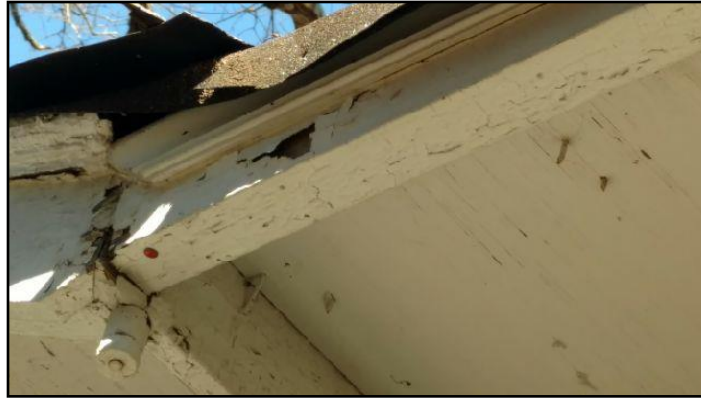
73. Water Damaged
