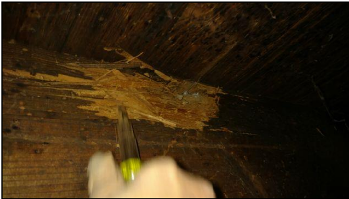
102. Rot, insect or fire damage
