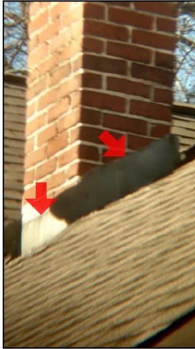
3. Not let into mortar joints
