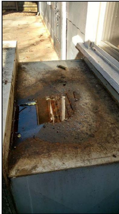
48. Cowling is sagging and retaining water and...
