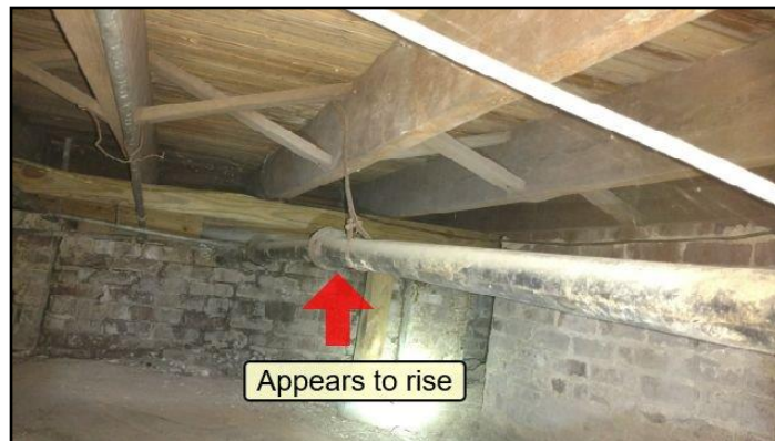
52. Fall on drain line is not sufficient
