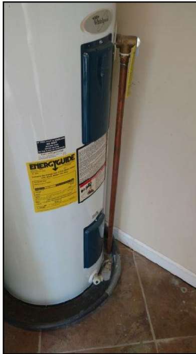
127. TPR Drainline draining in to pan instead of...
