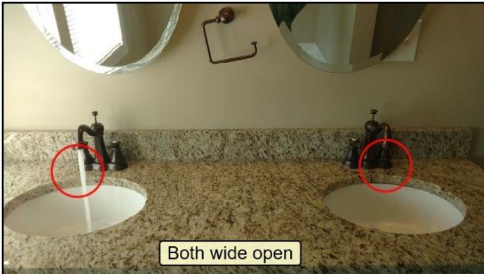
53. Flow lower than balance of home
