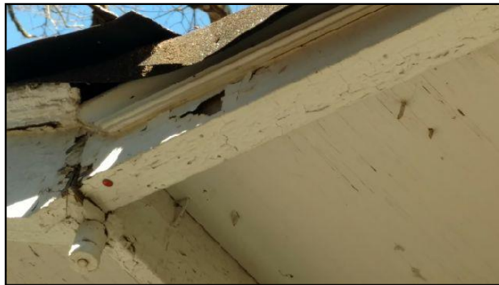
5. Water Damaged
