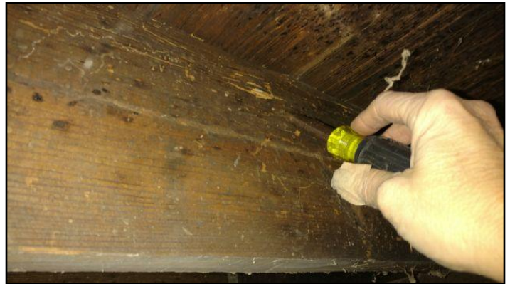
103. Rot, insect or fire damage
