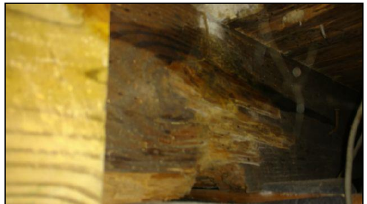
33. Rot, insect or fire damage
