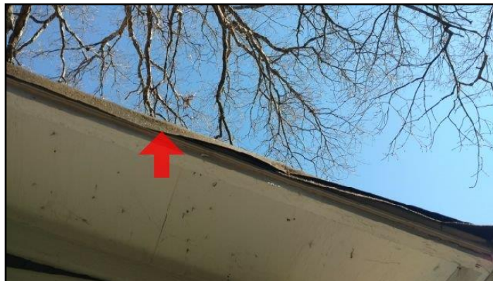
1. Overhangs too big or small Asphalt roofing...
