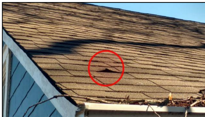
70. Raised fasteners under roofing - When you...
