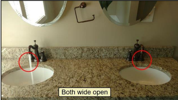
129. Flow lower than balance of home
