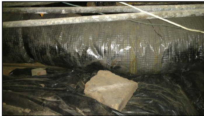
119. Ductwork is laying on the ground. This will...
