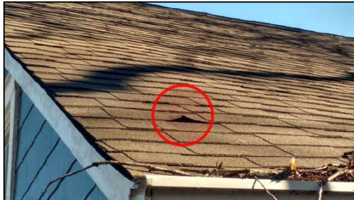
2. Raised fasteners under roofing - When you...
