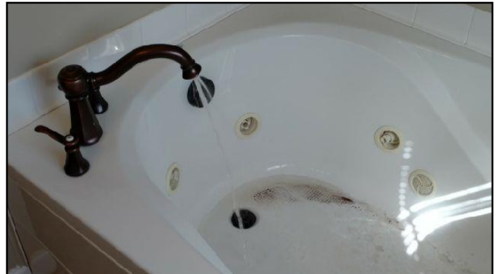
54. Flow lower than balance of home
