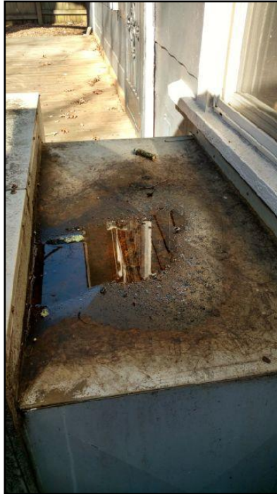
120. Cowling is sagging and retaining water and...
