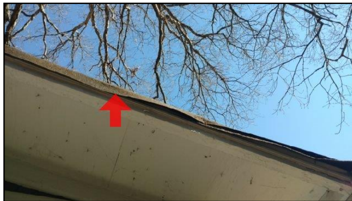
69. Overhangs too big or small Asphalt roofing...
