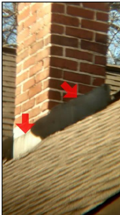
71. Not let into mortar joints
