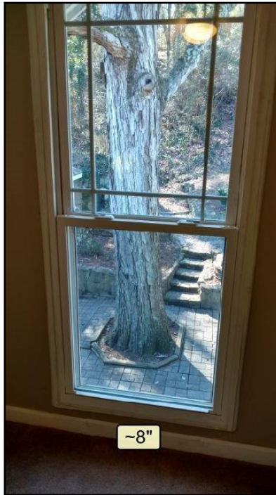
135. Safety glass not installed
