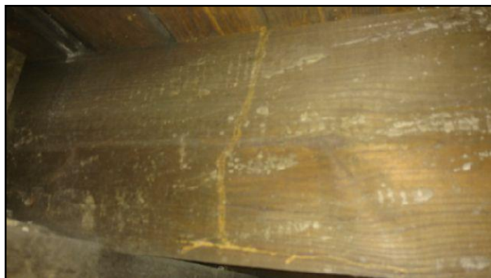
106. Rot, insect or fire damage
