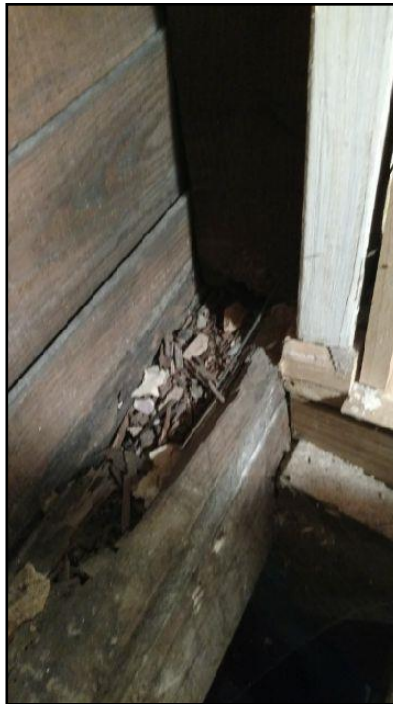
108. Rot, insect or fire damage
