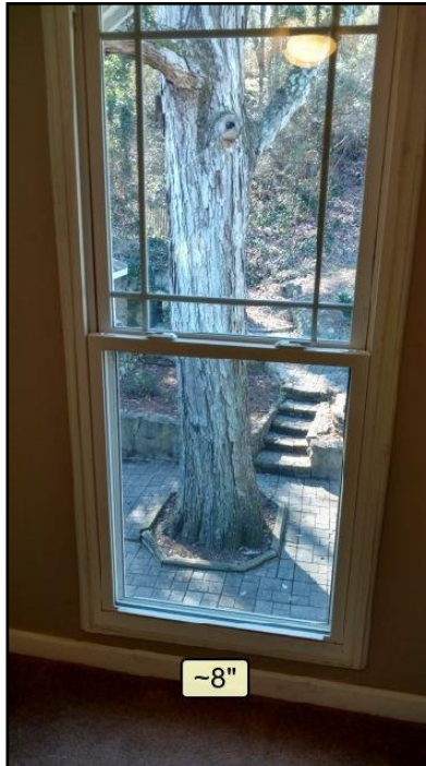
59. Safety glass not installed
