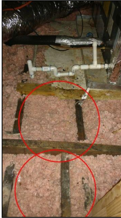
45. Equipment placed in the attic over finished...
