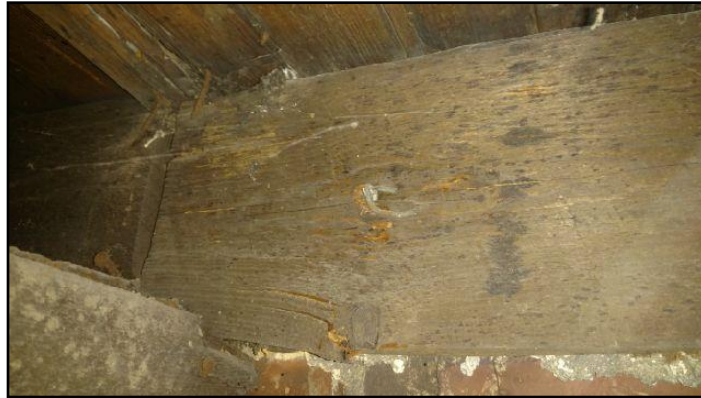
39. Rot, insect or fire damage
