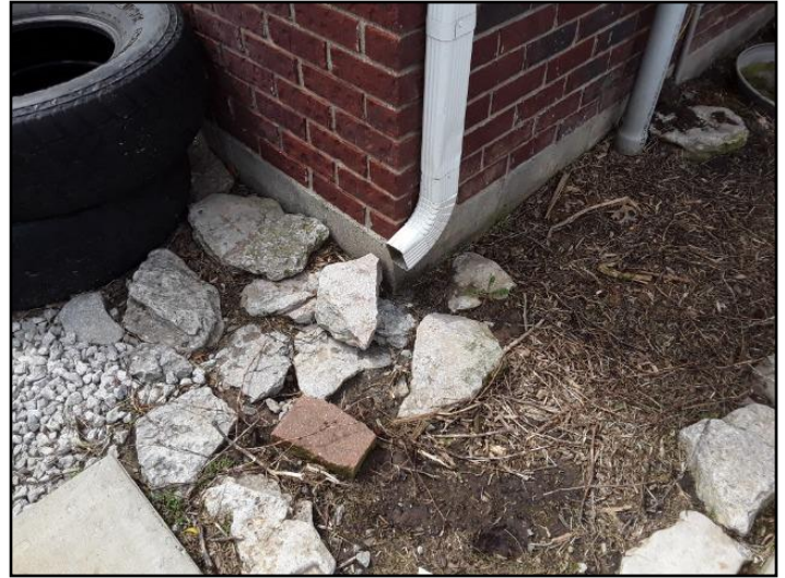
8. Missing splash block
