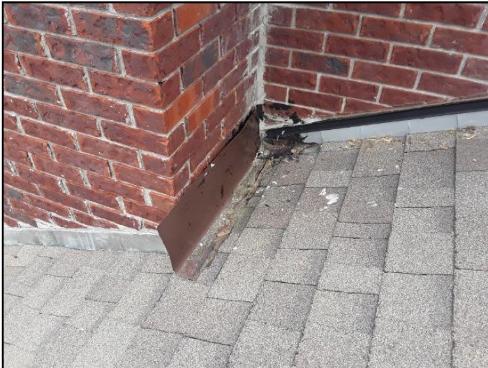
5. Evidence of trapped water
