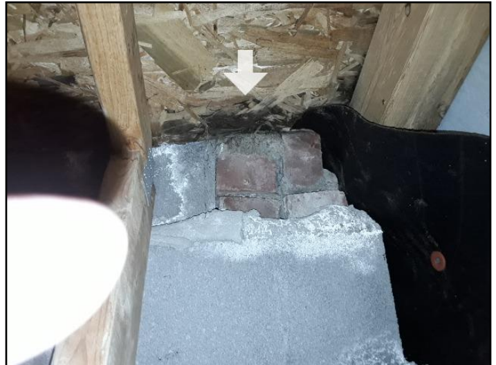
6. Signs of past leak (view from attic)
