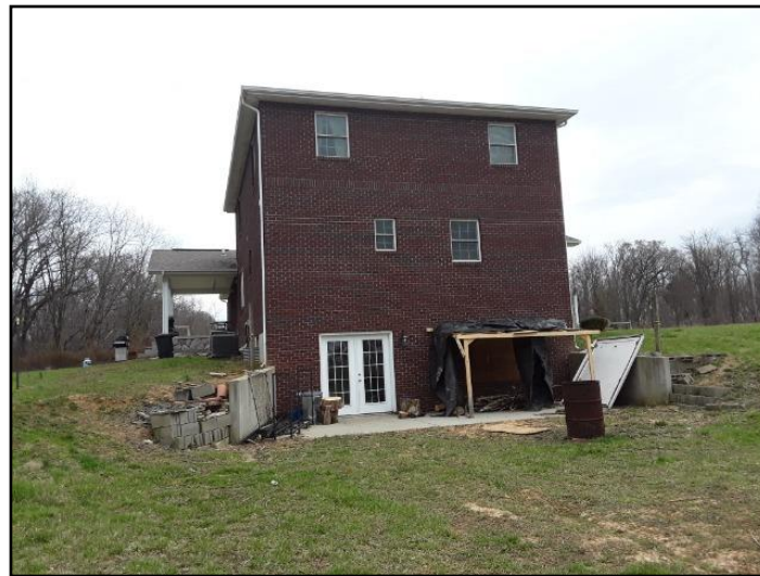
11. Improper slope - swale needed
