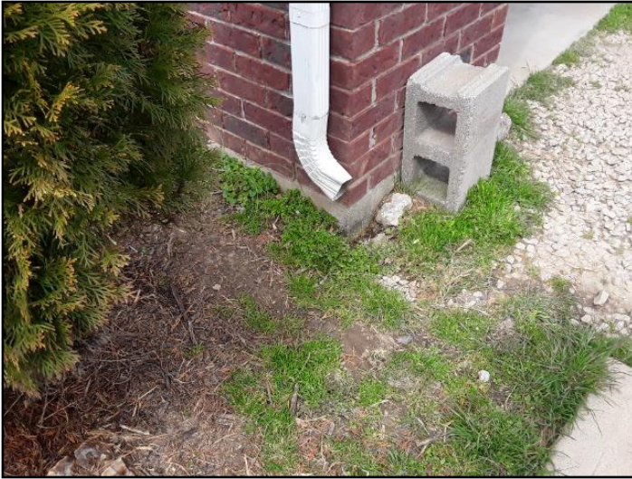
7. Missing splash block
