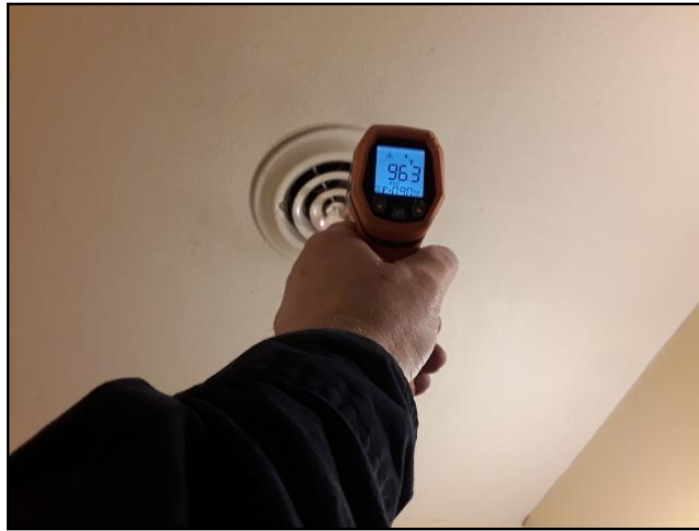
26. Heater supply temp 96 deg
