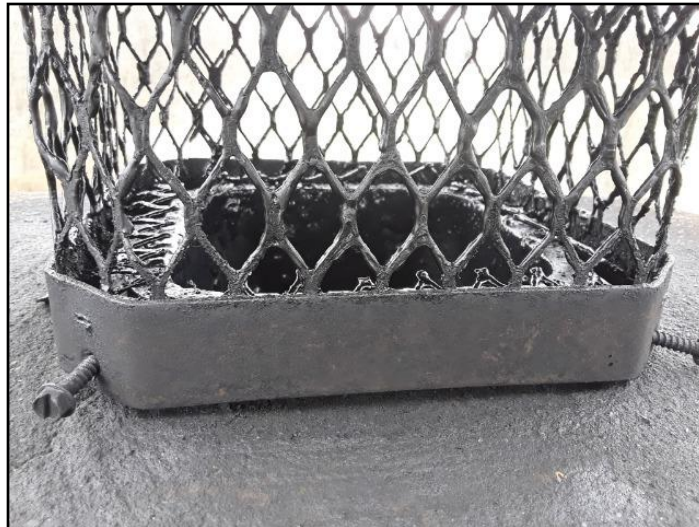
30. Creosote build-up (front flue)
