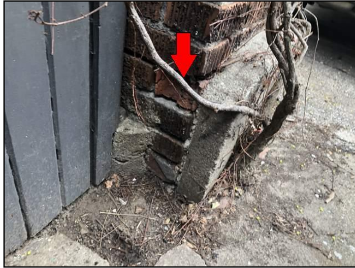
8. Minor spalling
