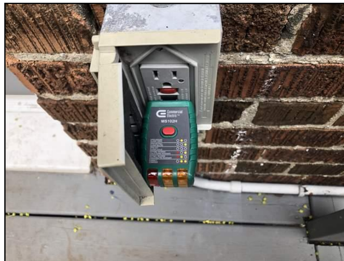
16. Test faulty on GFCI/GFI (Ground Fault...
