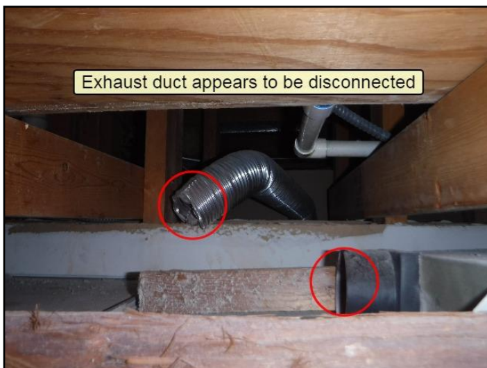
58. Discharging into the attic / ceiling space
