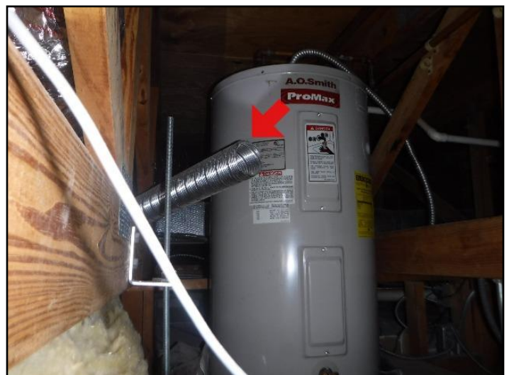
6. Discharging into the attic / ceiling space
