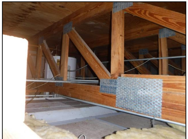
126. Supported by wood roof joists
