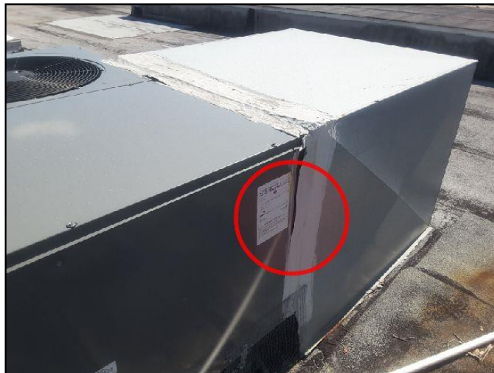
55. Exterior ductwork poor / damaged
