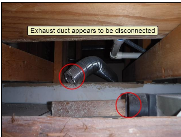
5. Discharging into the attic / ceiling space
