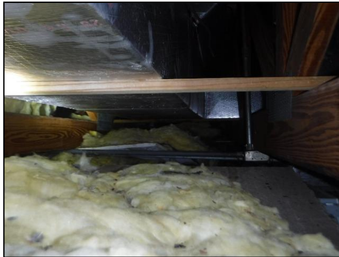
122. Fiberglass insulation
