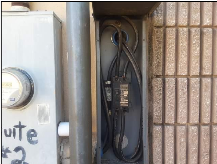
37. Circuit breakers
