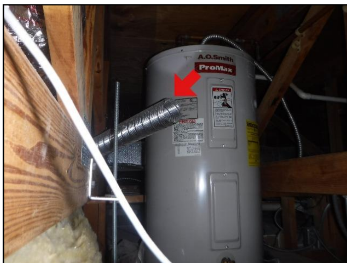
59. Discharging into the attic / ceiling space
