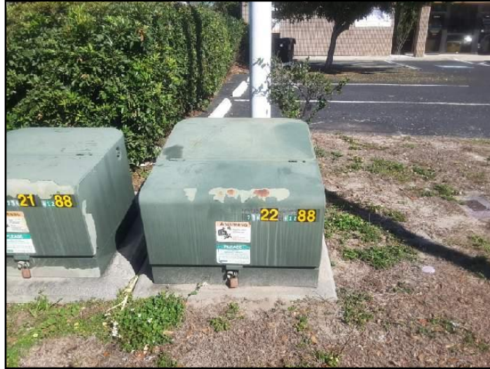
34. Pad-mounted transformer
