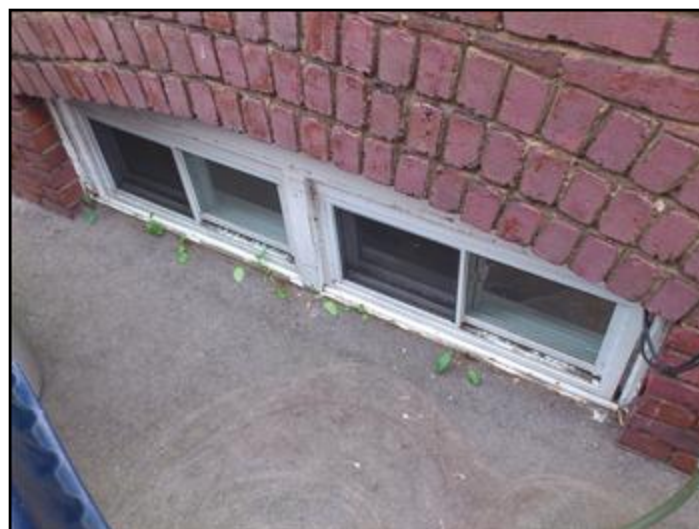
Window well - desirable
