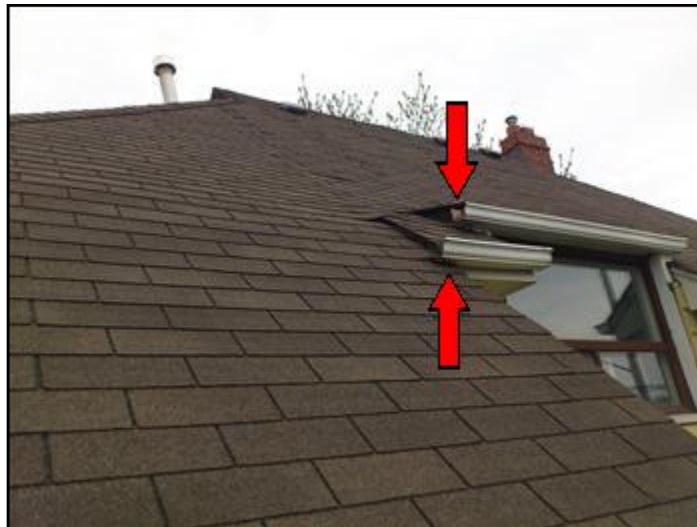
Ex: Upper roof draining onto lower roof
