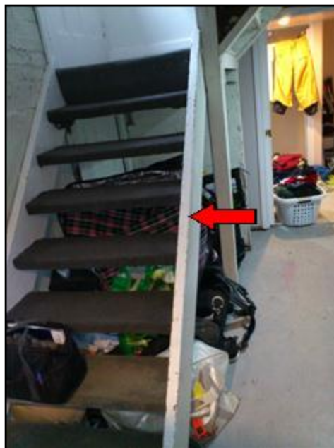
Railing missing
