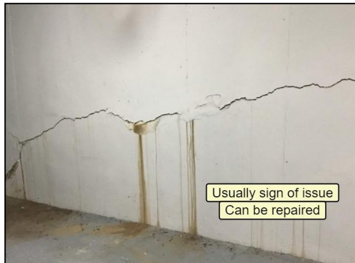
14. Horizontal crack
