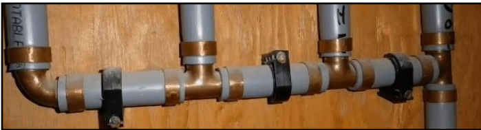
19. Poly B Piping- copper fittings
