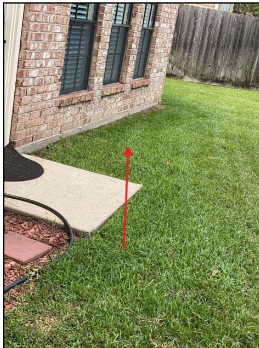
26. Improper slope or drainage
