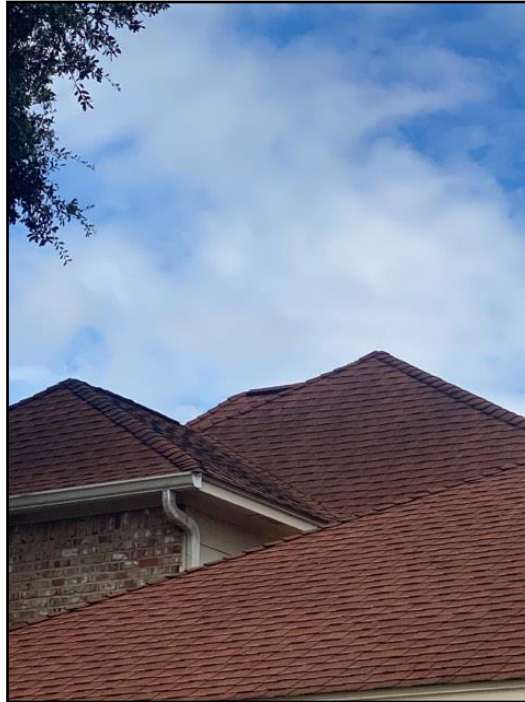
7. Asphalt shingles
