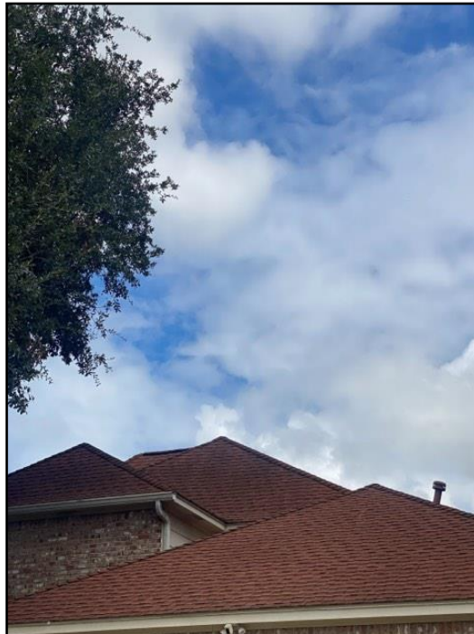
6. Asphalt shingles
