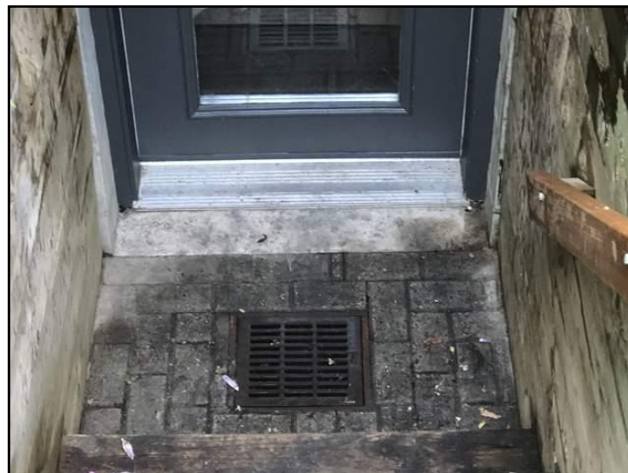
6. Door threshold missing, too low, not...
