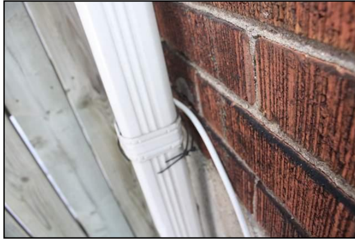
3. not secured to wall
