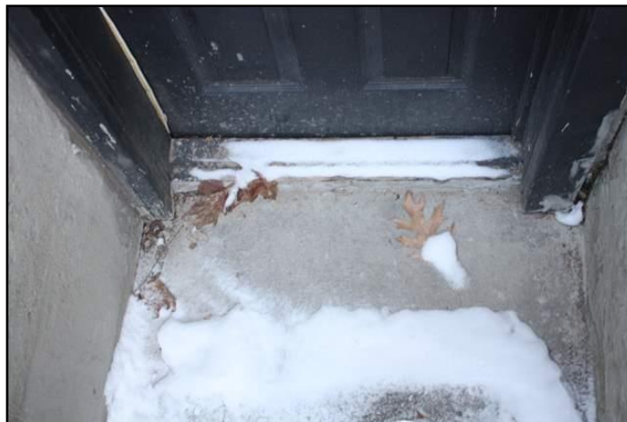
8. Door threshold missing, too low, not...
