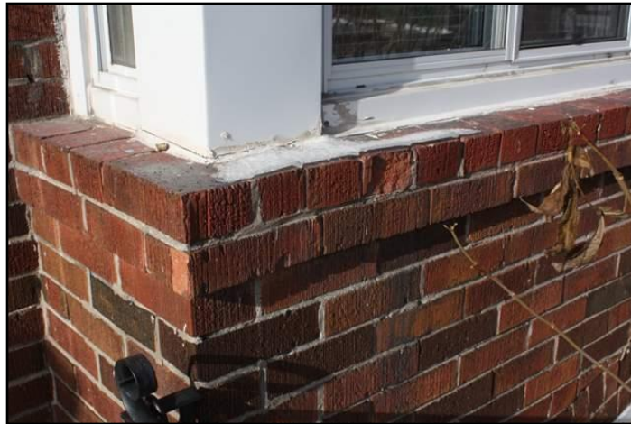
4. Spalling
