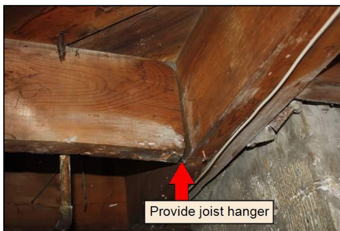
9. joist above boiler
