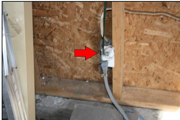
19. For outlet (receptacle) is damaged
