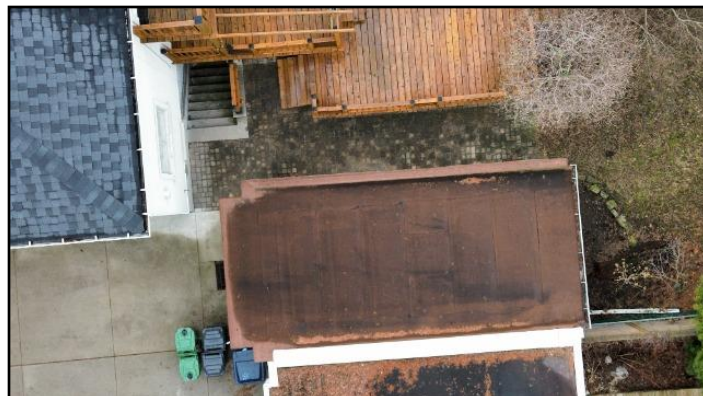
4. Garage Modified bitumen membrane
