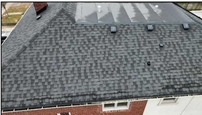
1. Asphalt shingles
