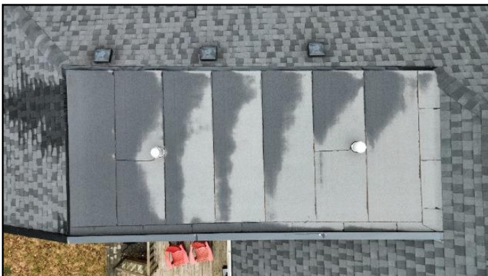
3. House Modified bitumen membrane
