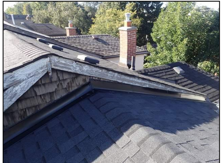
Deteriorated shingle siding
