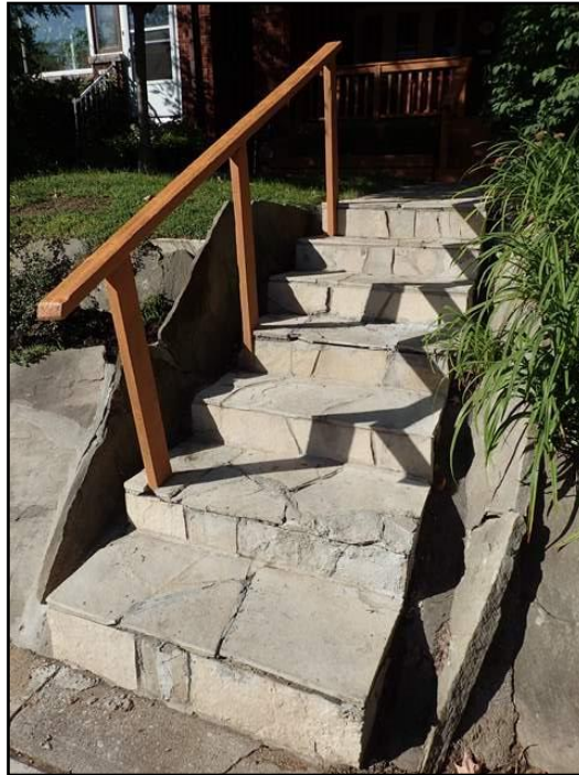
Low quality repairs to stairs
