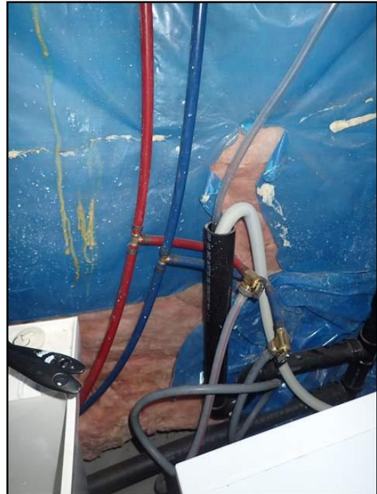
Loose supply and drain piping
