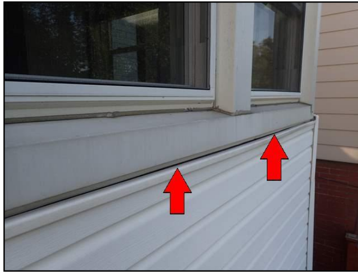
Seal gap between window trim & siding
