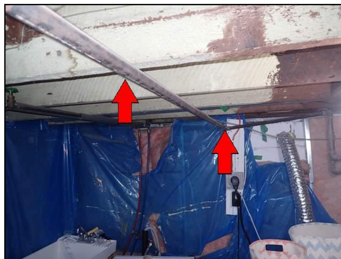
Piping support inadequate
