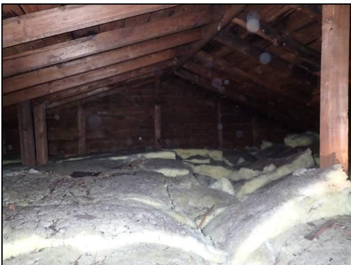
Insulation is relatively even
