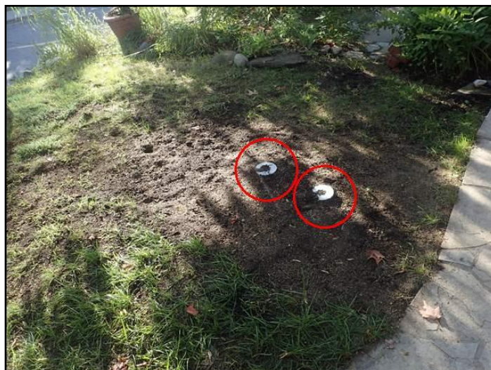
Cleanouts may indicate drain improvements
