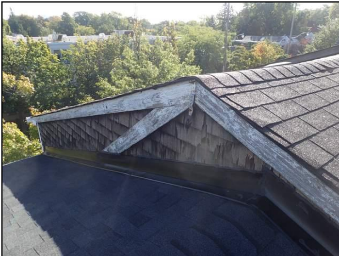
Deteriorated shingle siding
