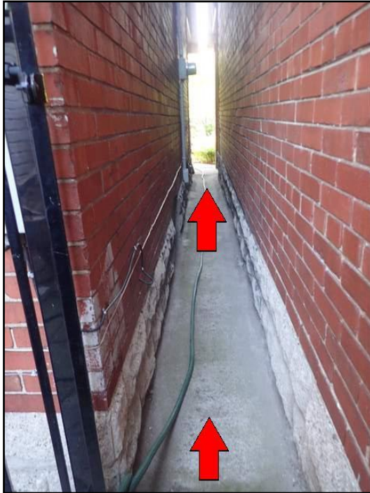
Maintain positive slope away from house
