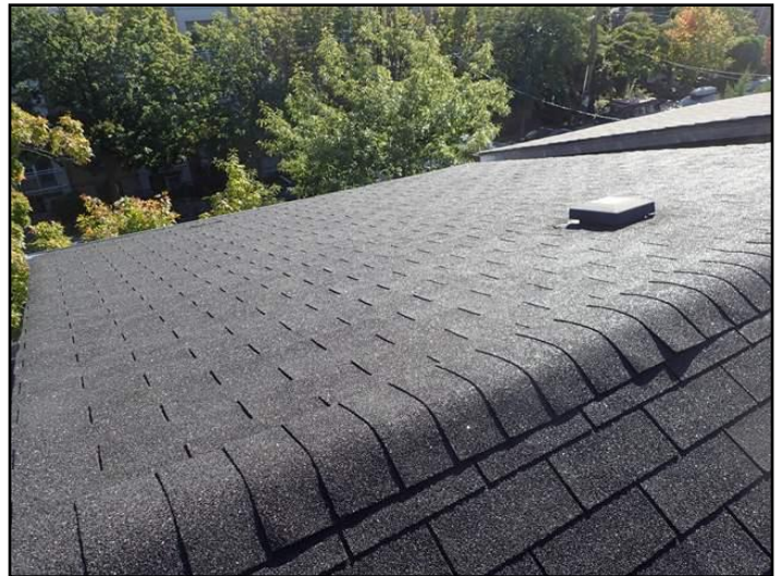
Shingles are in good condition
