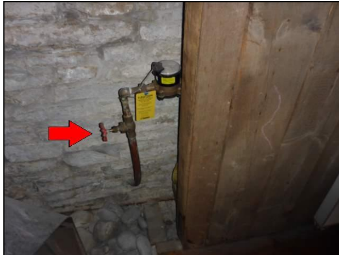
Front of the basement
