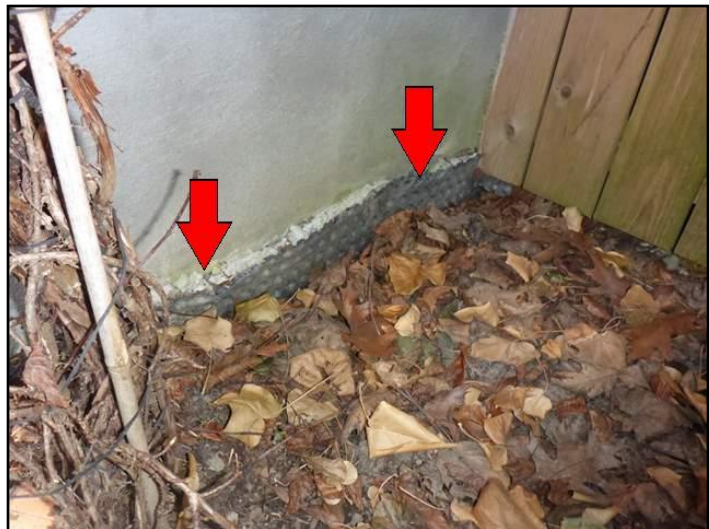
New damp proofing material
