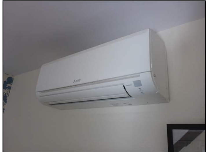
Ductless (Mini split) system- indoor unit
