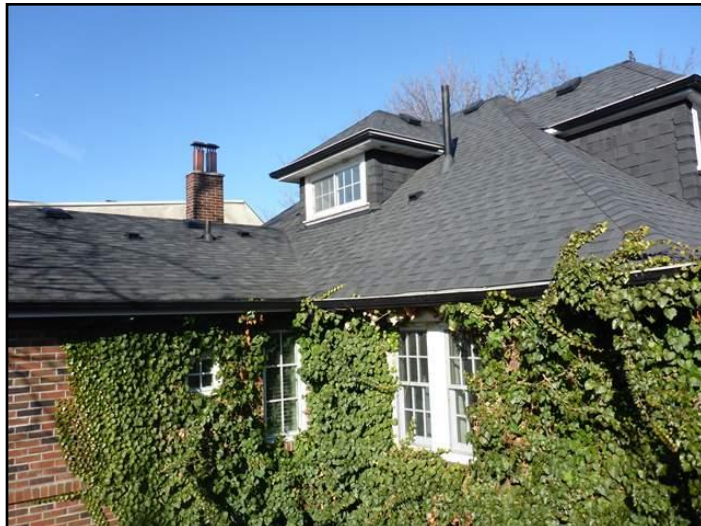
Asphalt shingles
