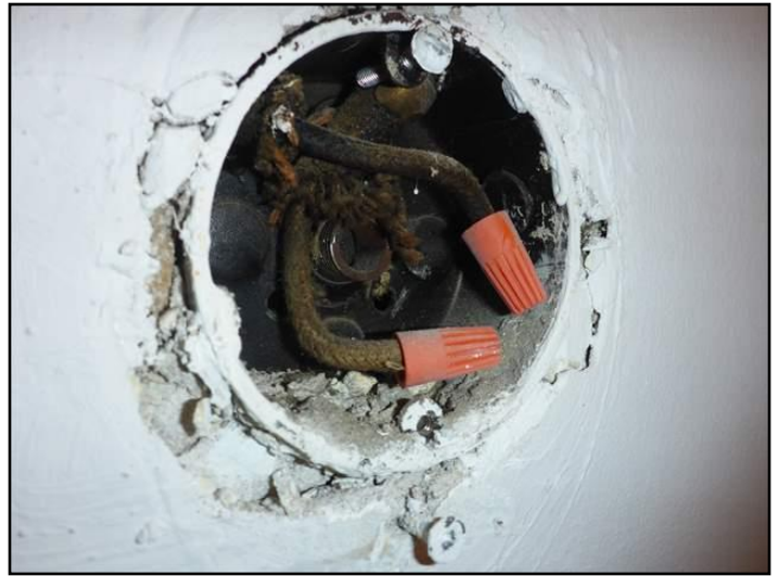
Abandoned, not-energized (third floor)
