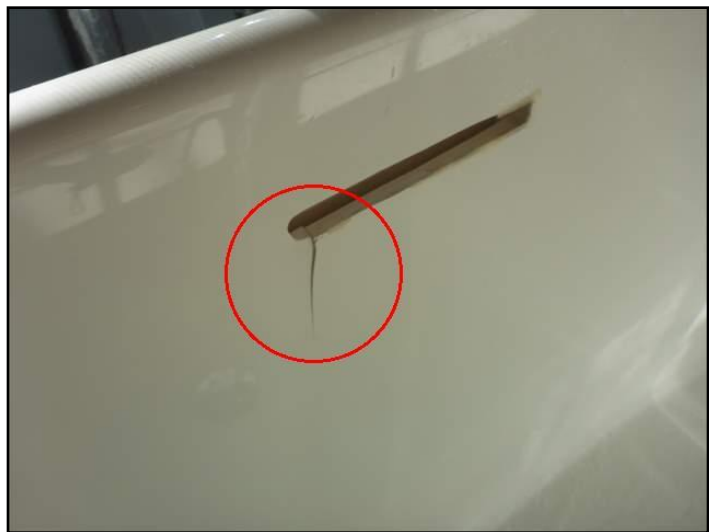
Surface defect (crack) at overflow
